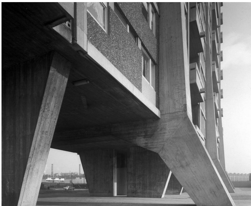
Figure 4.3: Hutchesontown C housing scheme by Basil Spence (RIBApix)
