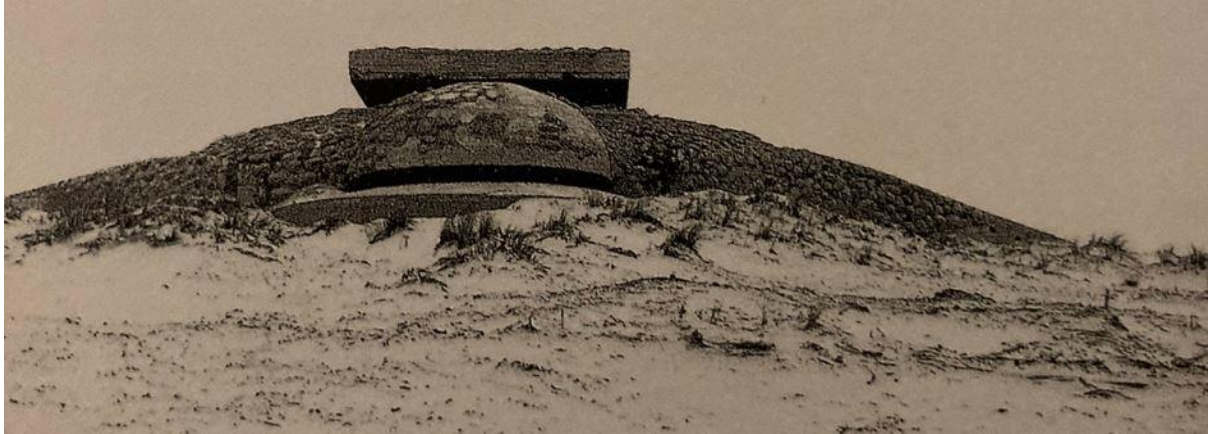
Figure 1.3: Atlantic Wall concrete camouflage 1 (Mallory and Ottar, Architecture of aggression , 1973)
