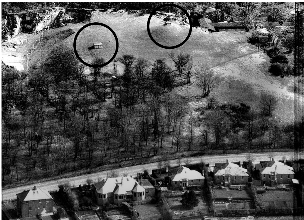
Figure 2.6: Barnton Quarry aerial photograph facing eastwards c.1953 (Barnton Quarry Restoration Group)
