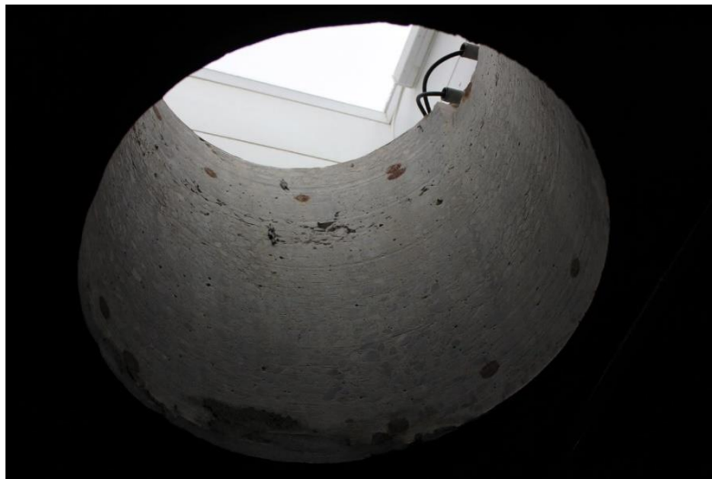
Figure 5.3: Gairloch Museum rooflight cored into concrete
