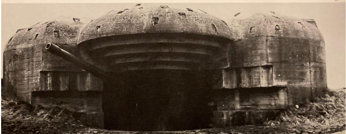
Figure 1.4: Atlantic Wall concrete camouflage 2 (Mallory and Ottar, Architecture of aggression , 1973)
