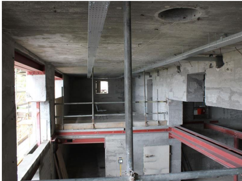
Figure 5.2: Gairloch Museum during construction
