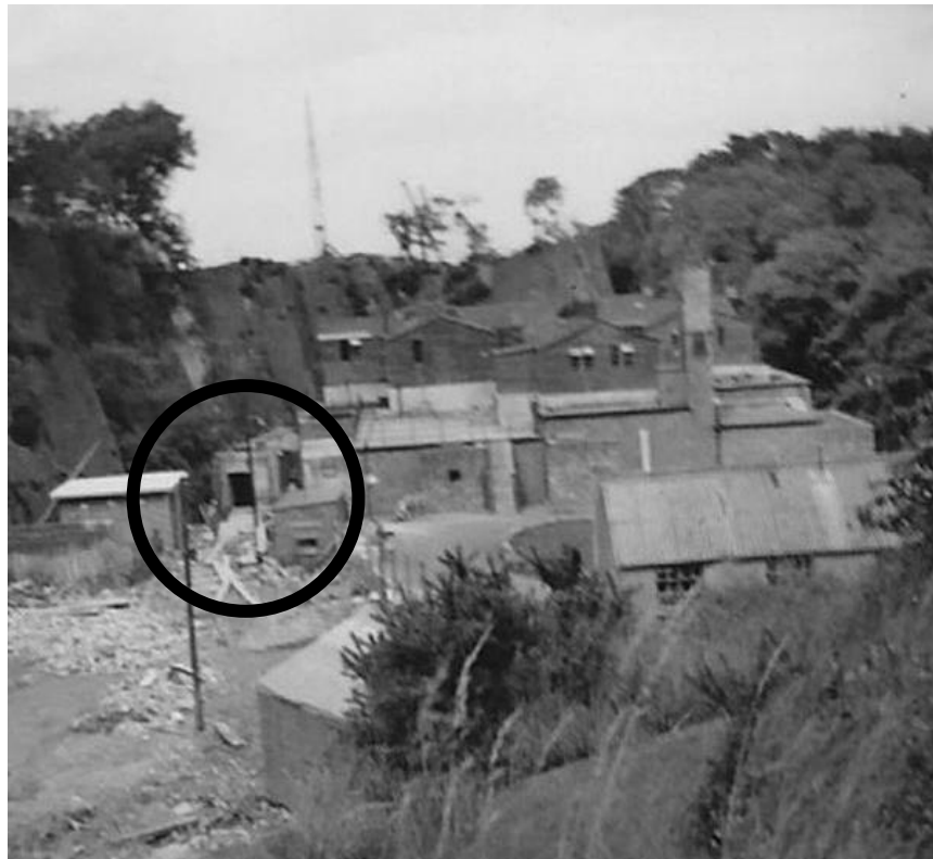
Figure 2.7: Barnton Quarry compound looking north c.1953 (Barnton Quarry Restoration Group)
