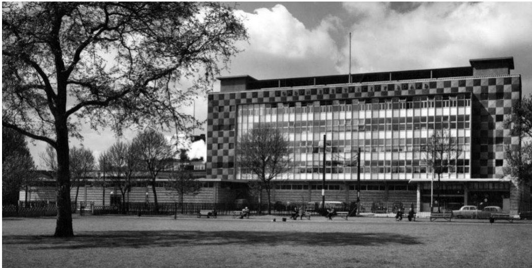
Figure 2.20: London Electricity Board HQ, London (RIBApix)
