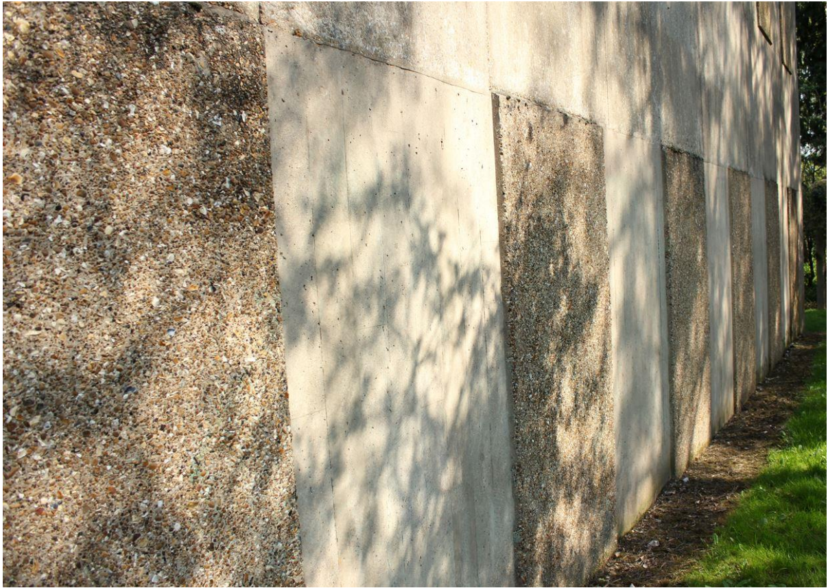
Figure 4.13: Existing concrete detail at Cambridge RSG
