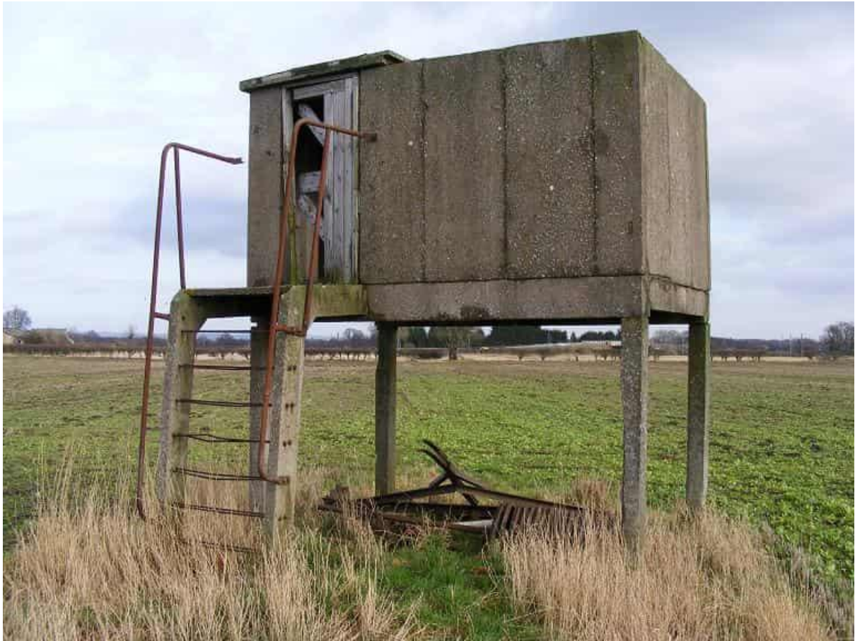
Figure 2.4: Typical above-ground 'Orlit' ROC post of the 1950s (Subbrit)
