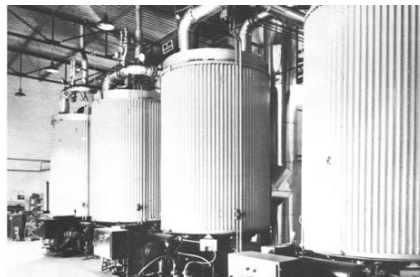
Fig.11.1 The boiler/heating systems
