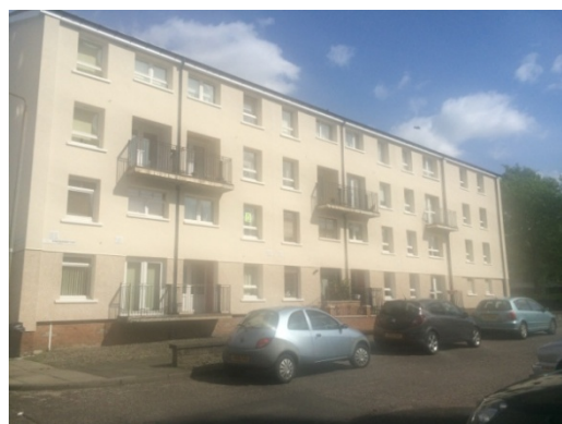
June 2015- Maisonette and walk up flats after refurbishment
