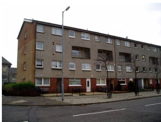
March 2008- Maisonette and walk up flats prior to refurbishment
