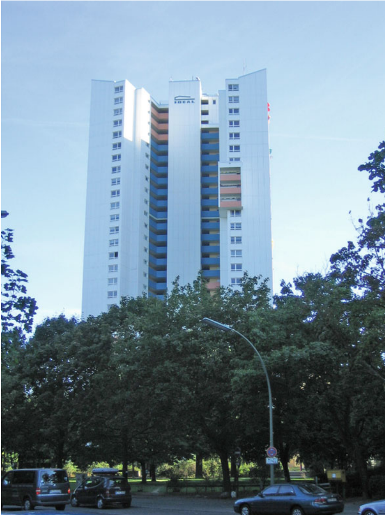
Fig. 5.5 The ‘Ideal Tower’ (1966–1969, Walter Gropius/Alexander Sviranovic), commissioned by the Ideal Construction Cooperative in the Gropiusstadt estate in West Berlin. Source Wikimedia Commons/Magnus Manske, 2008
