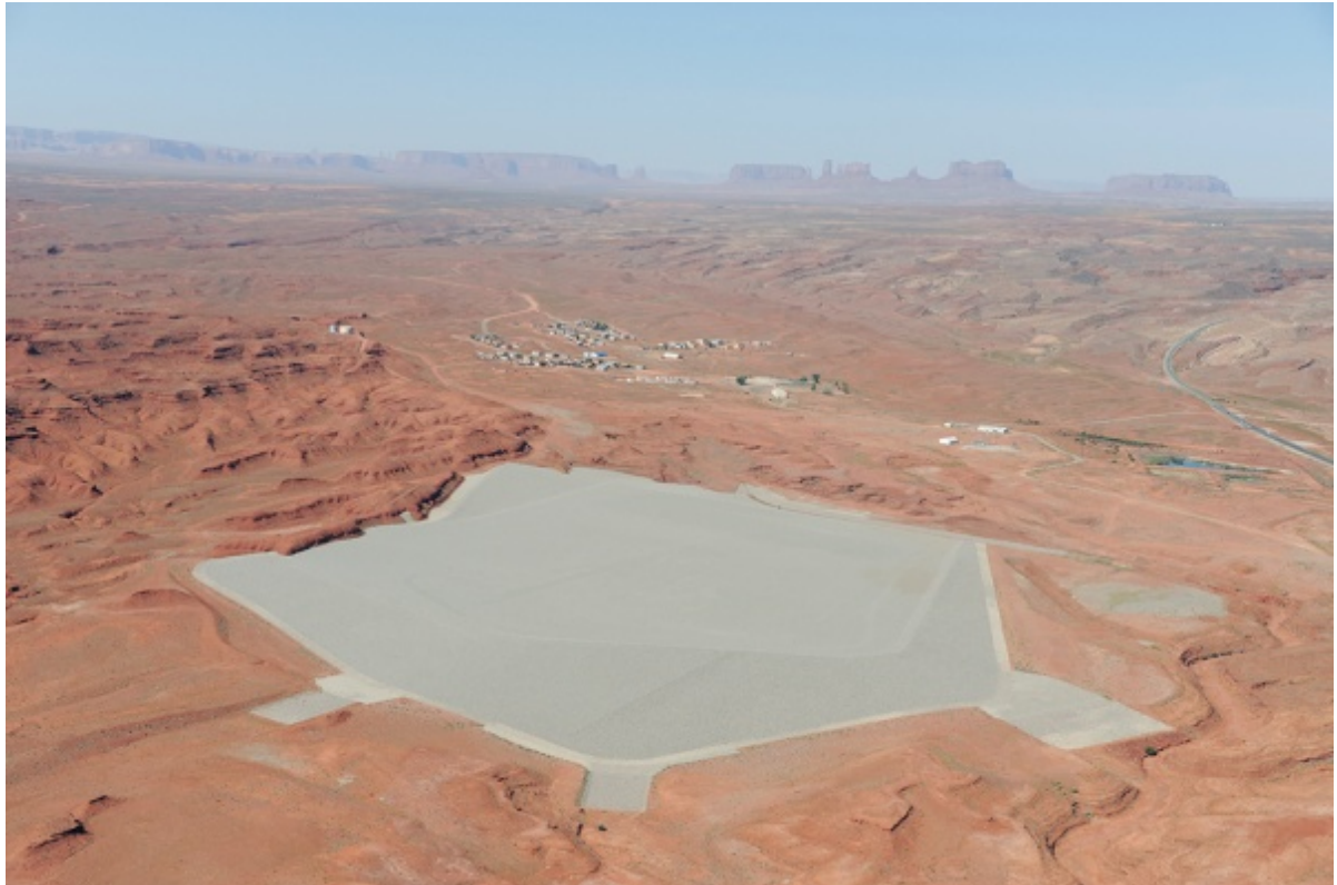
Figure 2 – CLUI Perpetual Architecture Archive (2012) Mexican Hat Disposal Cell, Utah
