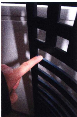
the body of the chair is ladderback type, which again is curved to the minimum, its attached to the side of the legs that runs the whole way through to the head rest.
