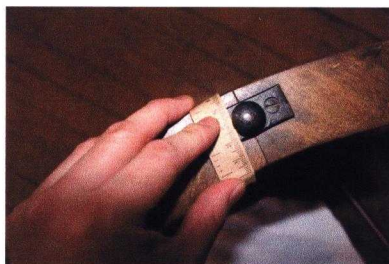
armrest bolted to the seat for more support was added later by GSA.
