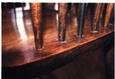
detail of how the columns are rested in the seat, the metal piece was added later on.
