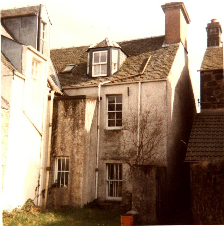
(2.8) Rear of building; close-up.
