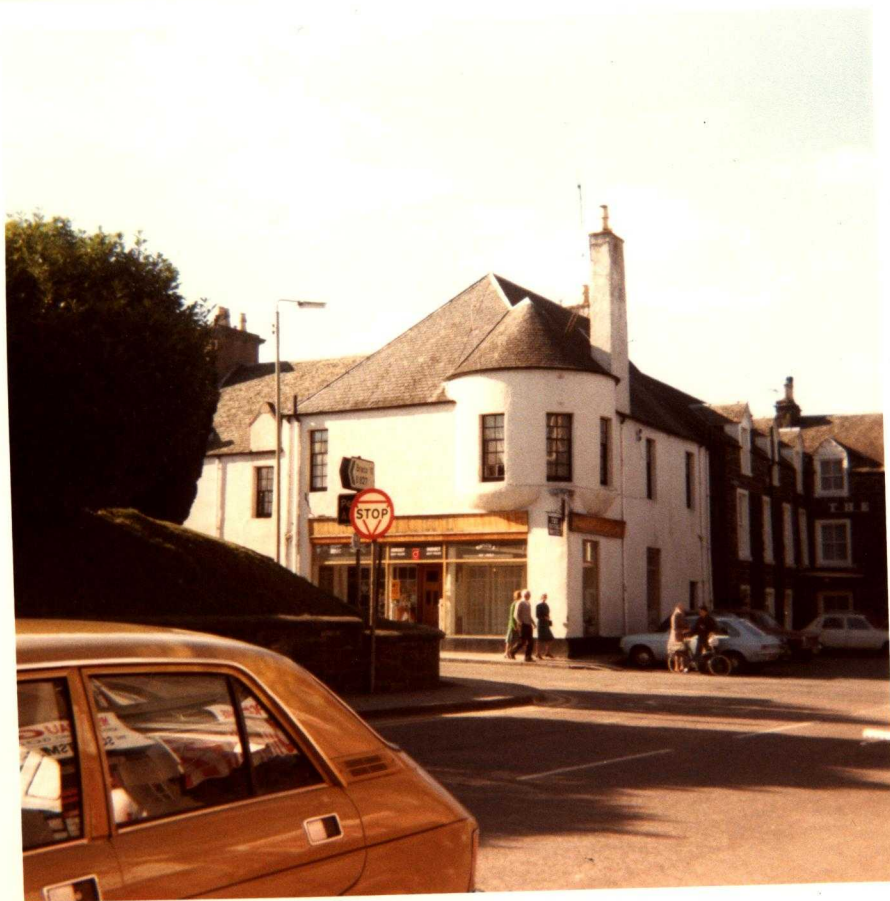
(2.2) General view of building.
