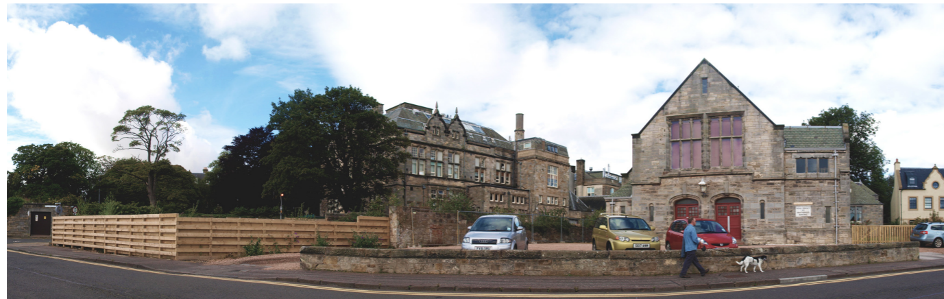
6. View from Westburn Lane looking towards junction at South Street.
