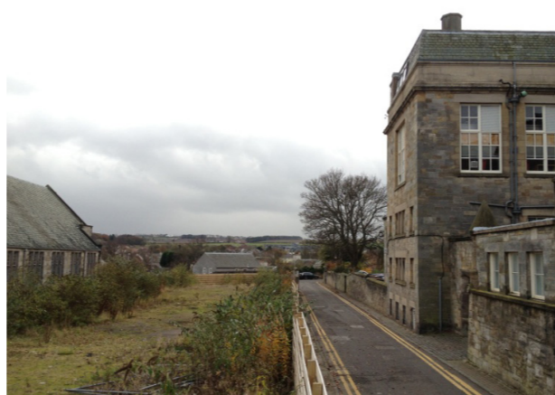
1. View looking east from West Burn Lane/ Queen's Terrace junction. The application site is bounded by timber fencing.
