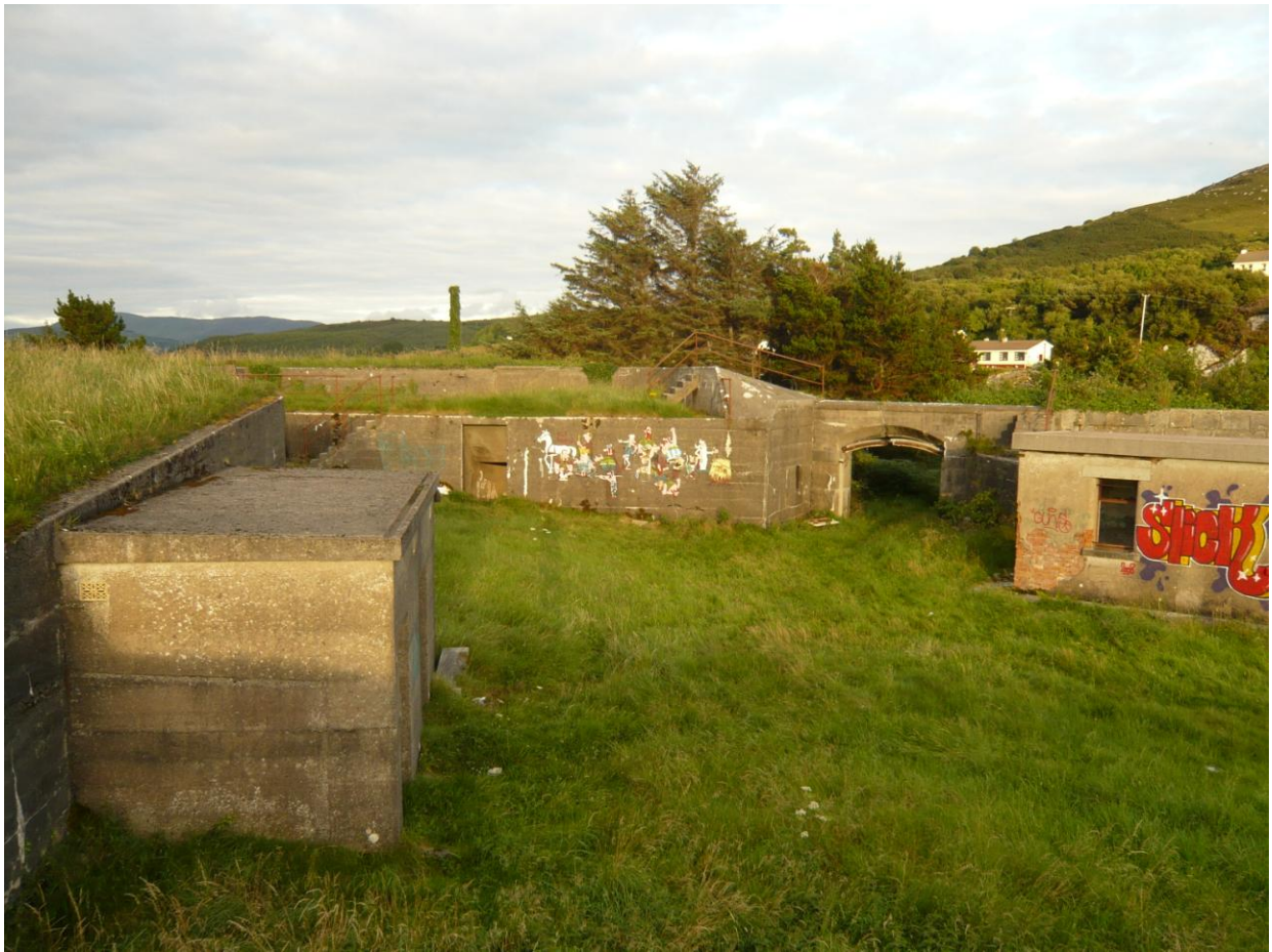
Fig. 24: Inch fort , photograph, 2011
