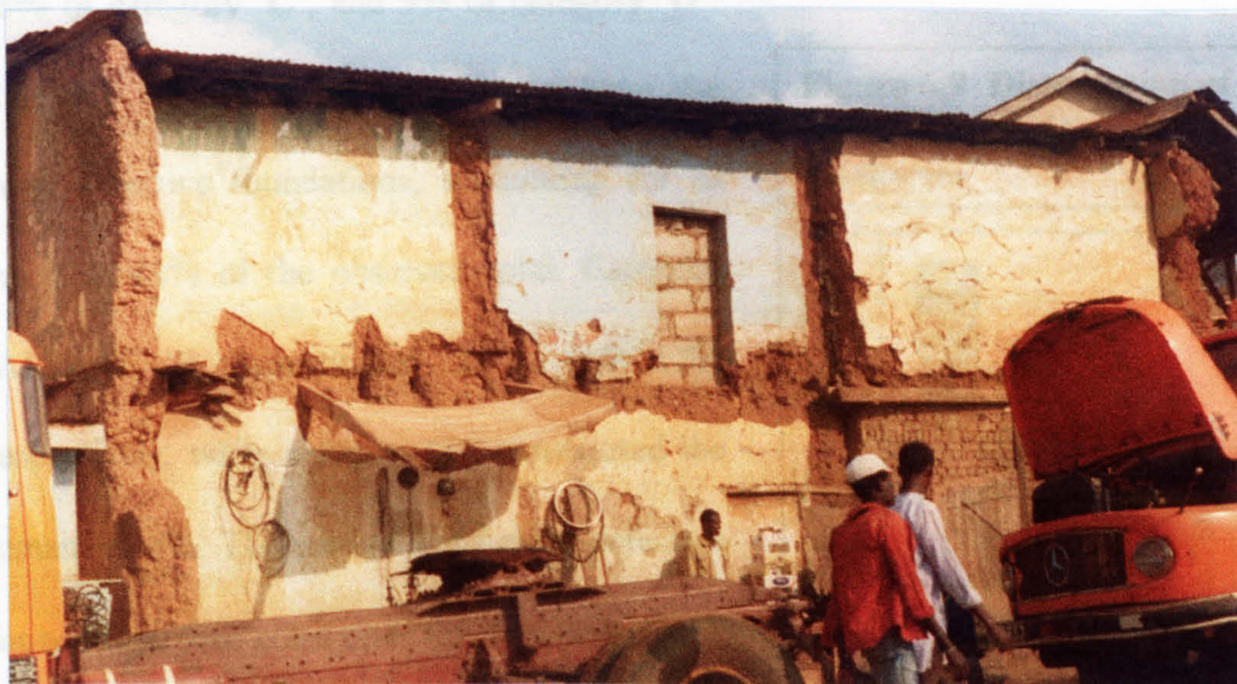
Figure 6.7 A part-fallen mud house in Sector 1
