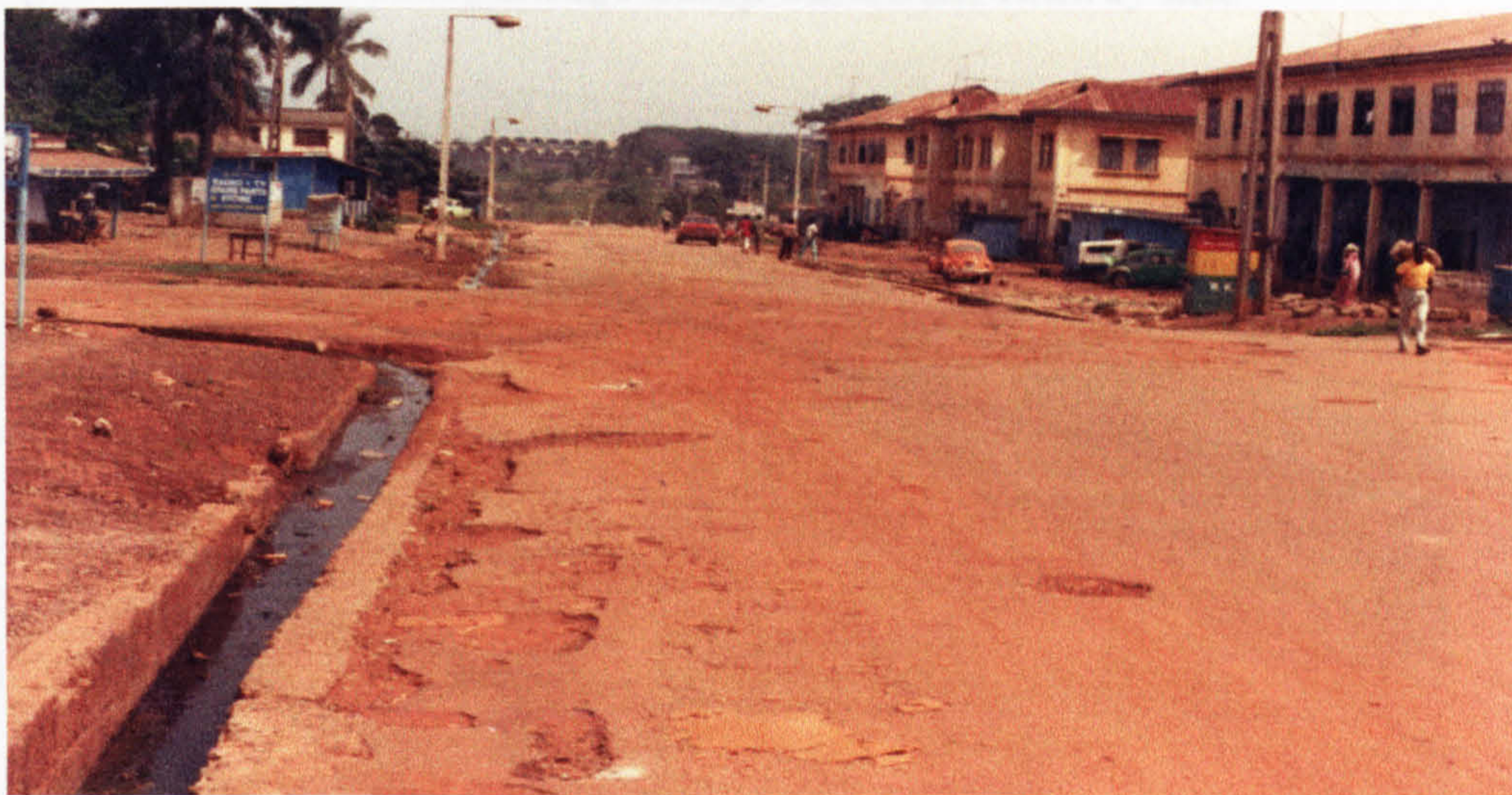
Figure 6.21 Stagnant, waste-water in a choked gutter
