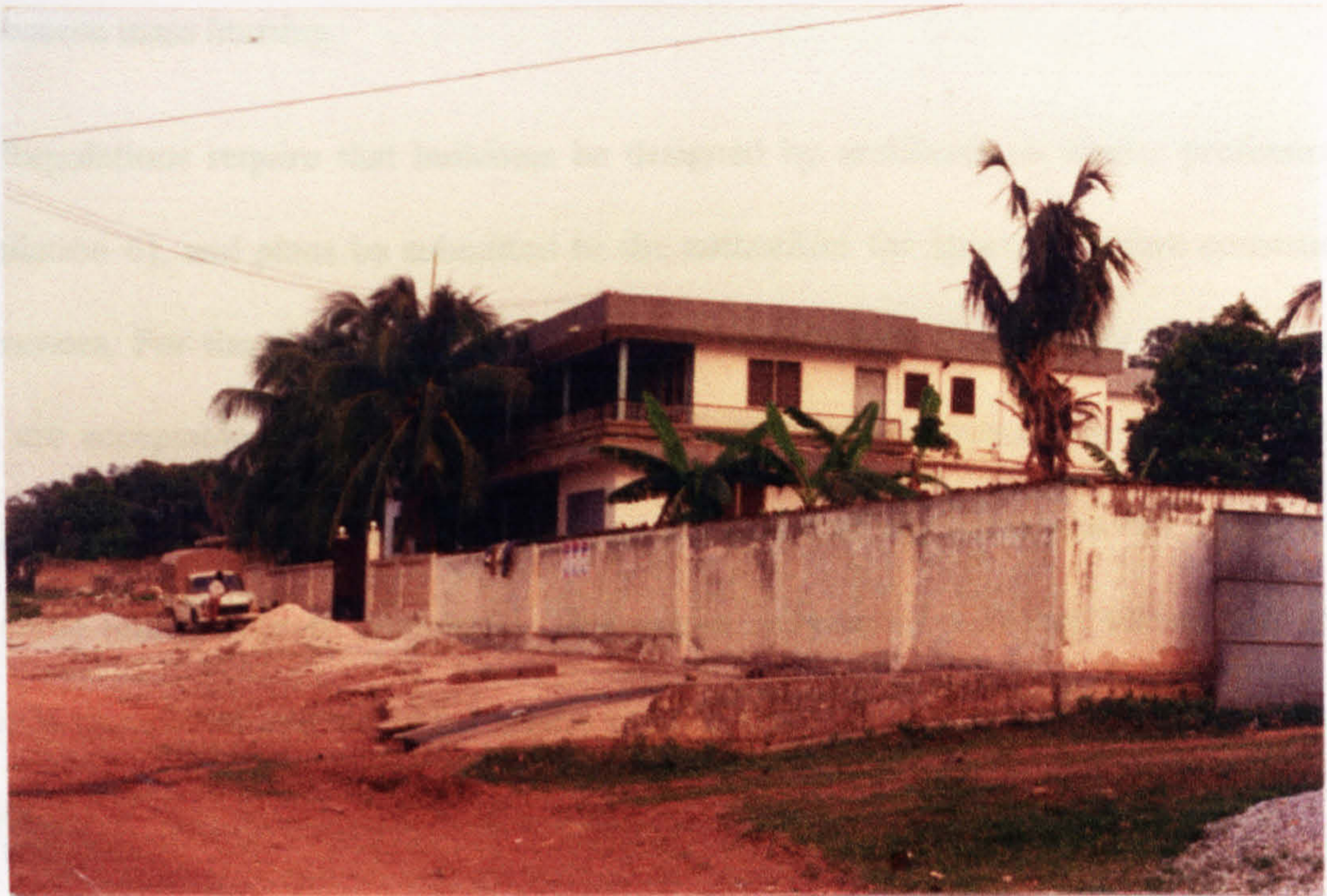
Figure 2.14 House with a two-metre high fence wall
