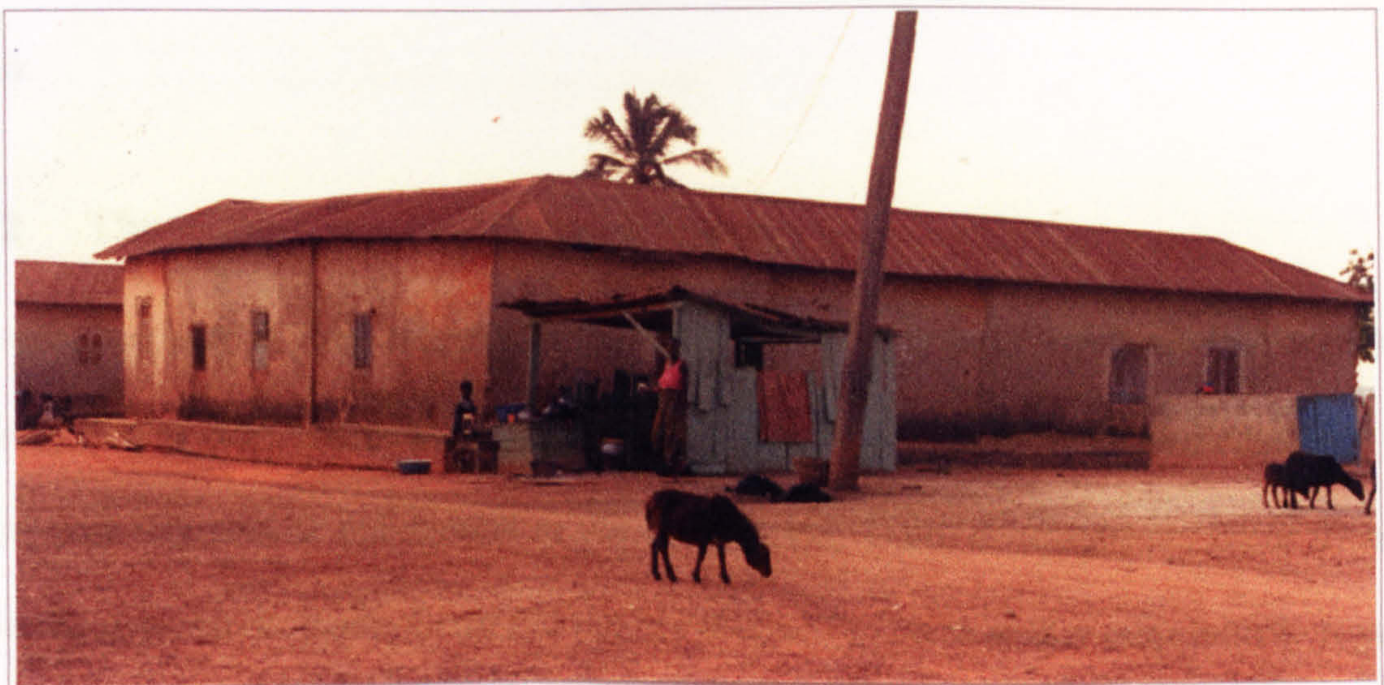
Figure 2.5 A single-storey traditional compound house (private, informal)
