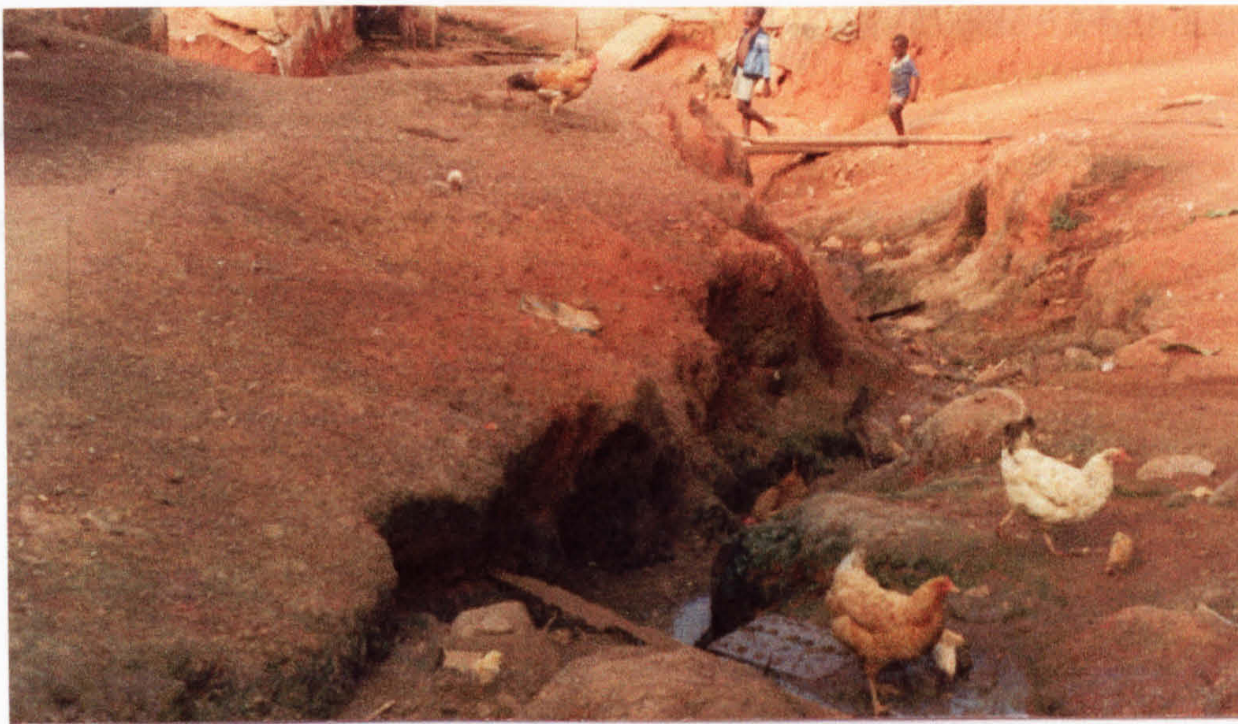
Figure 6.23 The effects of erosion on a street
