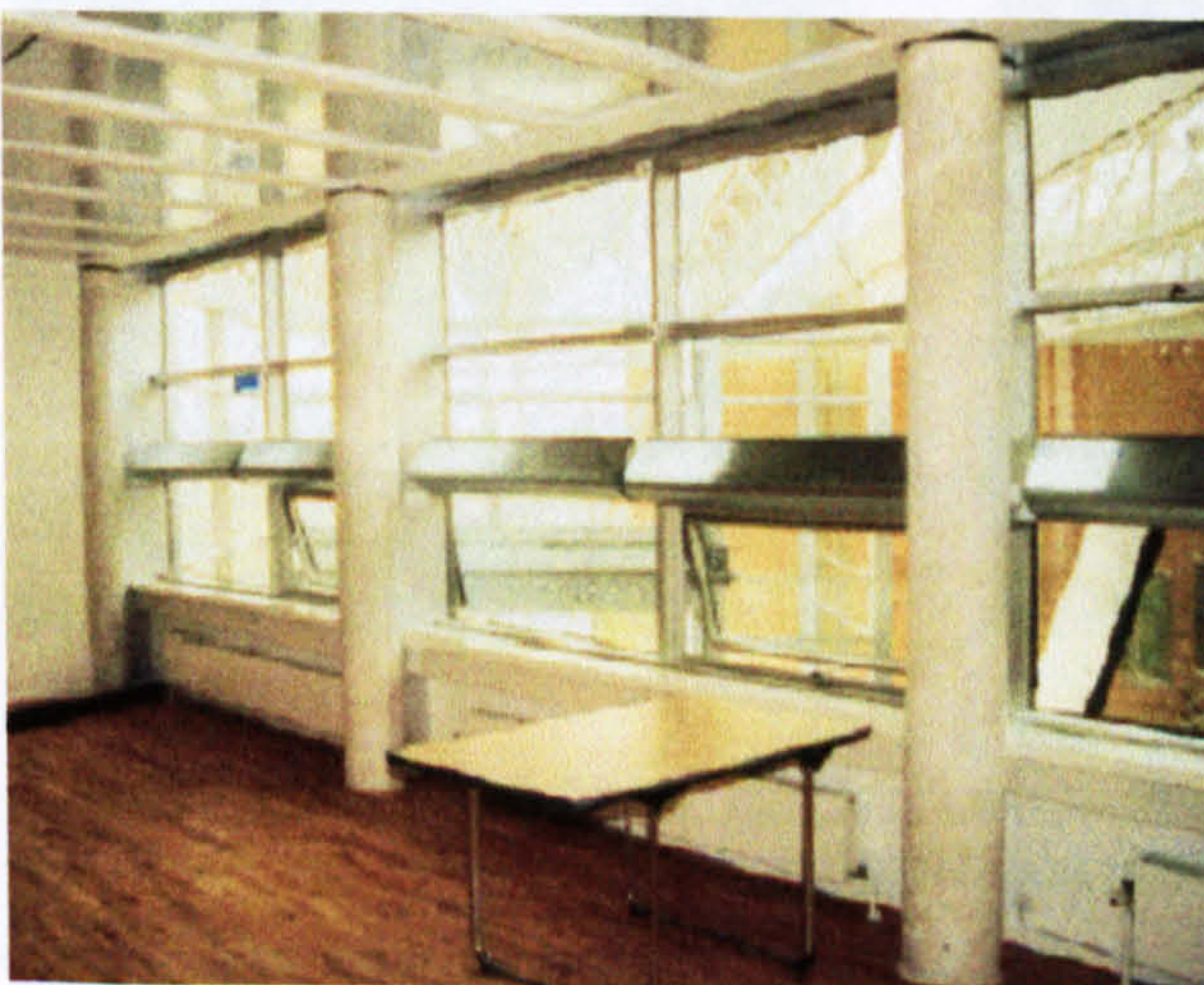
Fig. 2.24 Brundtland Centre, Tofthund, Denmark. Daylight control in offices
