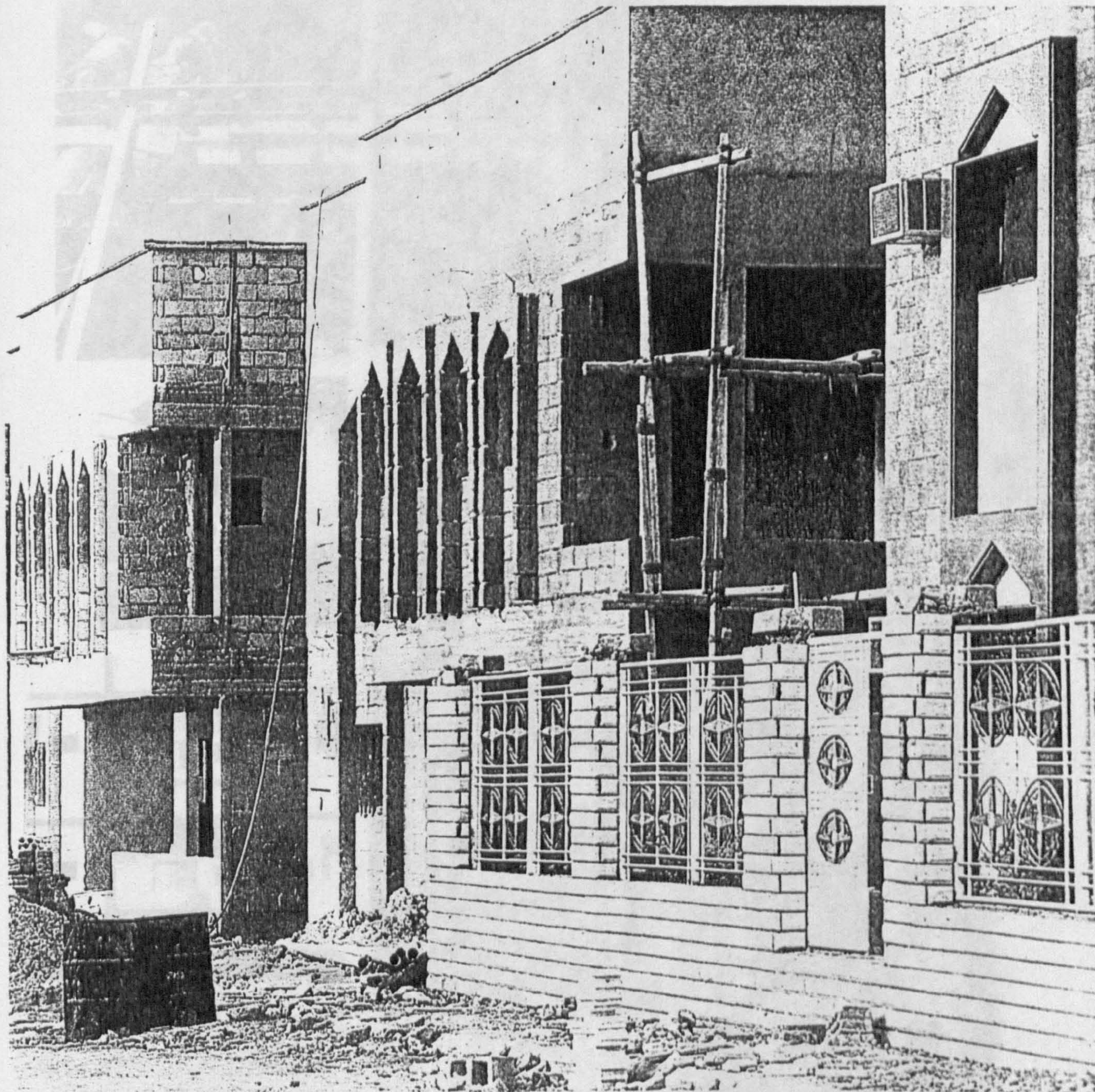
Fig 15-28 VIEW OF CONTEMPORARY BUILDING MATERIALS (3) (The use of cement brick and concrete).
