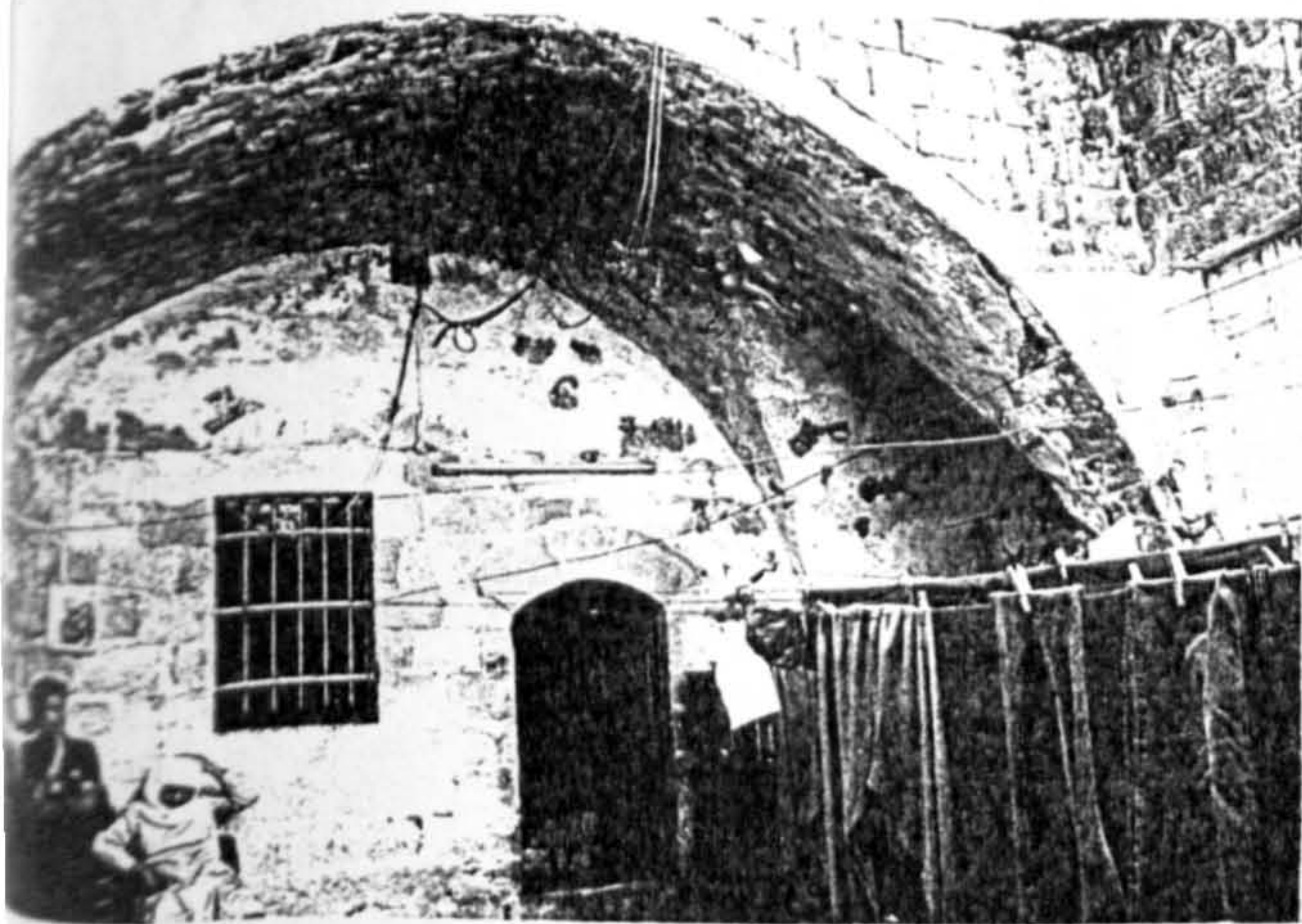
Plate (1.8): The covered part of the interior court of flat (1.G1).
