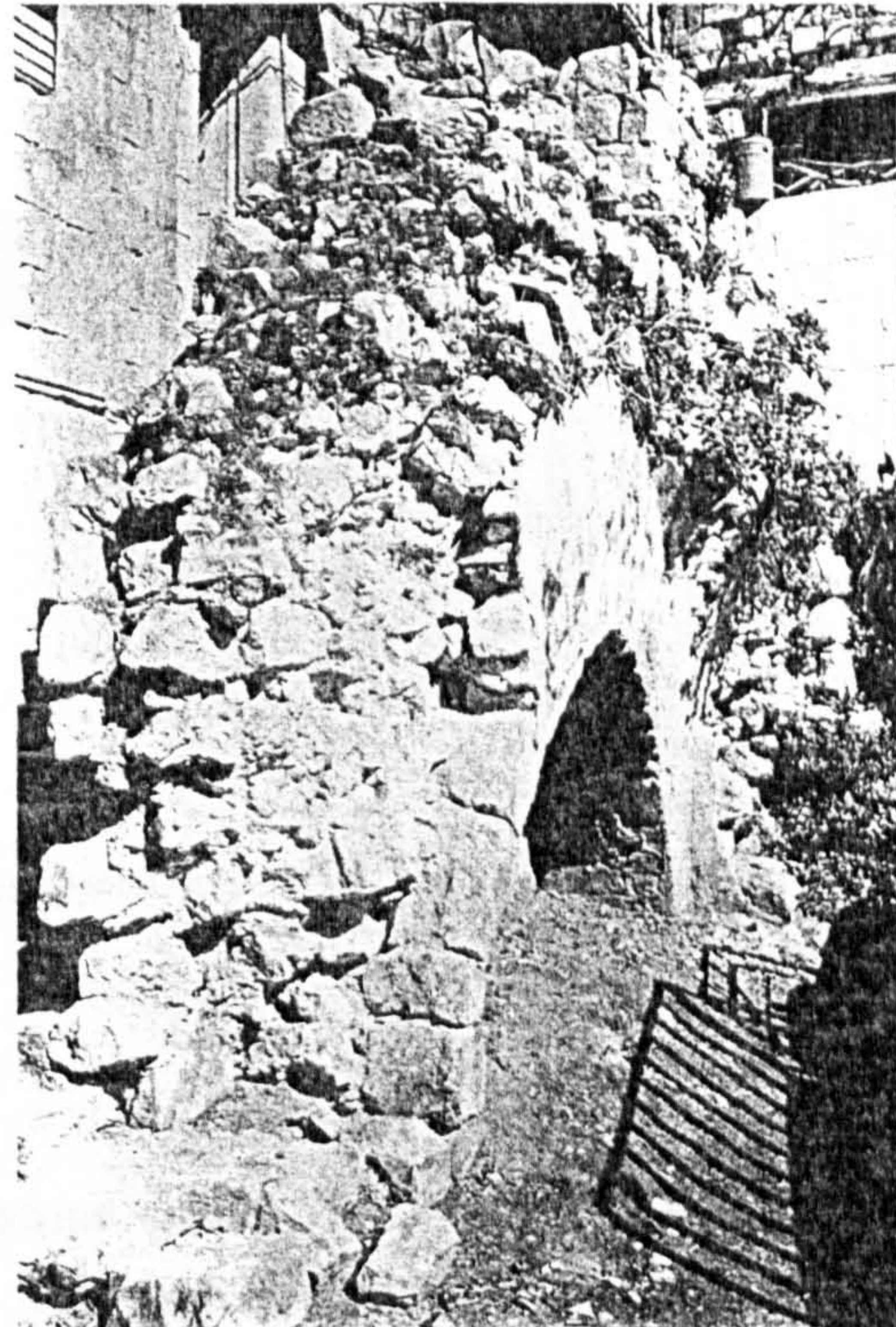
Figure (4.52): A cross-section of a collapsed traditional wall.
