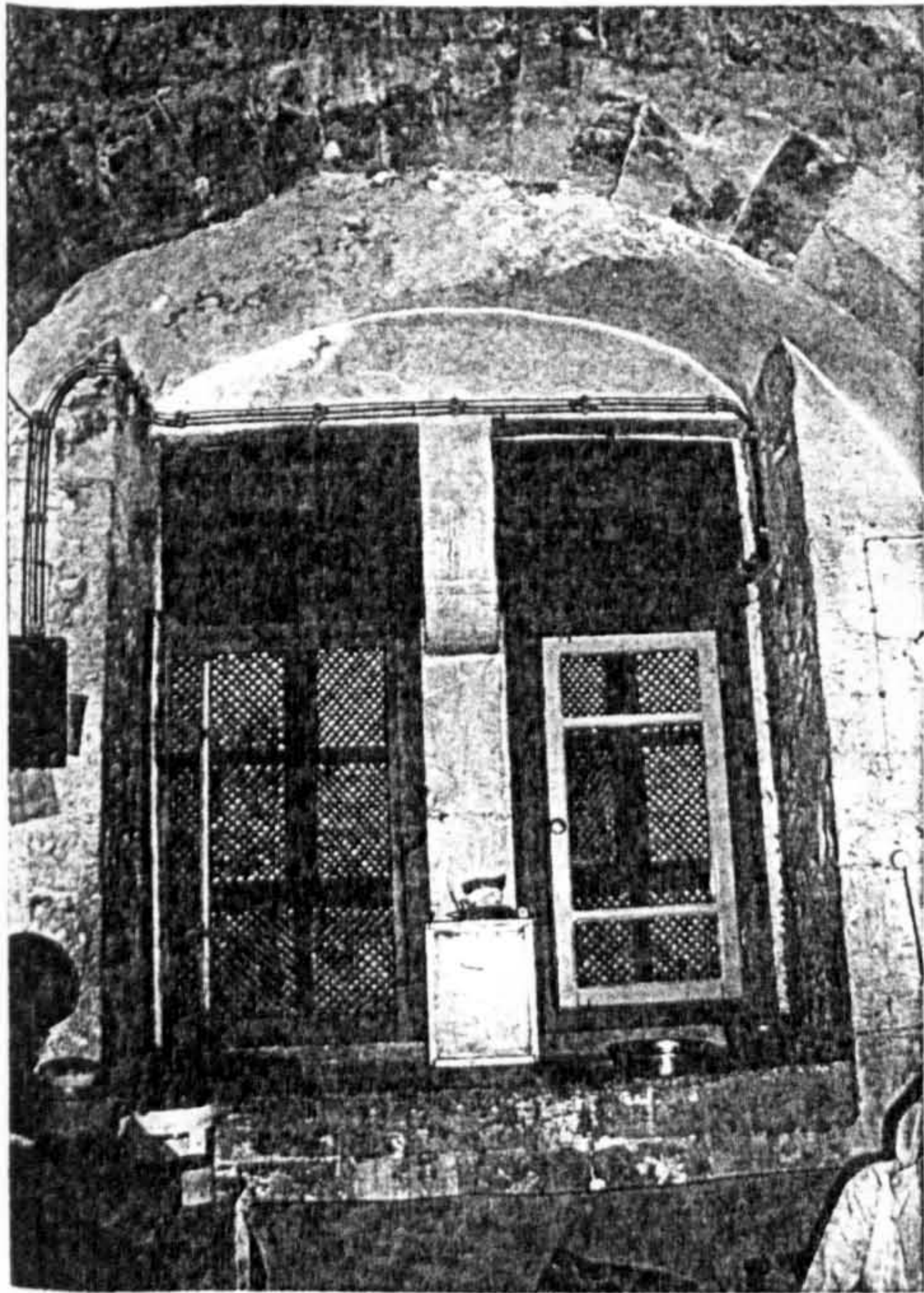
Plate (4.20): Traditional windows within flat (4.F5); notice the closure of their tops with wooden sheets.
