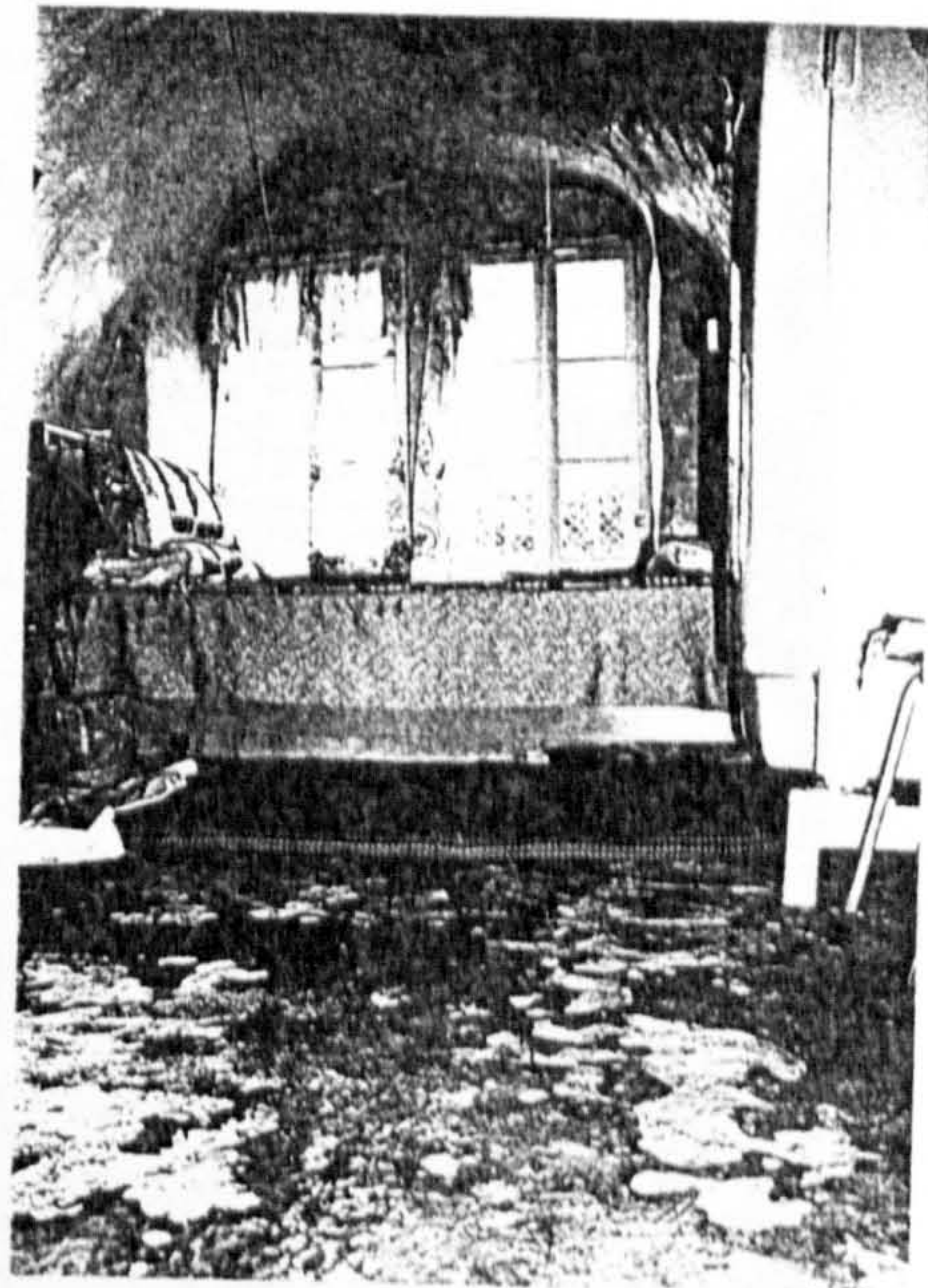
Plate (5.21): First floor main room of the same flat (5.GF2).
