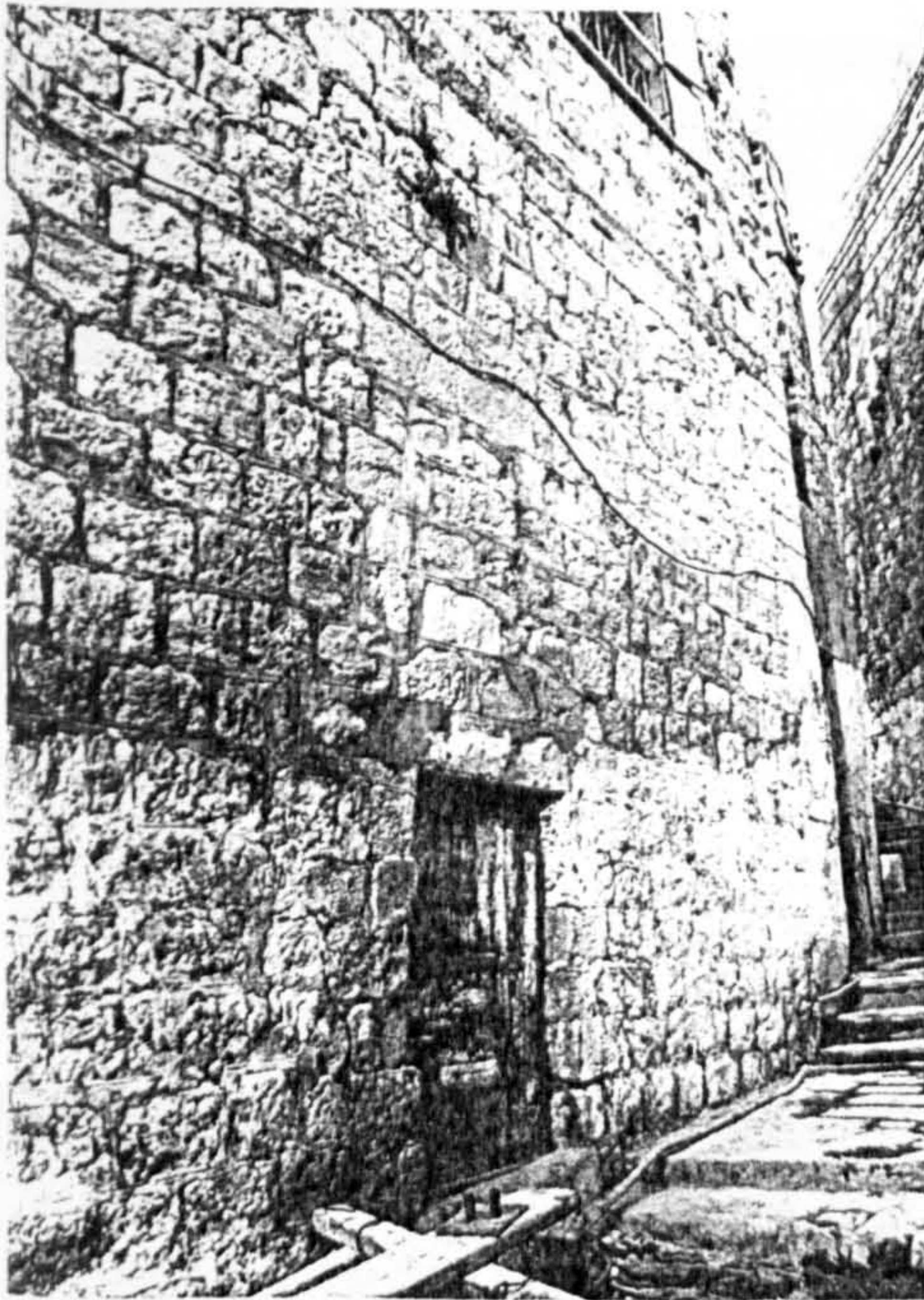
Plate (6.5): The west elevation of the southern part of building no.6; which has a store place on the basement.
