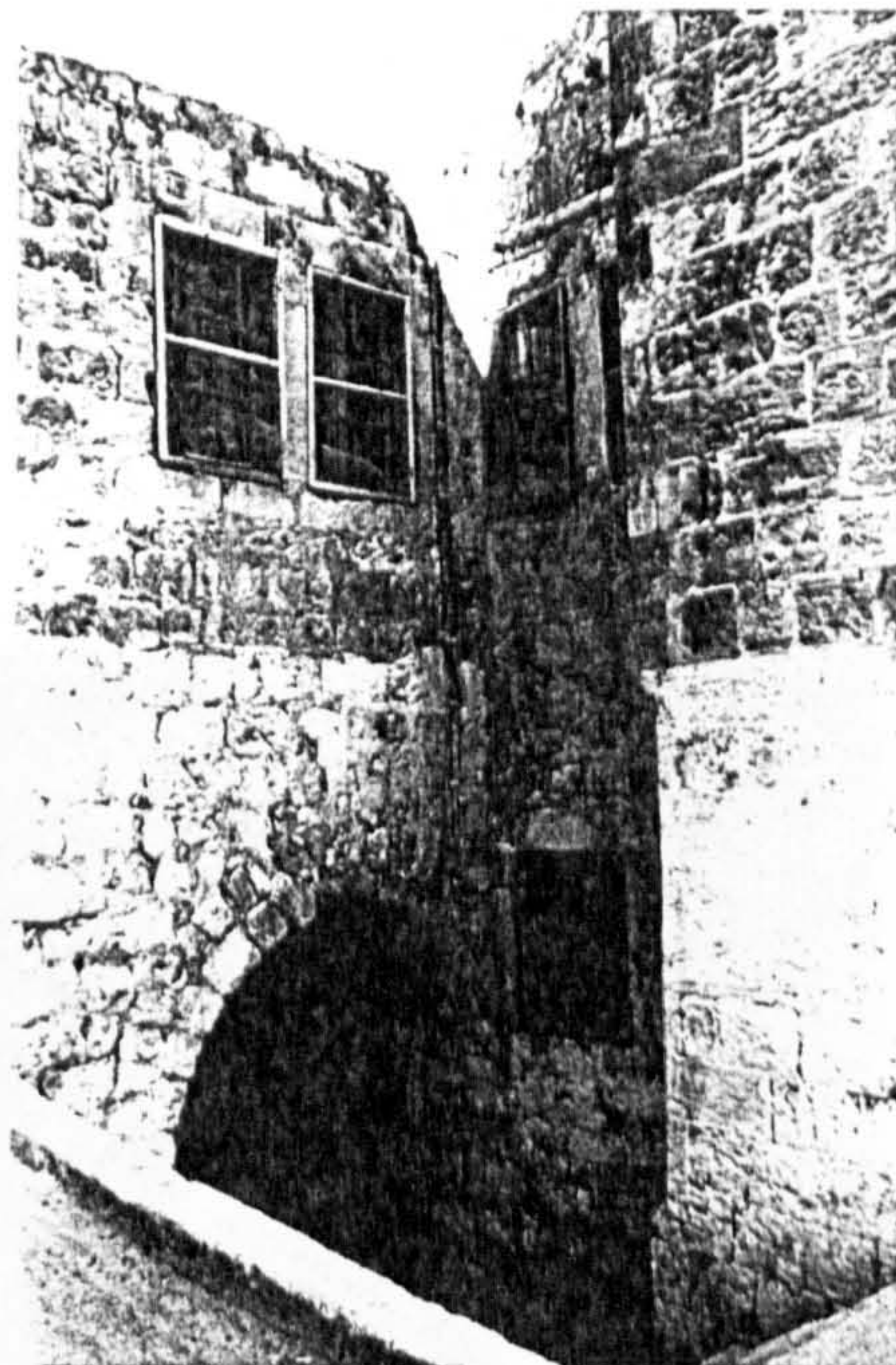
Plate (5.7): South-east elevation which has the main entrances of flats (5.GF2) and (5.GF3).
