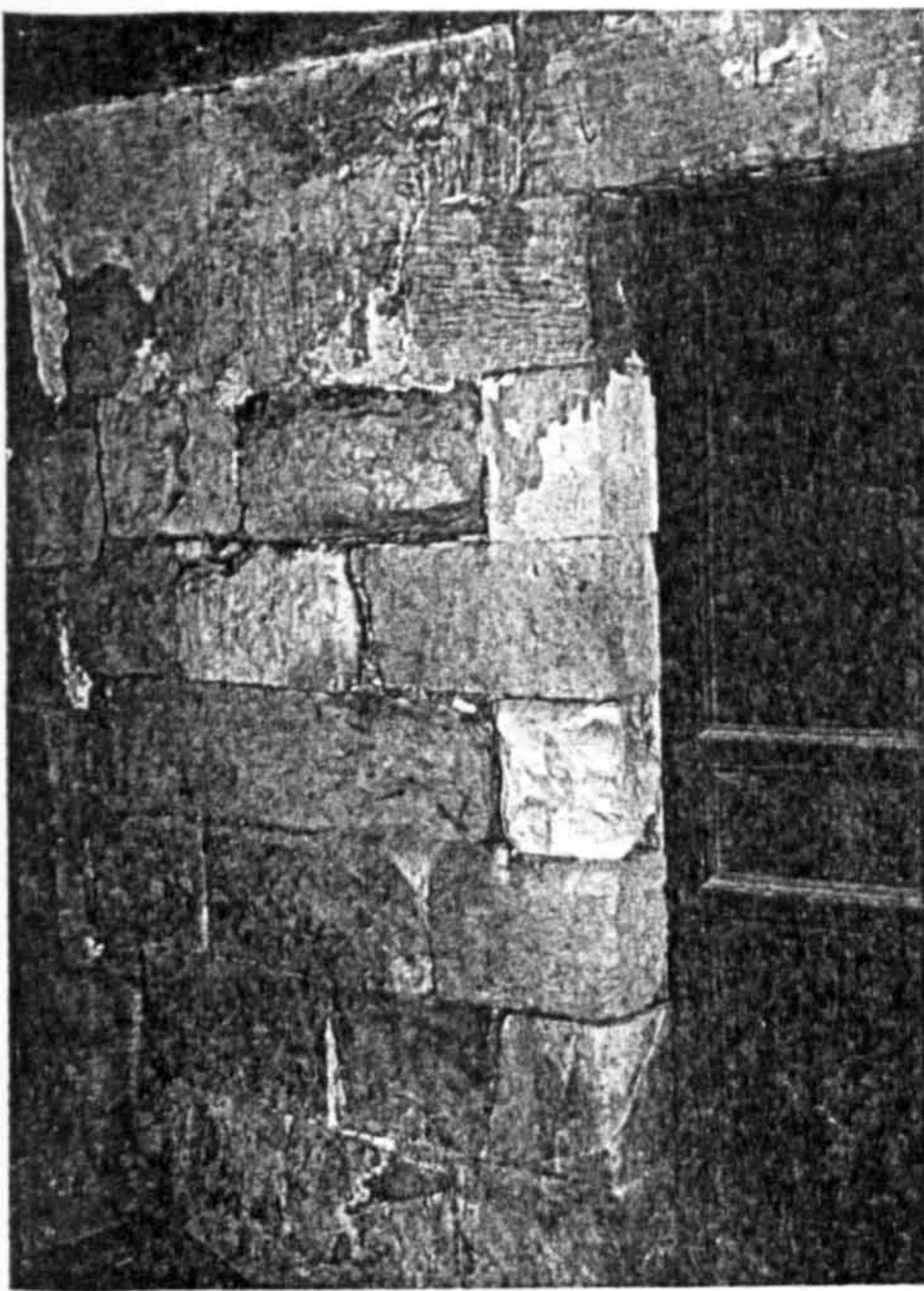
Plate (2.9): The condition of interior stone within the ground floor.
