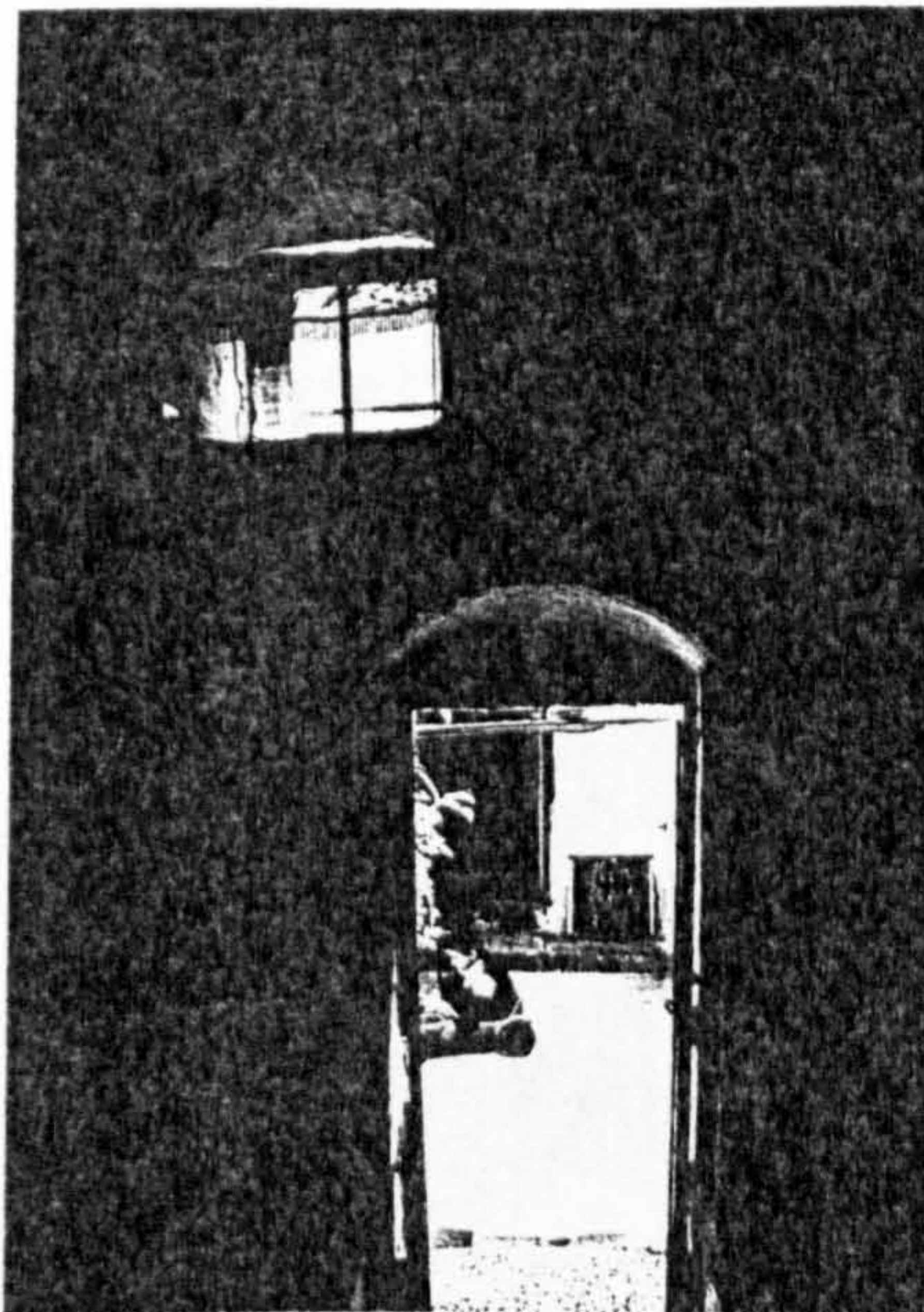
Plate (5.14): Looking towards the court of flat (5.GF3) from this bed room; notice the only upper window it has.
