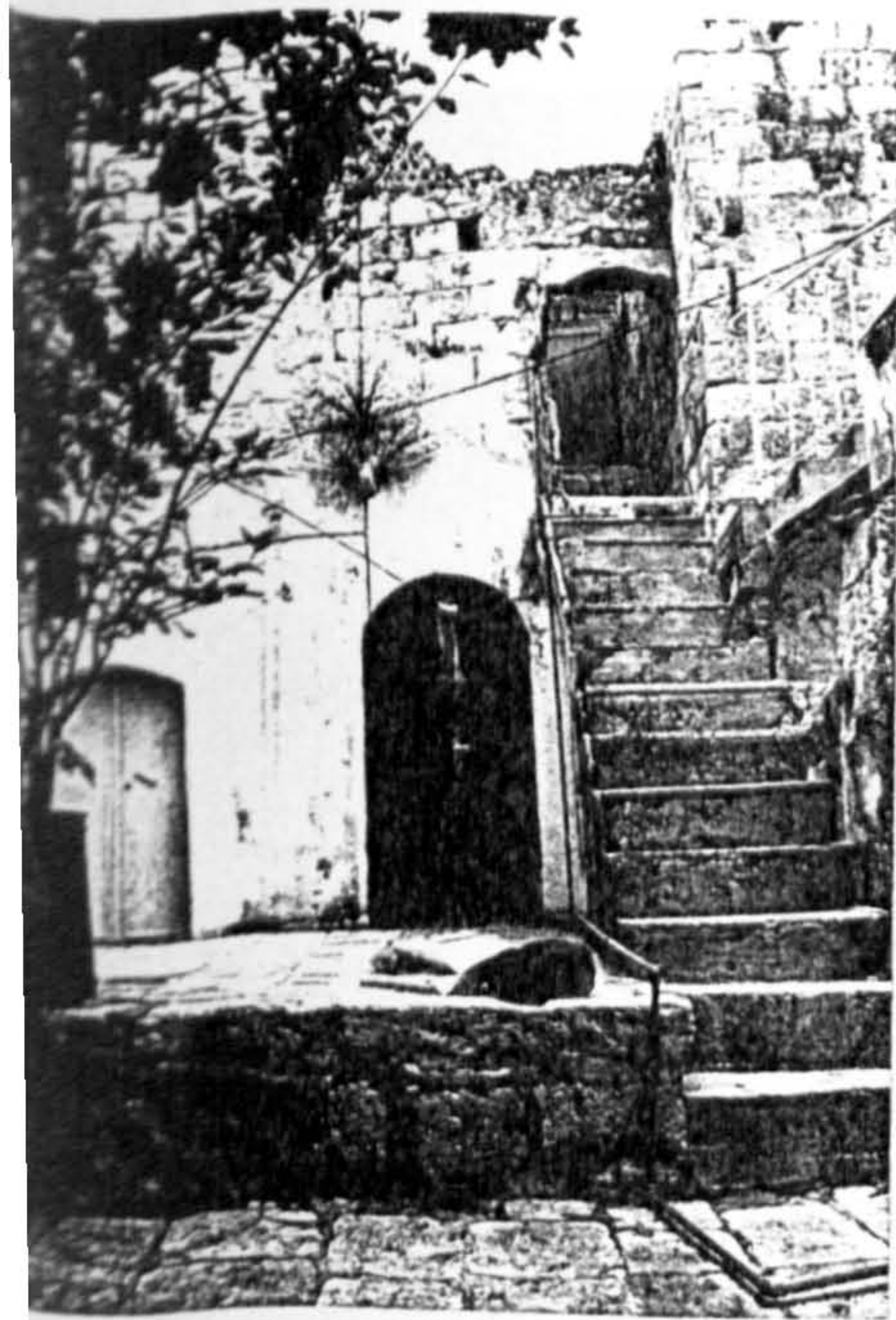
Plate (1.10): First floor terrace looking north. Figure (8.15): Building no. 1, Existing Condition.
