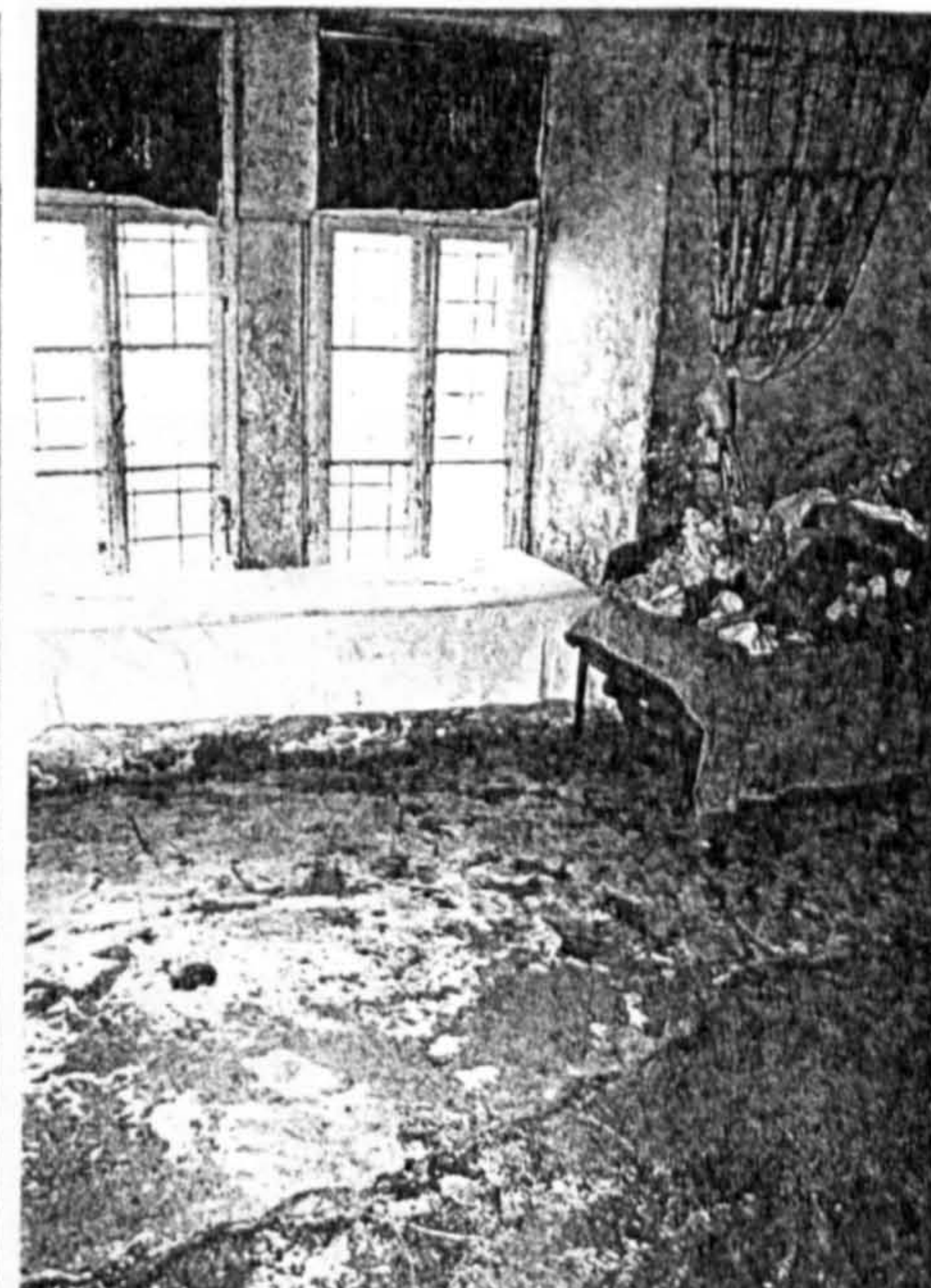
Plate (4.7): A traditional floor within flat 4.G2 in bad condition.
