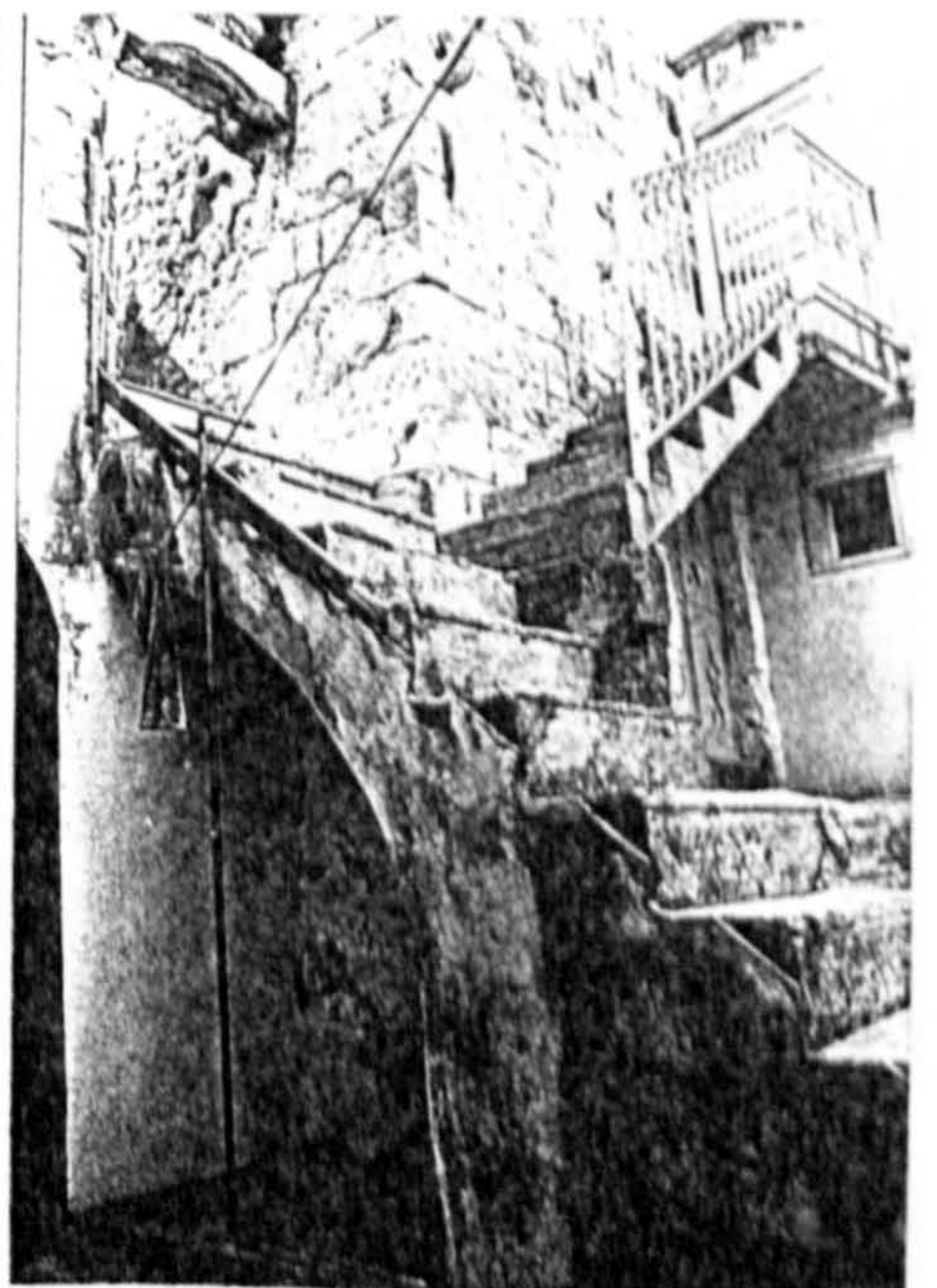
Plate (1.12): Stairs leading to the second floor flats; notice their unsafe design.
