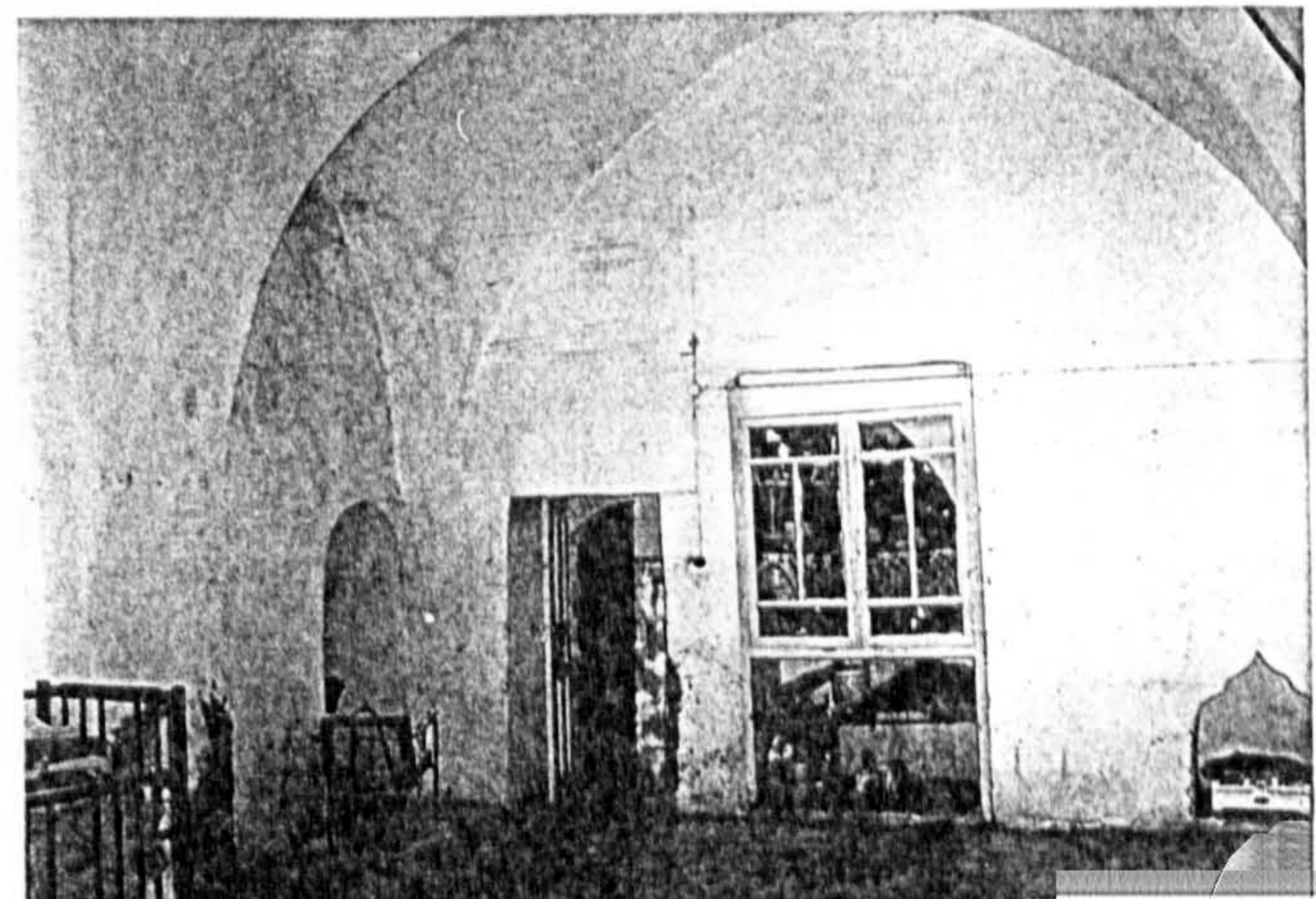
Plate (4.24): Interior view of a bed-setting room within flat (4.F.5); notice how large it its size is.
