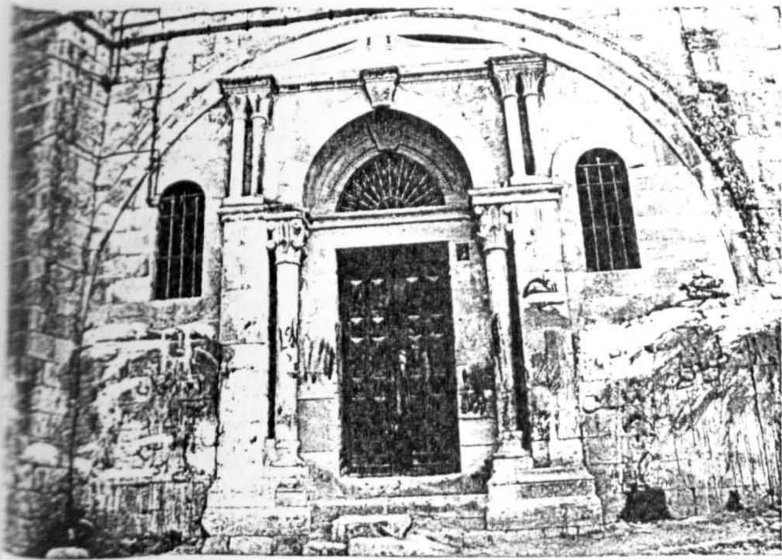
Plate (2.1): Main entrance of building no.2; notice stone bad condition.
