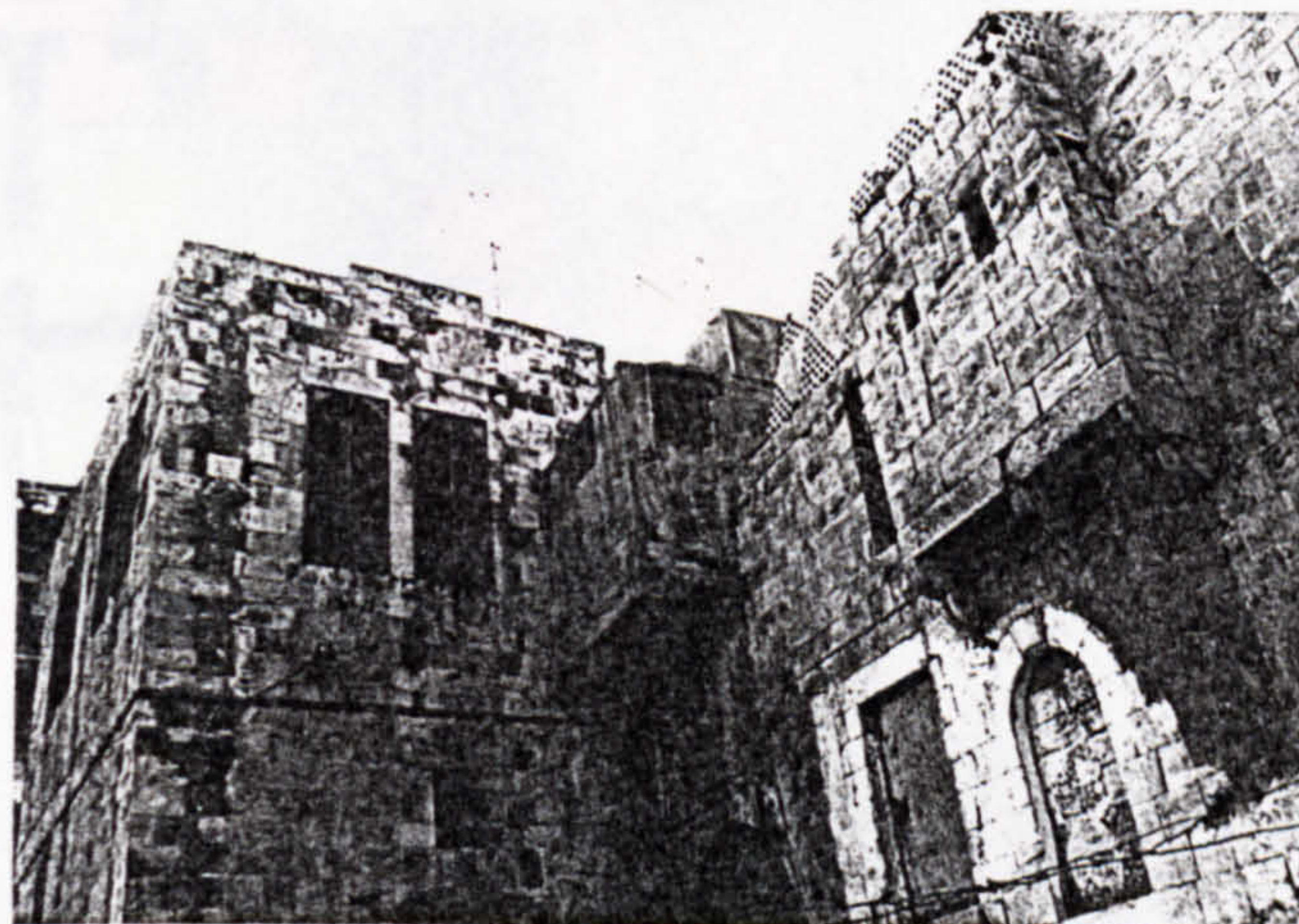
Plate (4.C): The two cantilever structures on the east elevation.
