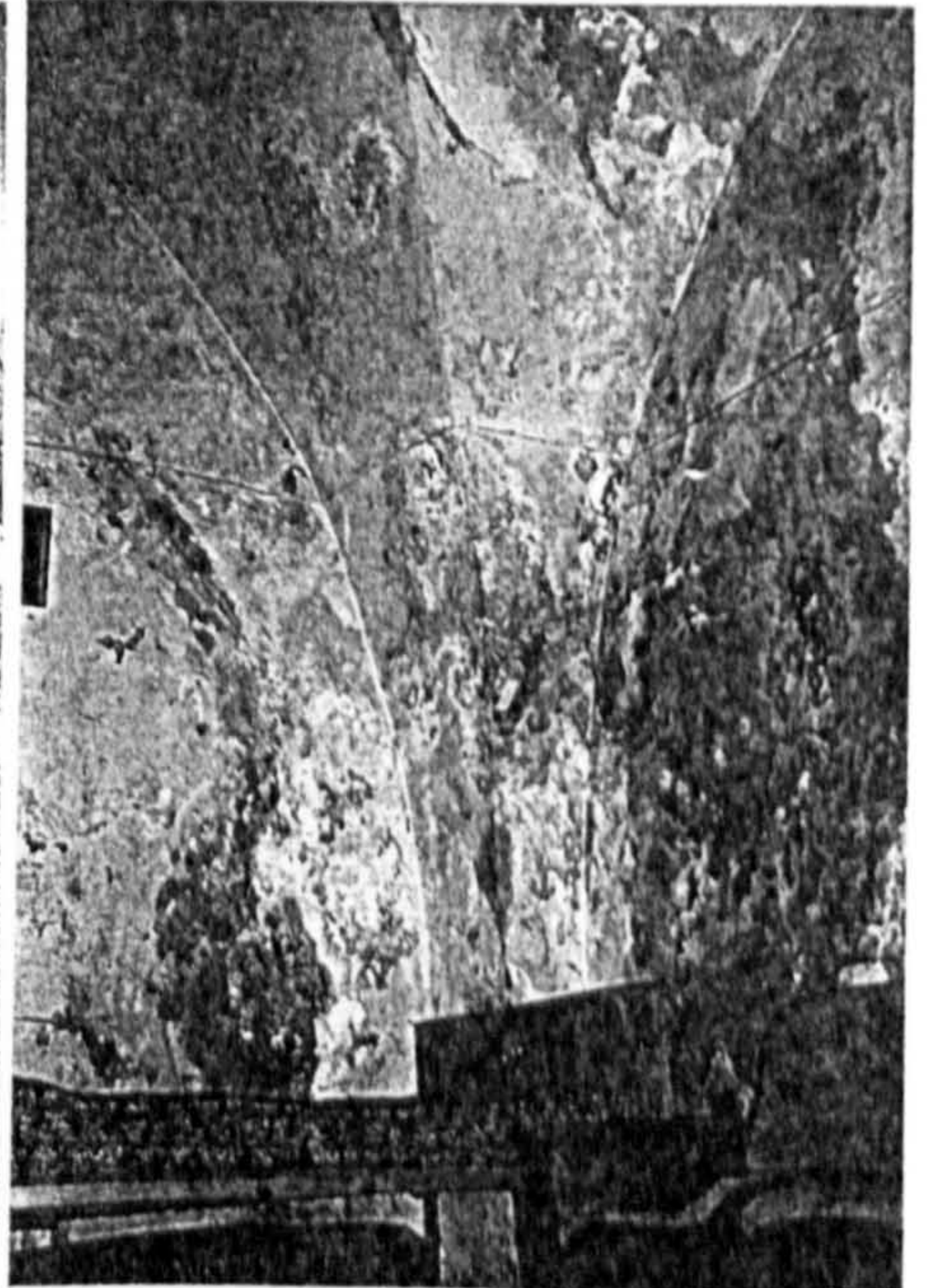
Plate (10.8): One corner inside a bed-setting room within flat (10.F2); notice the dampness effects on the walls and vault structures.
