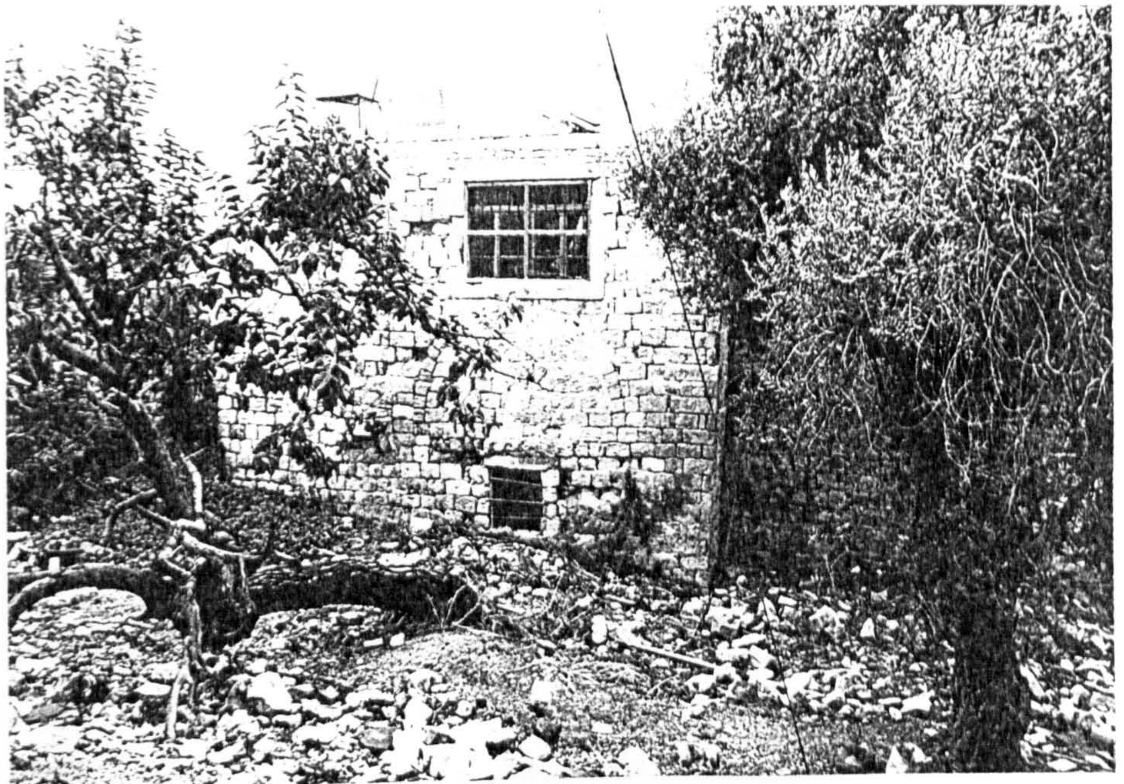
Plate (8.1): South elevation; notice the ignored garden.
