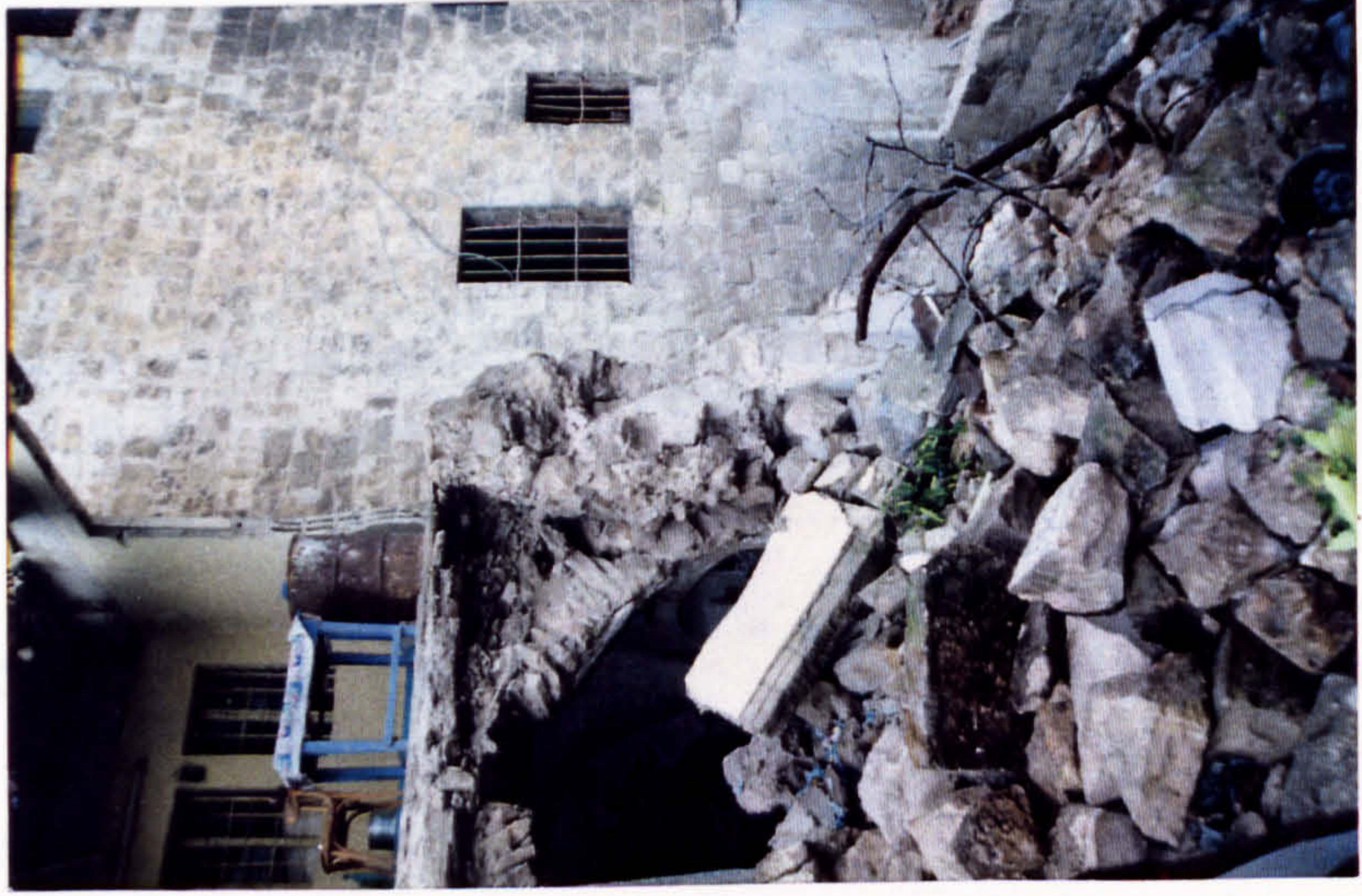
E & F. The effect of using explosives on neighbouring buildings to demolish one housing unit among the highly concentrated built environments of the Old Town. Source: Courtesy of Mr Tibawi, 1989.
