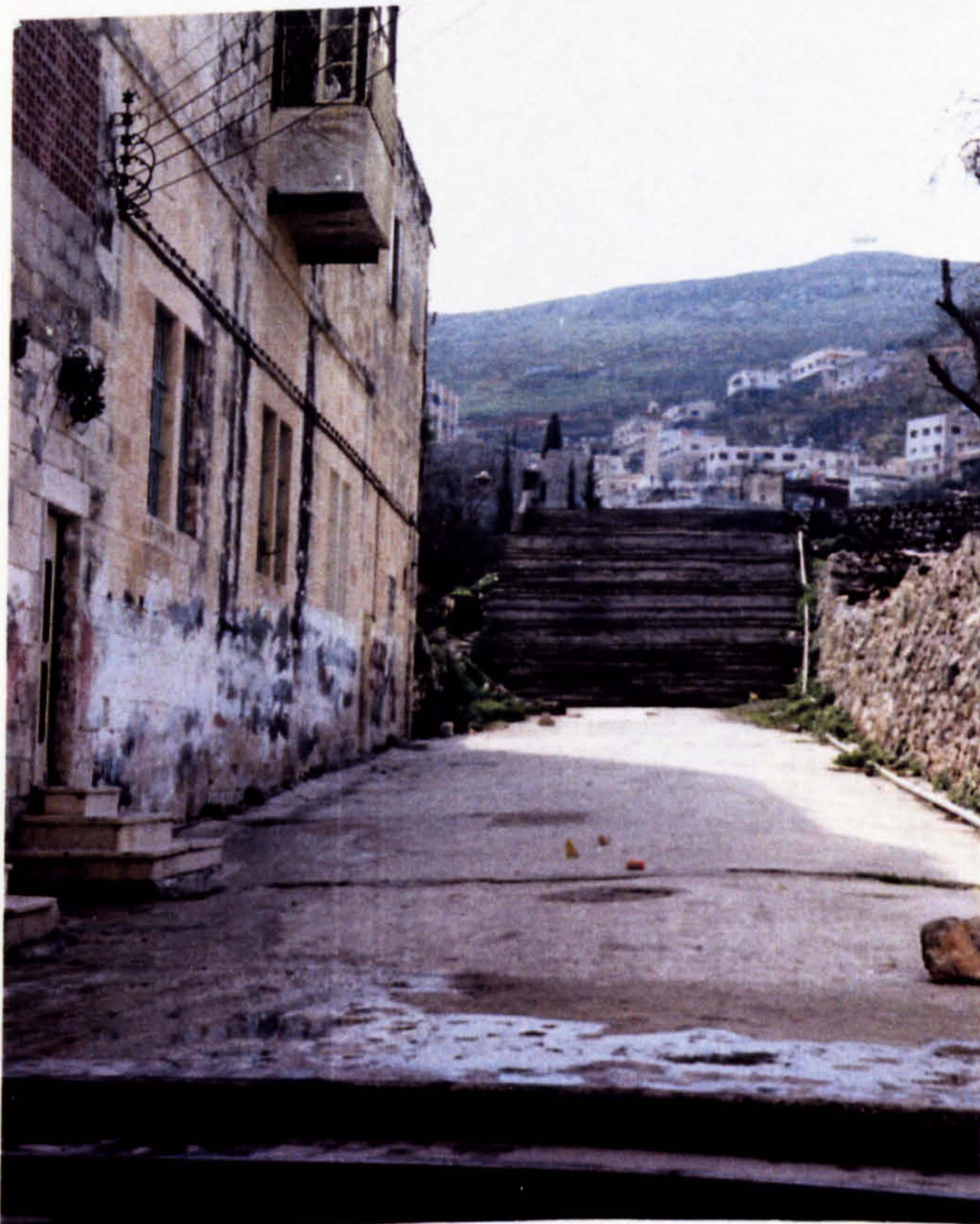
D. Concrete surfaces and steps. Source: Courtesy of Mr. F. Yaish,1991.
