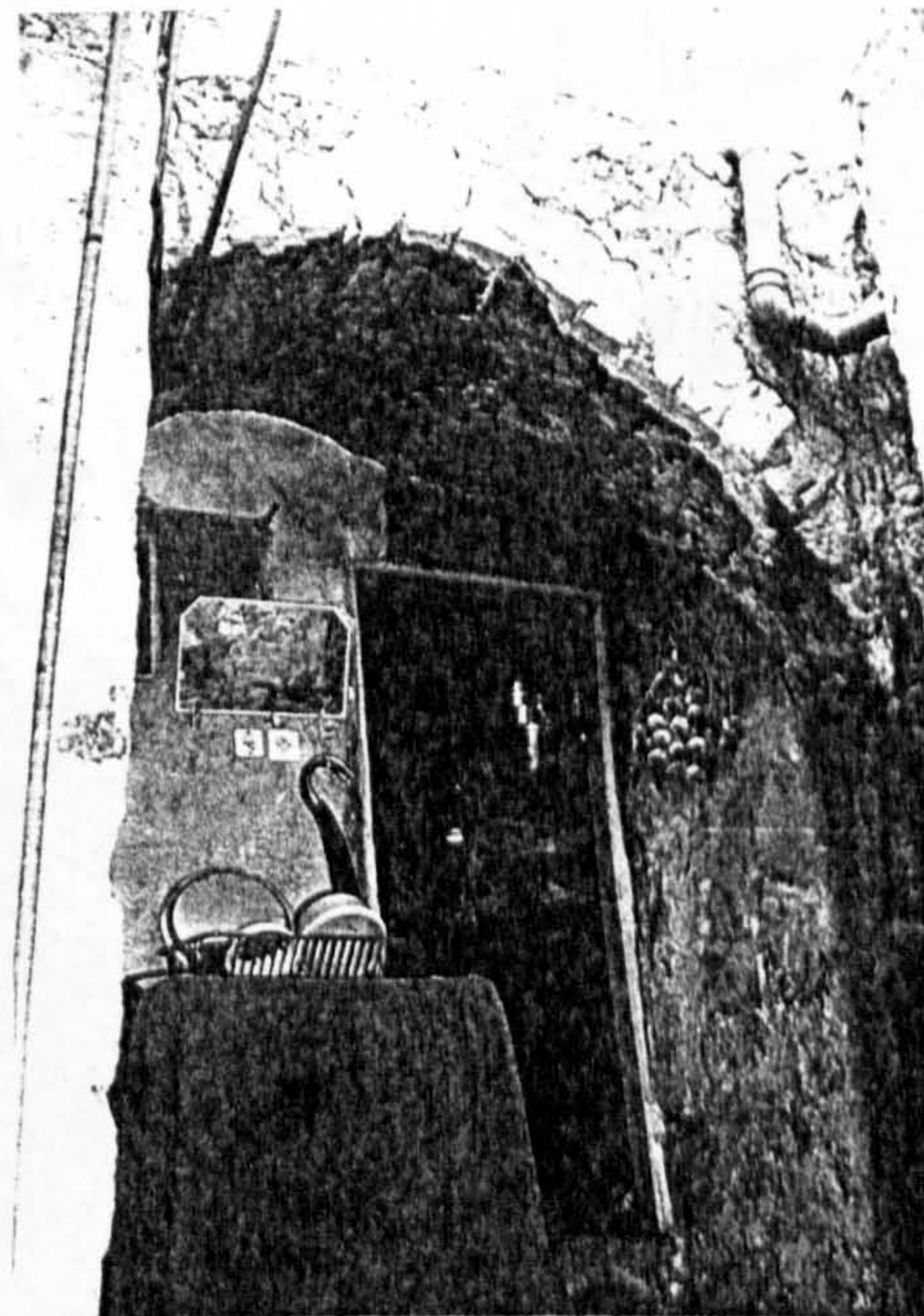
Plate (5.20): The kitchen of flat (5.GF2) at the end of this open court.
