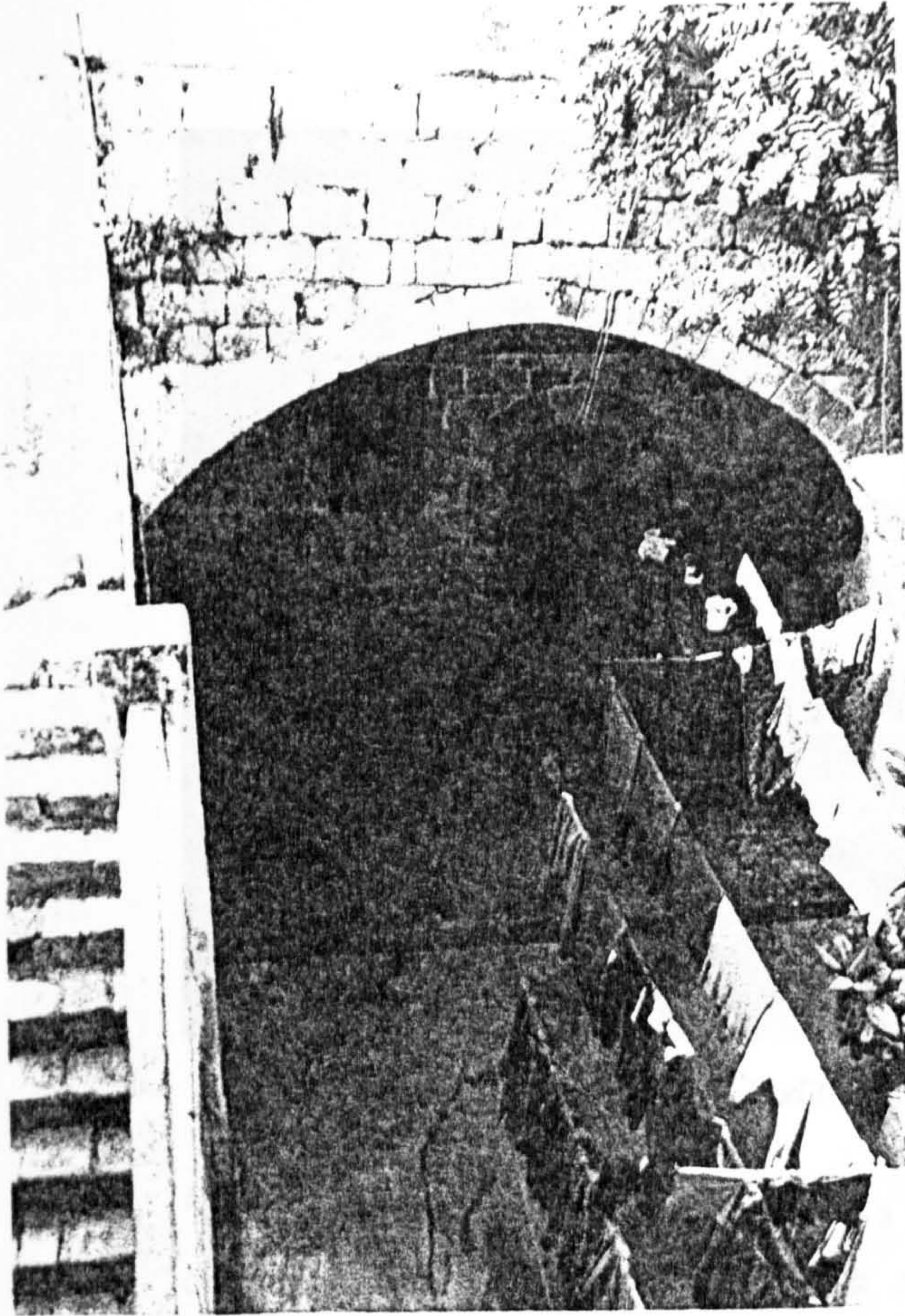
B. A courtyard within a middle-class house. Notice the covered and the un-covered parts.
