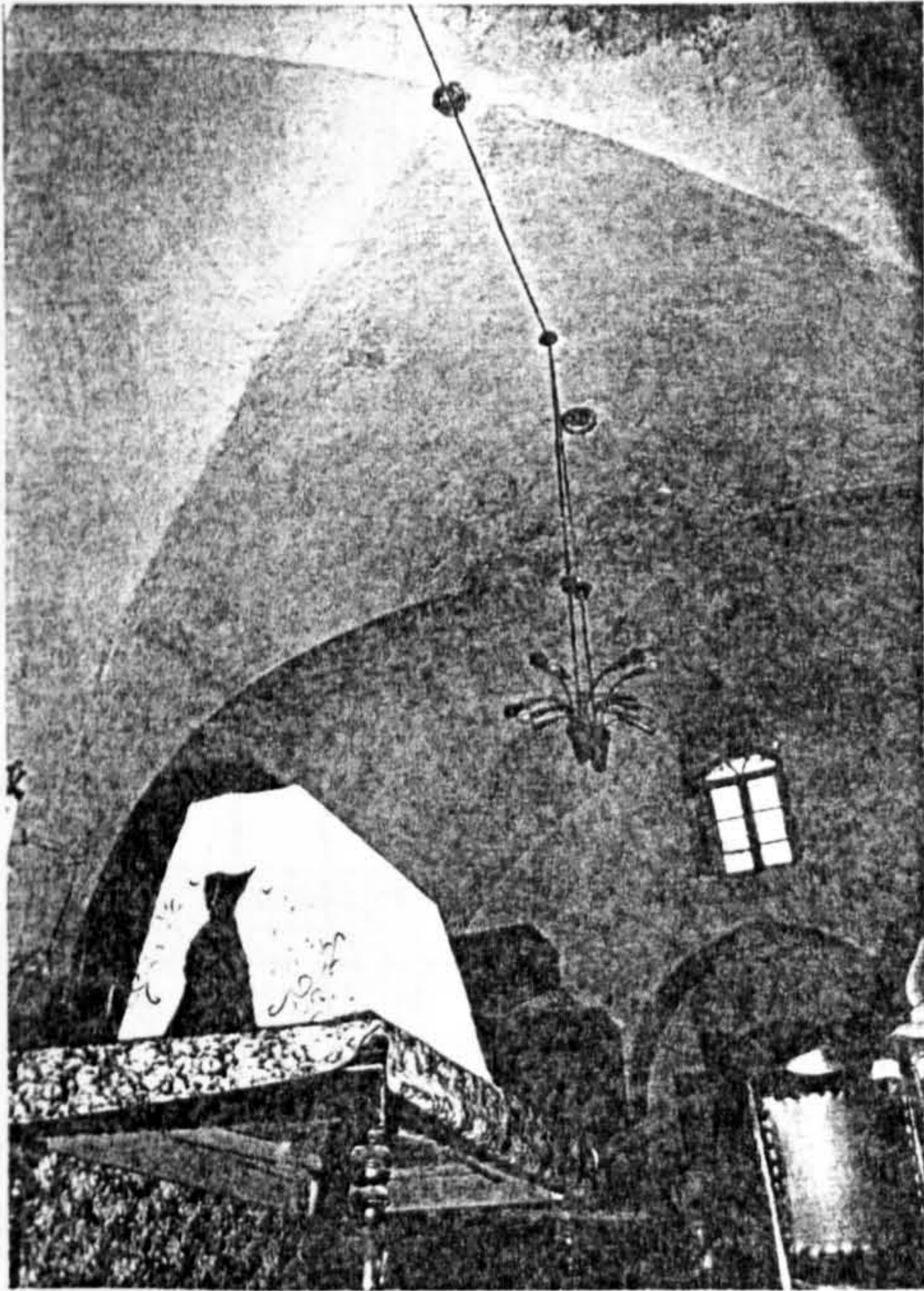
A. A cross vaulted room.
