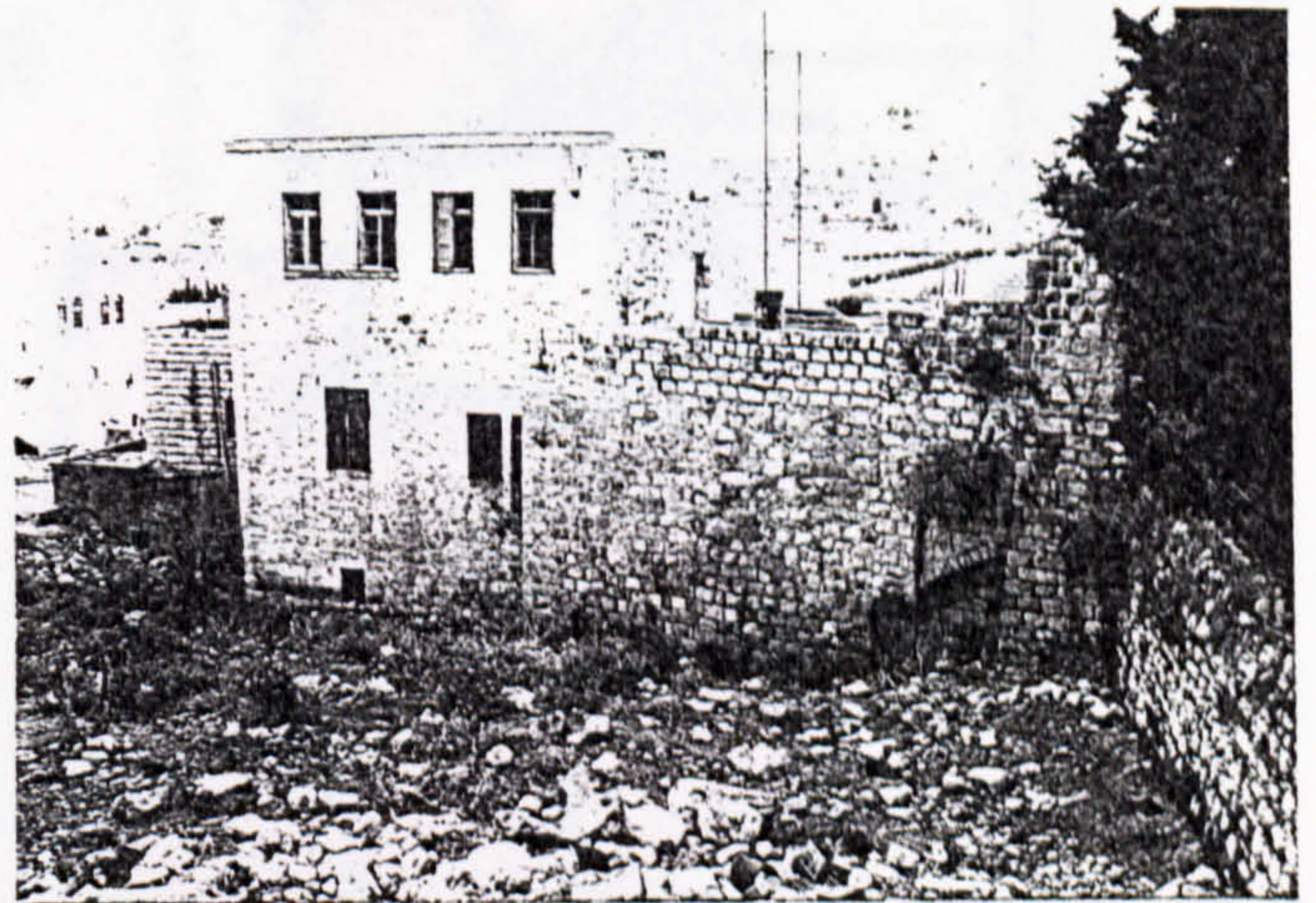
Plate (1.4): A closer look to the south elevation of buildings 1, 2 and 3.
