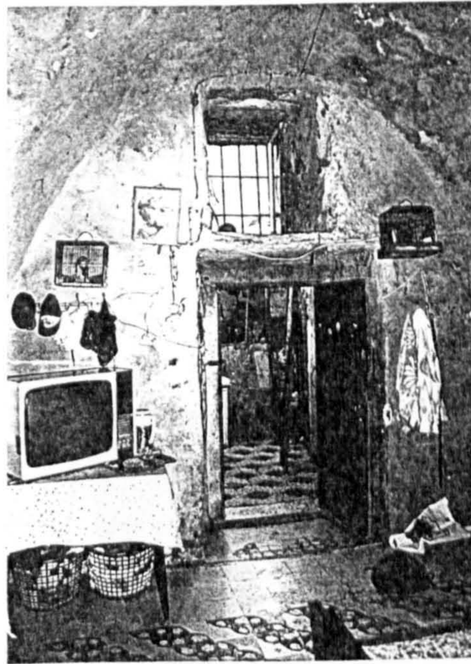
Plate (8.7): Interior of a bed setting room in flat (8.G3); notice the vault condition.
