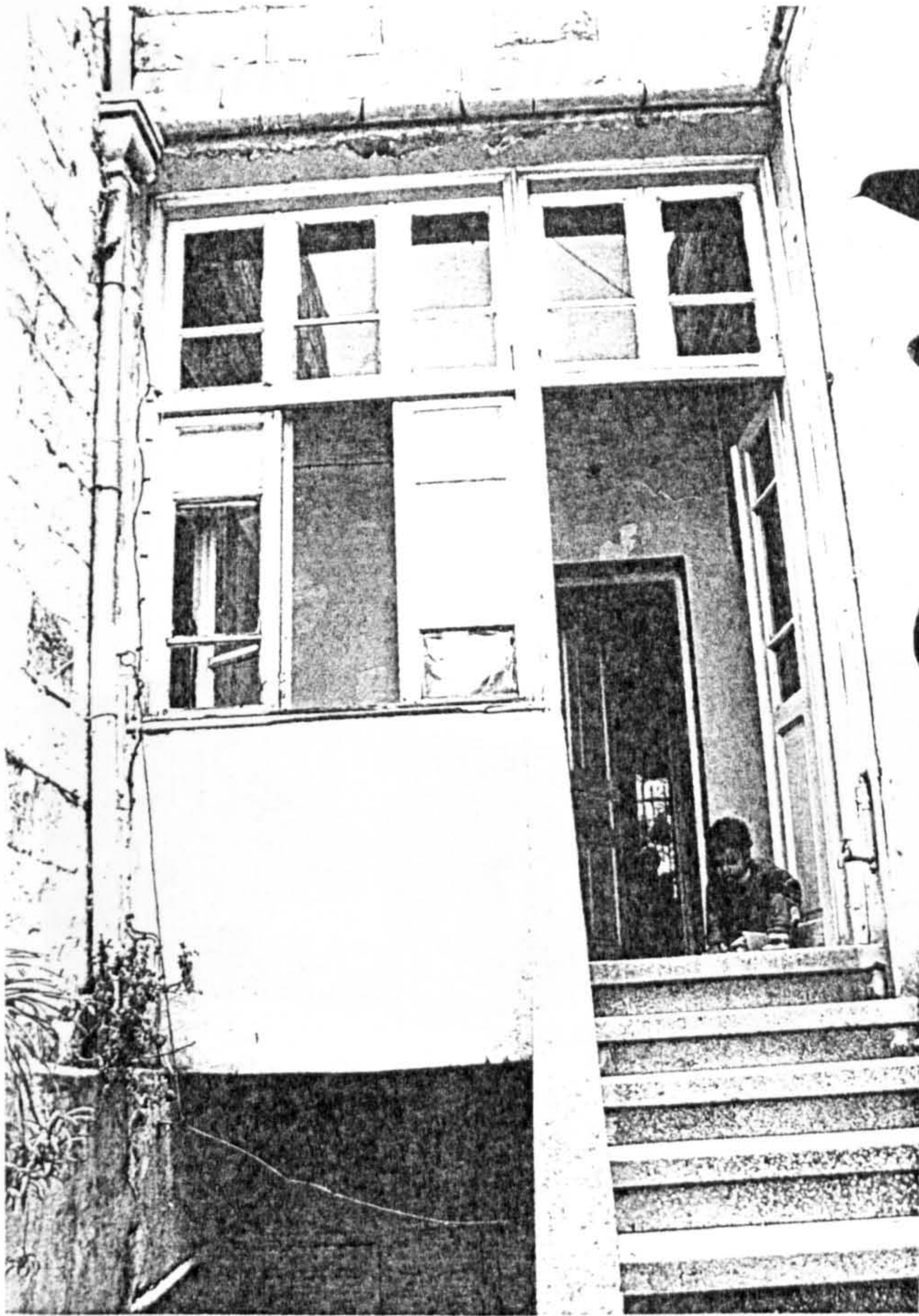
Plate (3.1) Uncovered staircase leading to the first floor.
