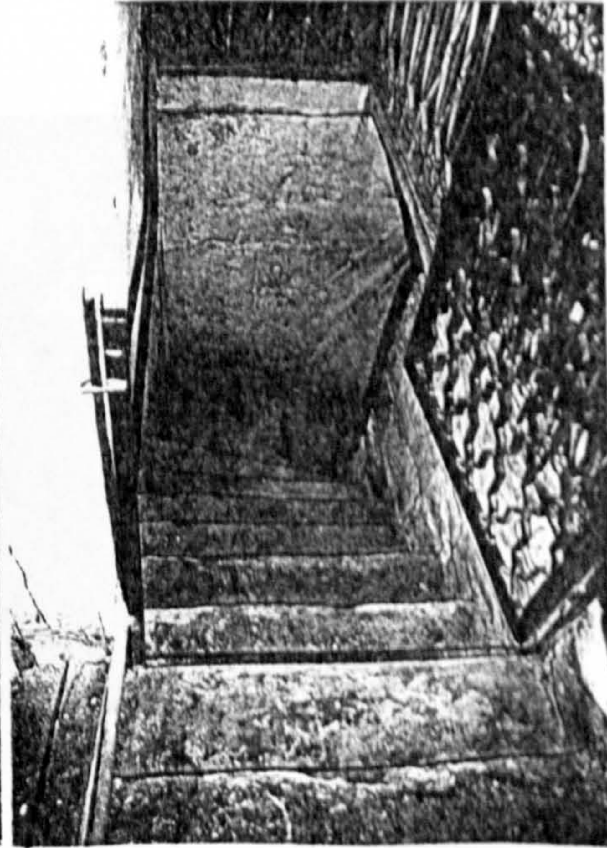
Plate (2.8): The top of the stair case leading to the first floor.
