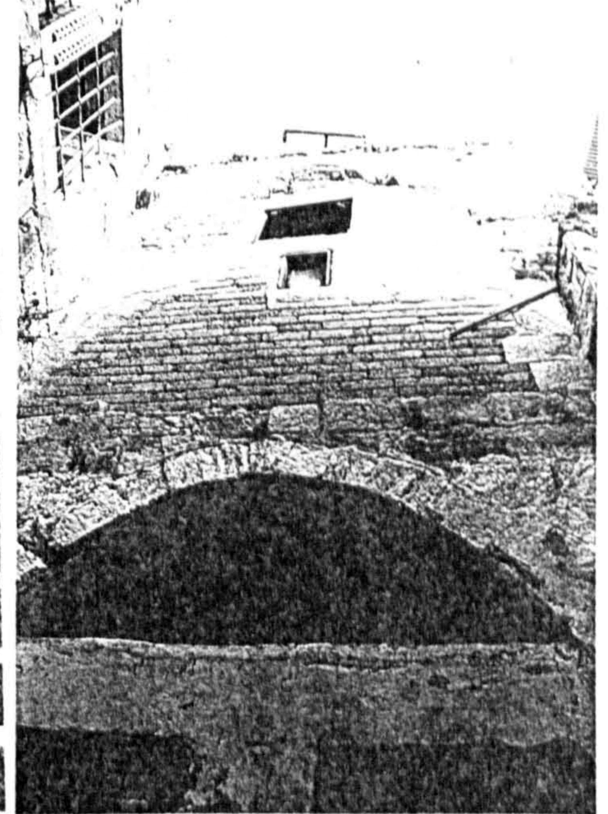
Plate (8.12): Looking upward from the court of flat (8.F3); notice the used building materials in closing the arch opening.
