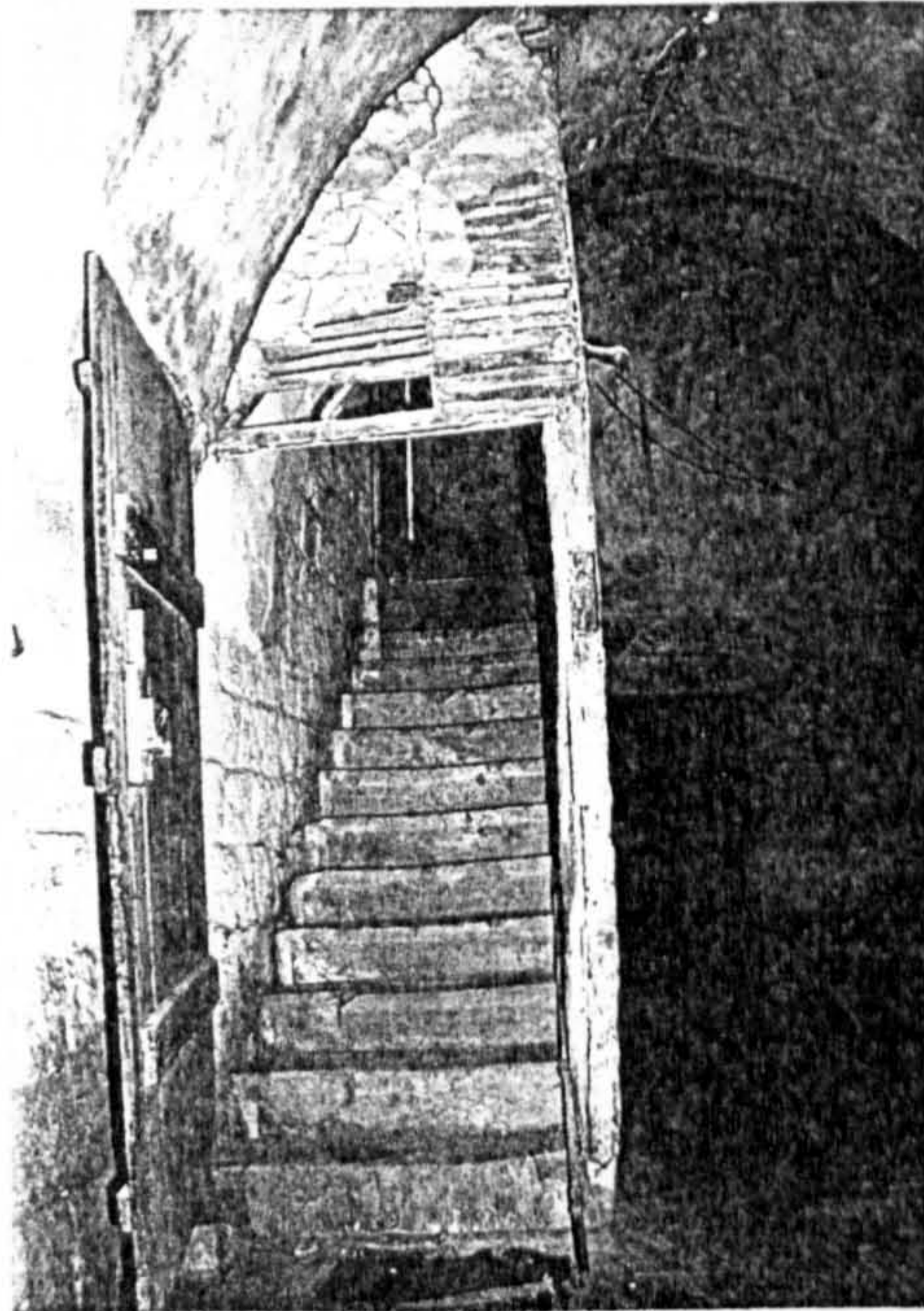
Plate (2.4): The upper floors stair case through the main hall; notice the bad condition.
