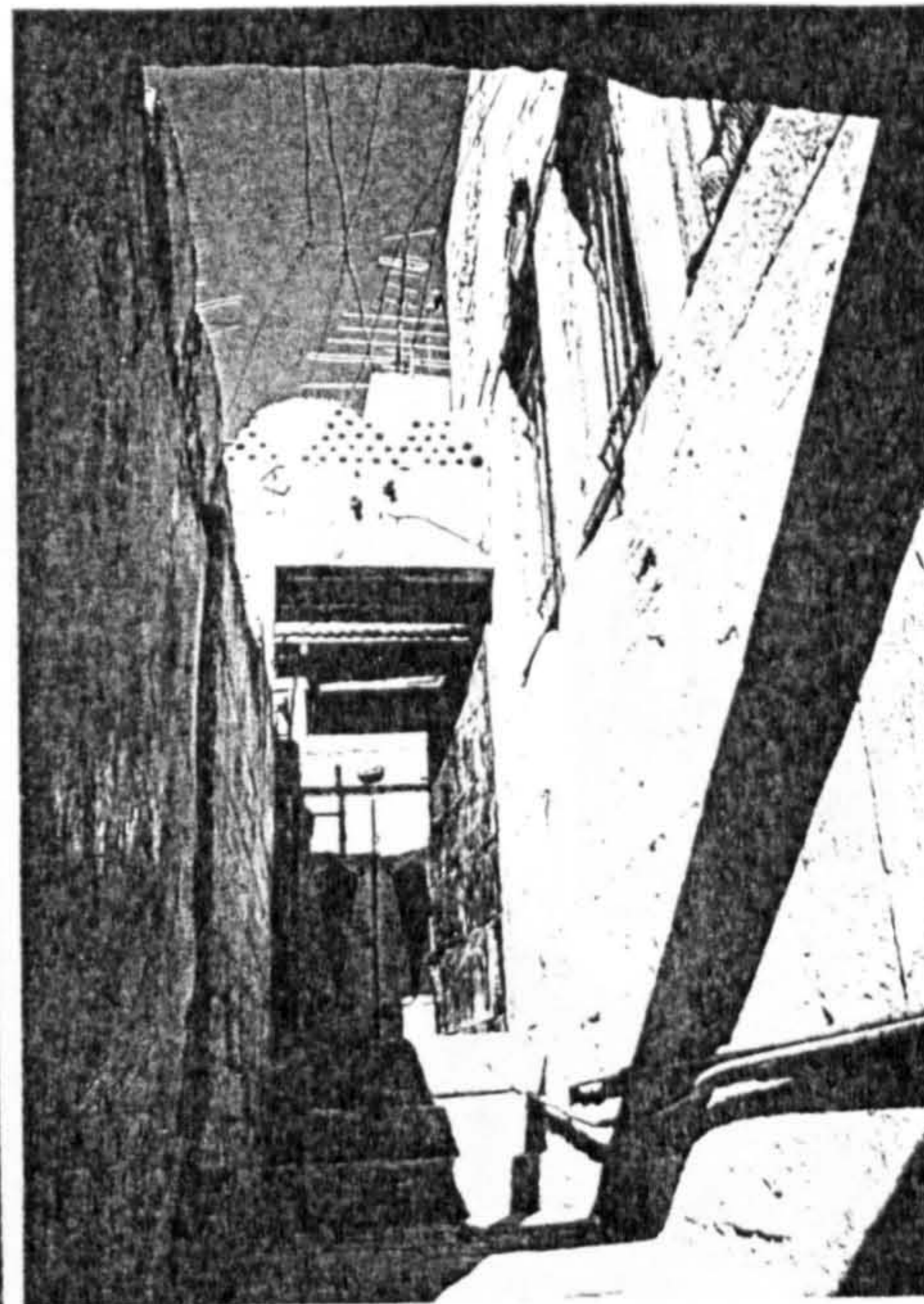
Plate (4.10): The stair leading up to the first floor flats; notice the high screen wall on the left.
