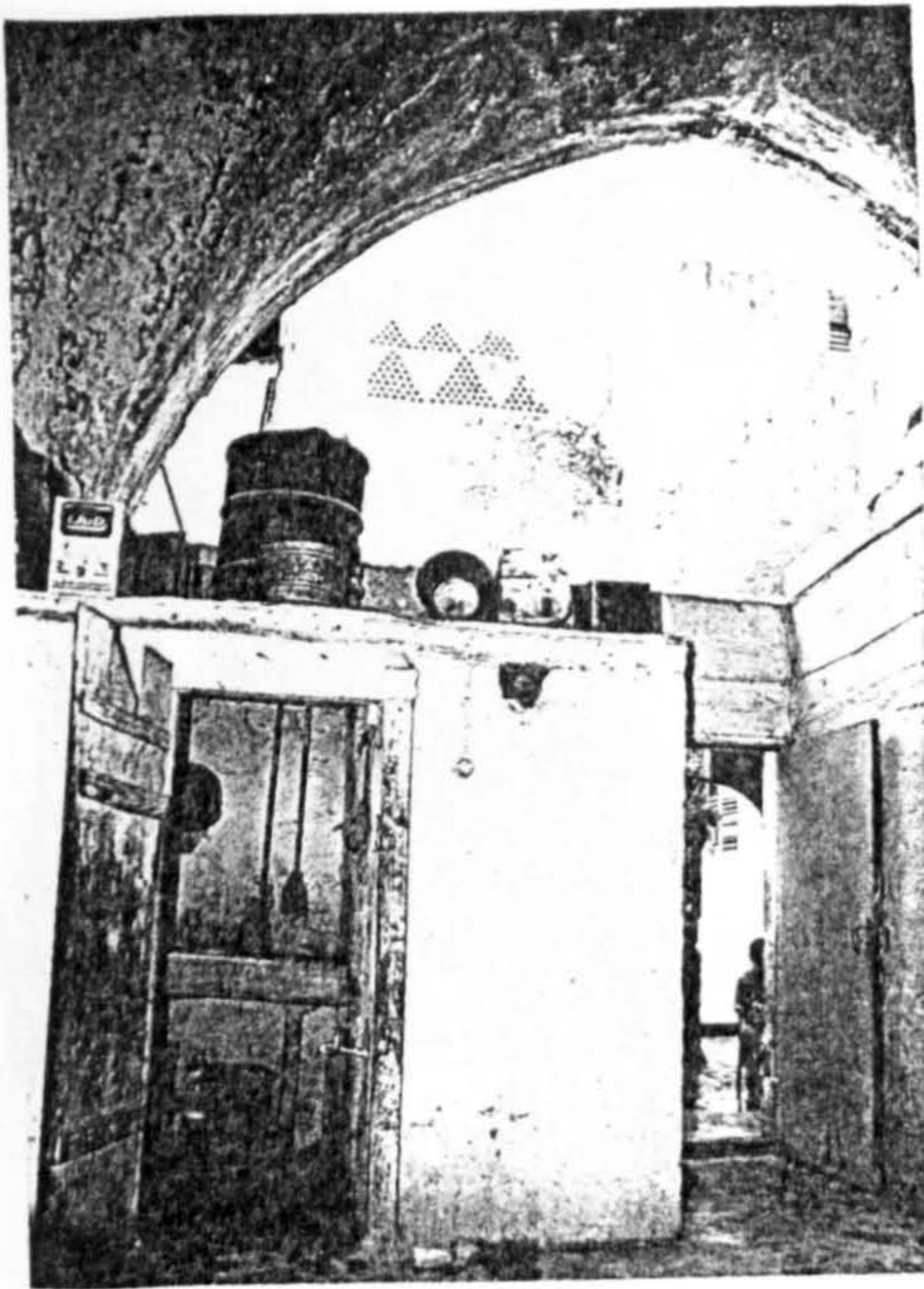
Plate (4.9): Entrance of flat (4.G4); notice the added toilet and bath room.
