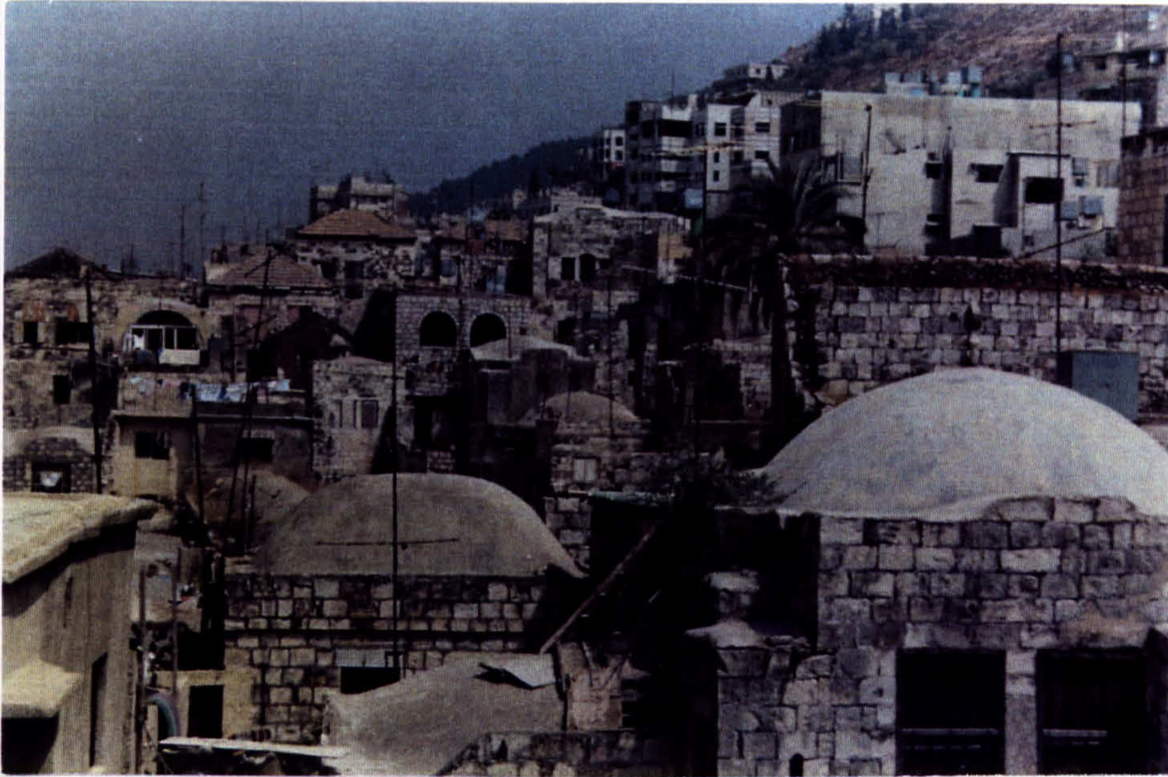
Figure (4.10): The traditional arched and vaulted structures of the Old Town. Source: Courtesy of An-Najah Univ. Arch. Students, 1989.
