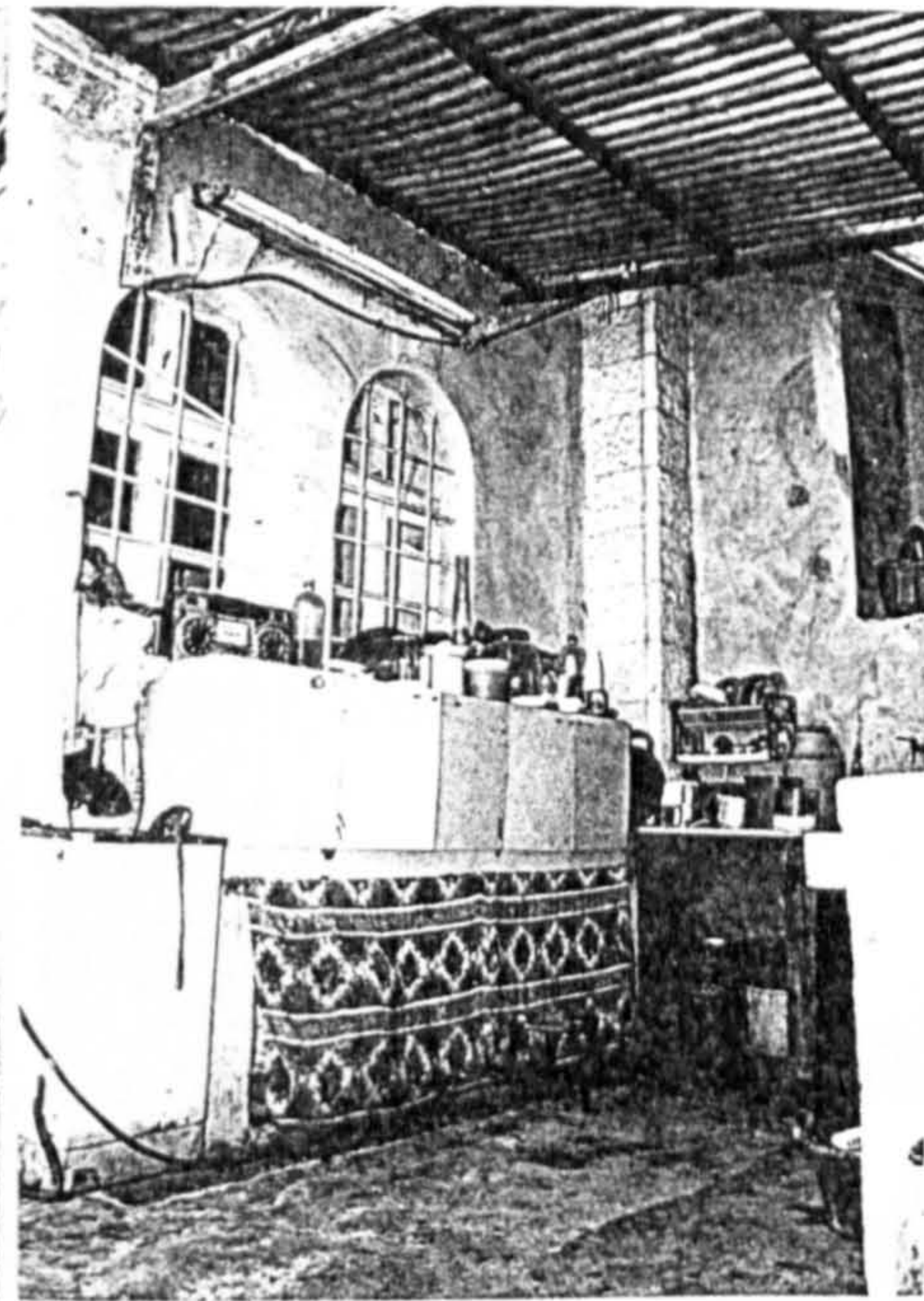
Plate (4.2): Kitchen of flat (4.G3); built within the main court of the building.
