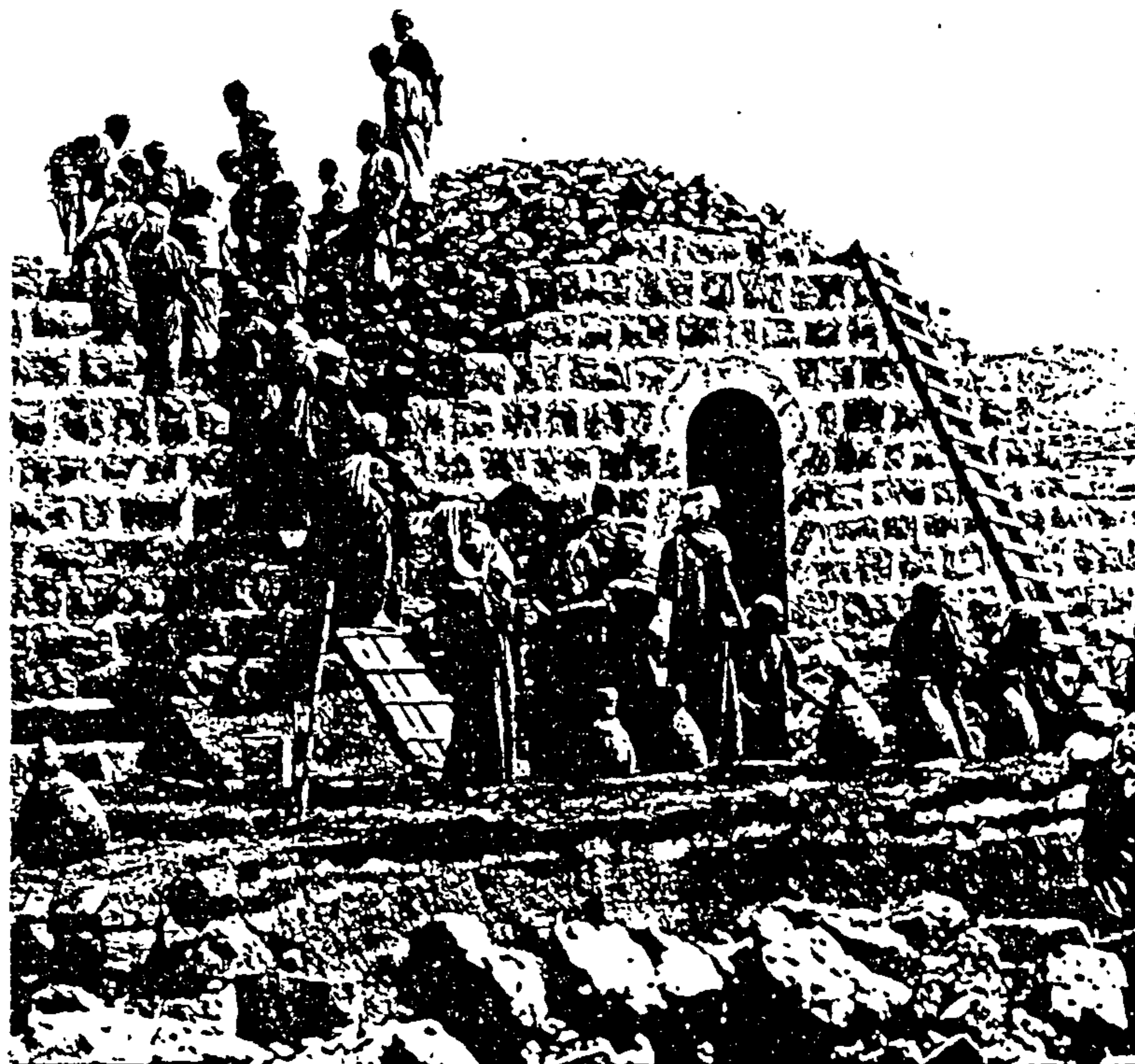
Figure (4.51): Building a traditional stone house in a Palestinian village.
