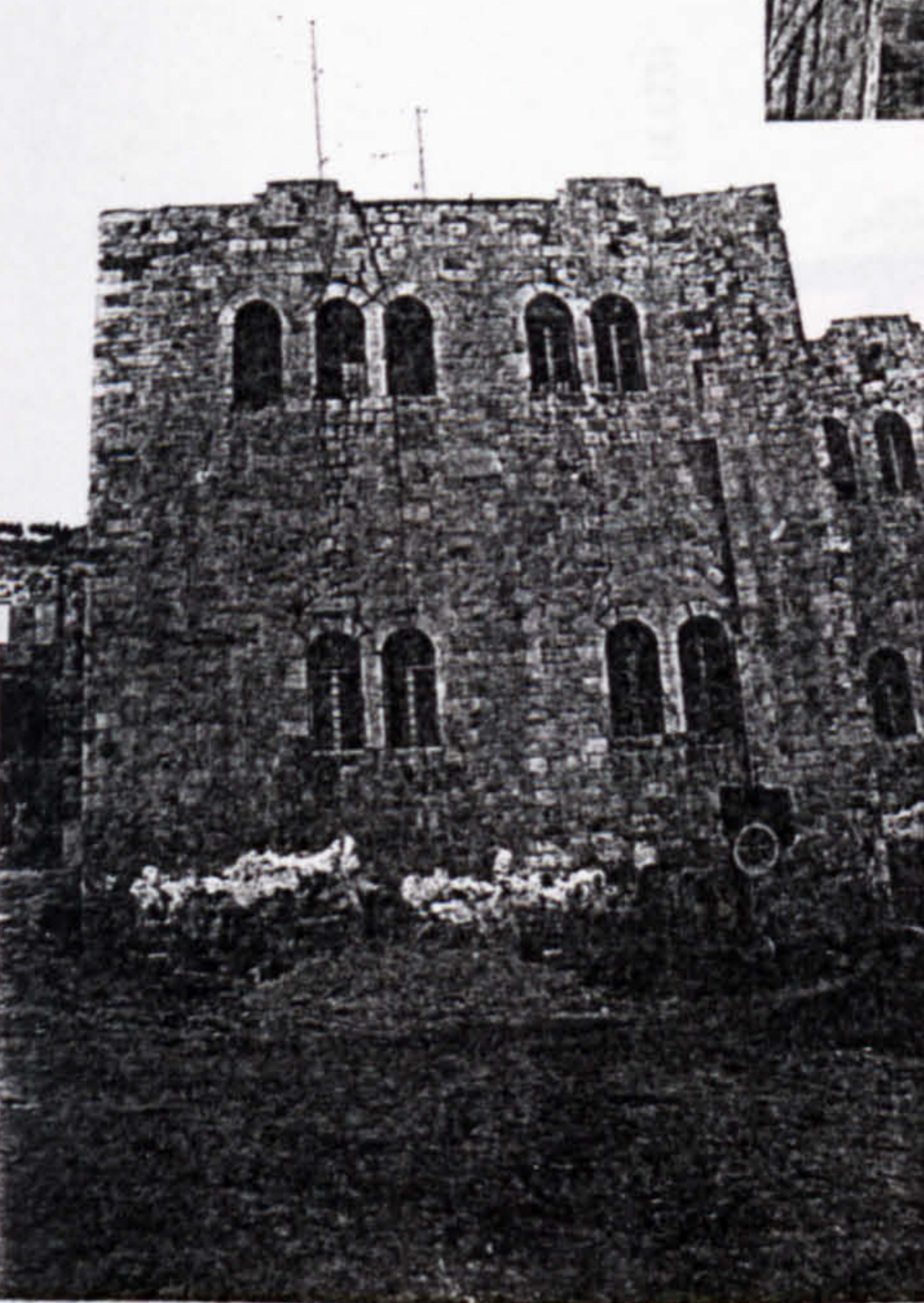
Plate (4.D): Part of the north elevation; notice the wall cracks.
