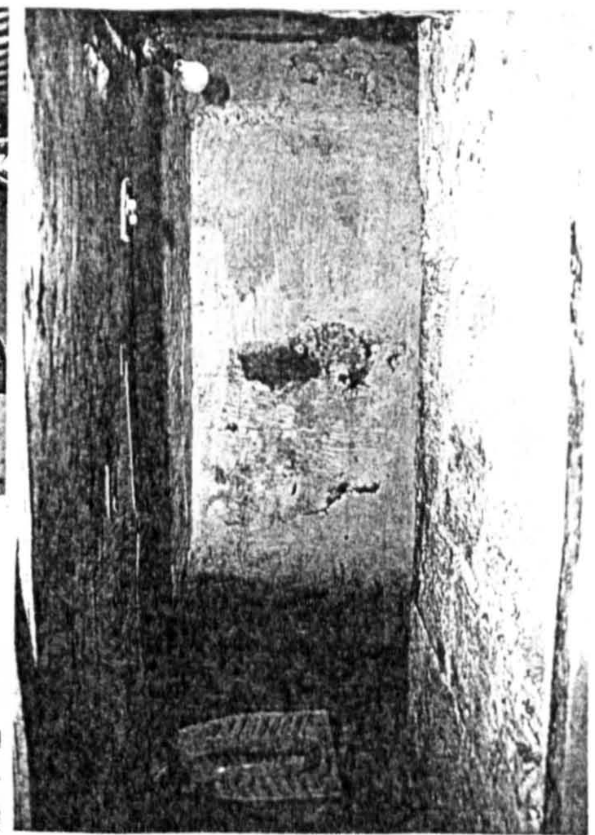
Plate (4.3): WC. of flat (4.G3); built under the first floor stair.
