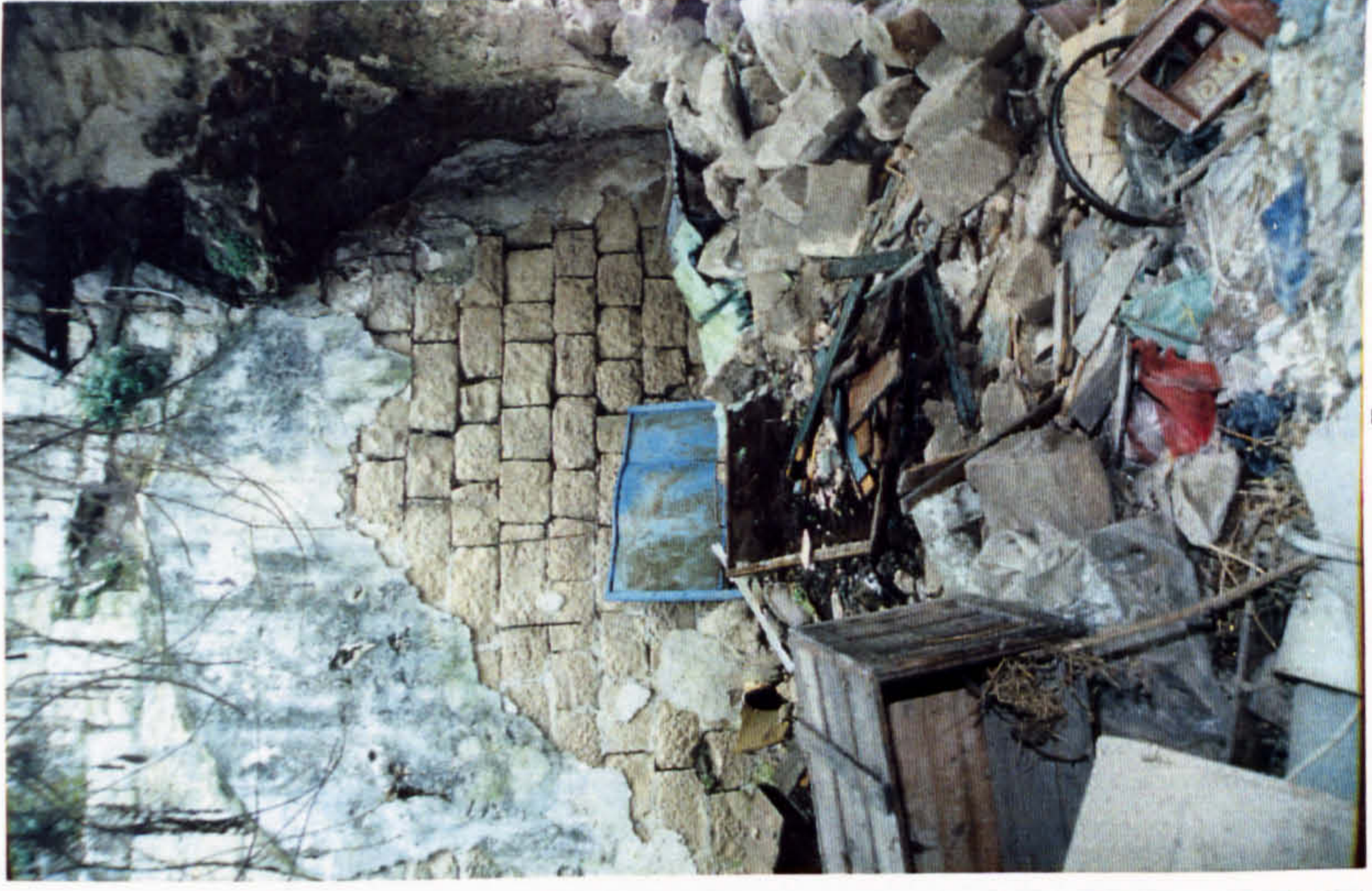
E & F. The effect of using explosives on neighbouring buildings to demolish one housing unit among the highly concentrated built environments of the Old Town. Source: Courtesy of Mr Tibawi, 1989.
