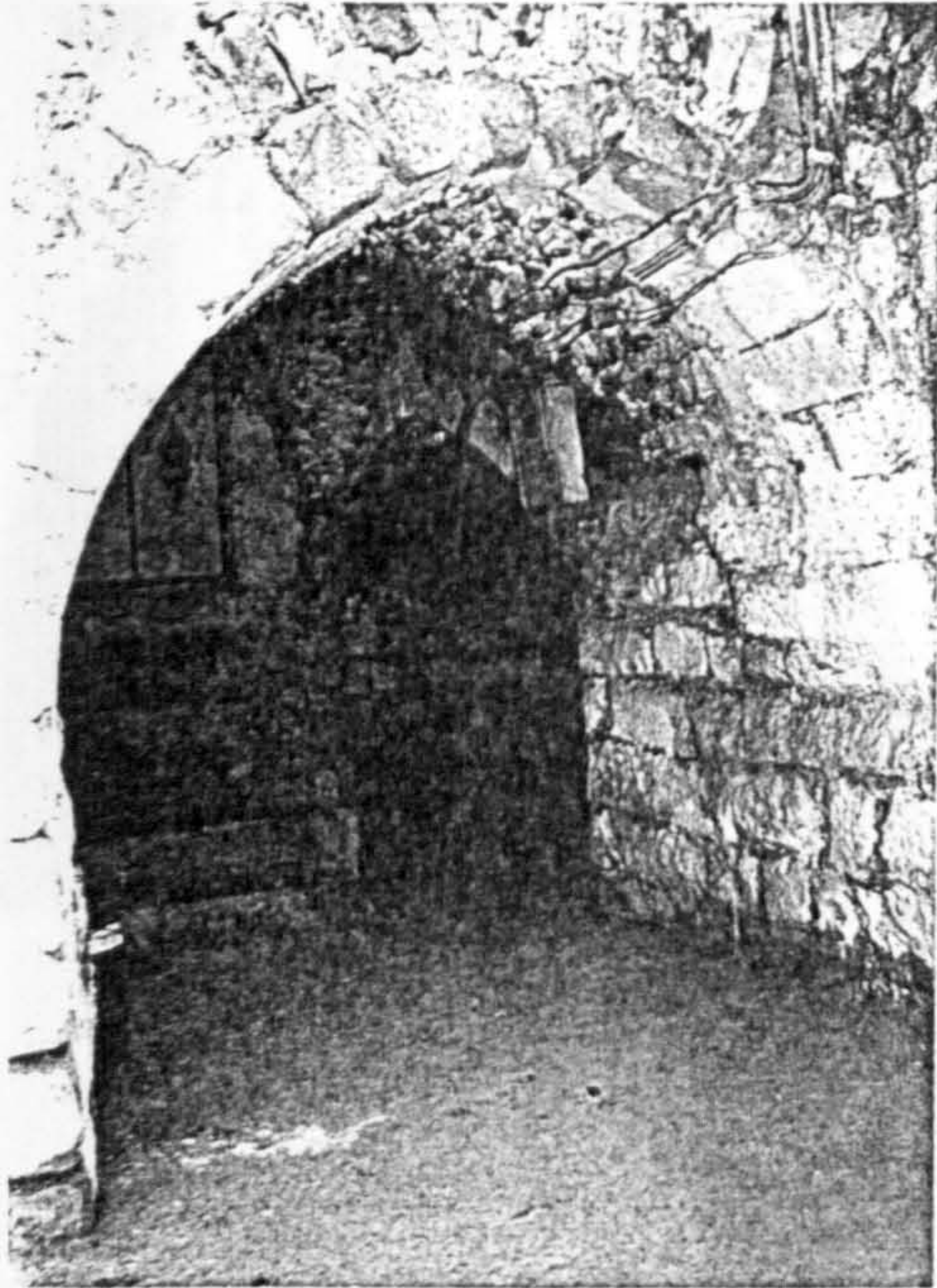
Plate (5.10): Approaching the entrances of the two flats (5.GF2) and (5.GF3).
