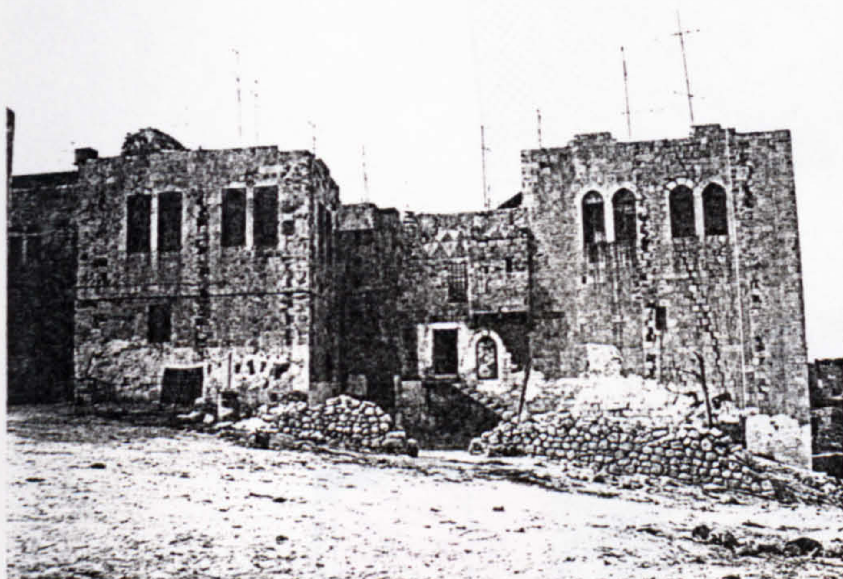
Plate (4.A): East elevation; notice the walls' cracks.
