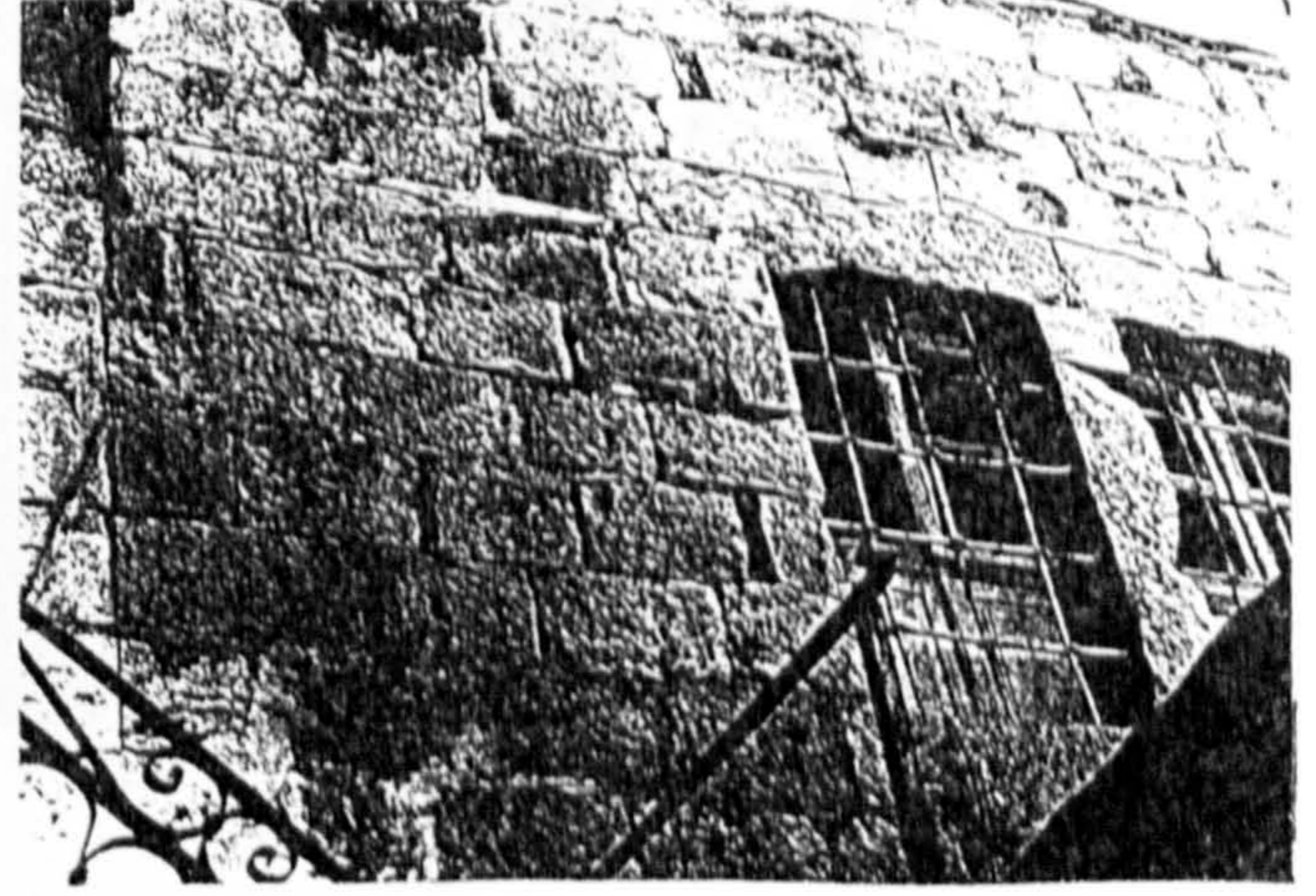
Plate (8.23): A stone wall near the entrance of flat (8.S3); notice the condition of stone units and the mortar.
