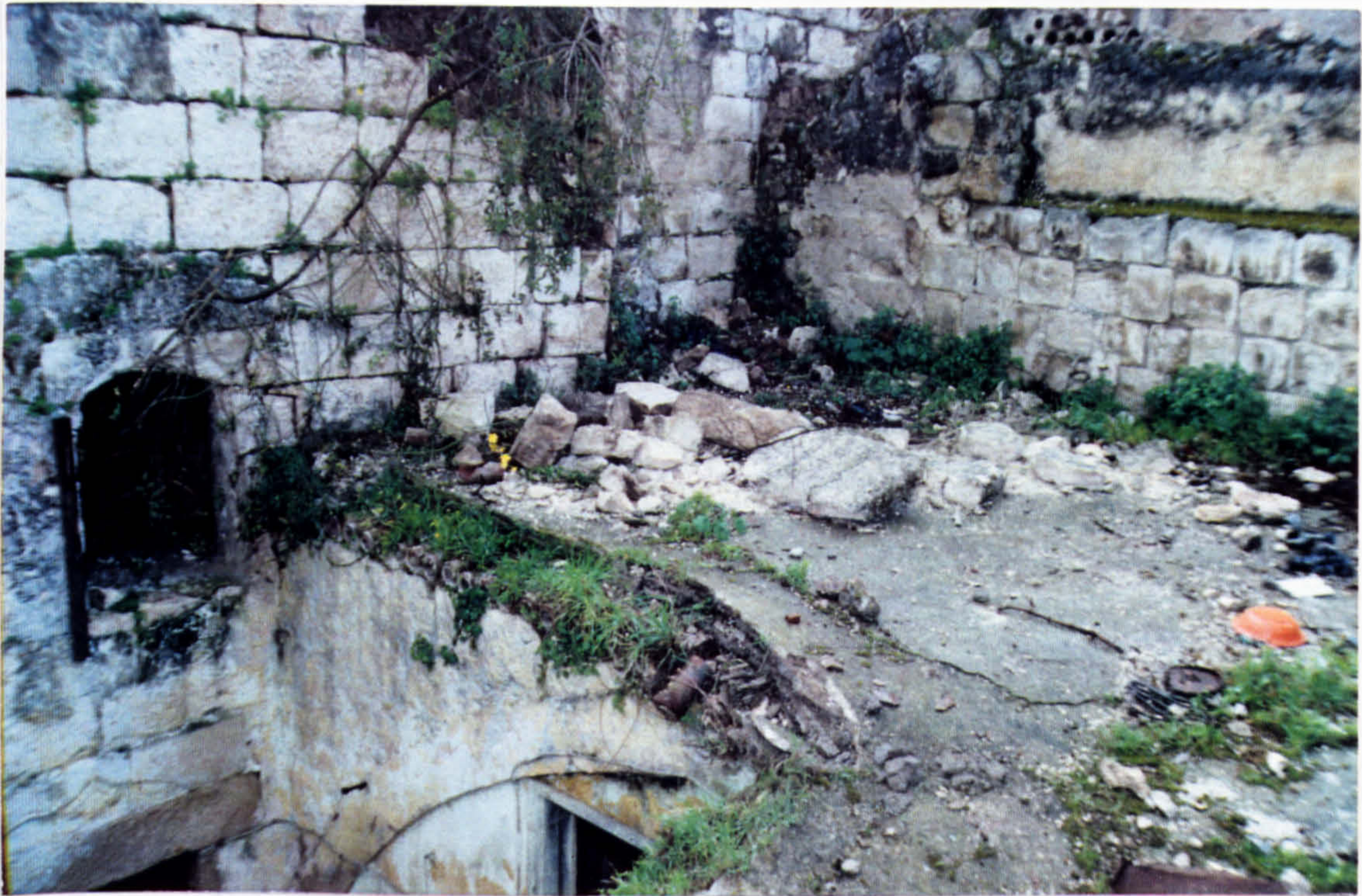
Figure (5.14): Neglect effect on growing creeping plants within the historic buildings of the Old Town. Source: Courtesy of Mr Tibawi, 1989.
