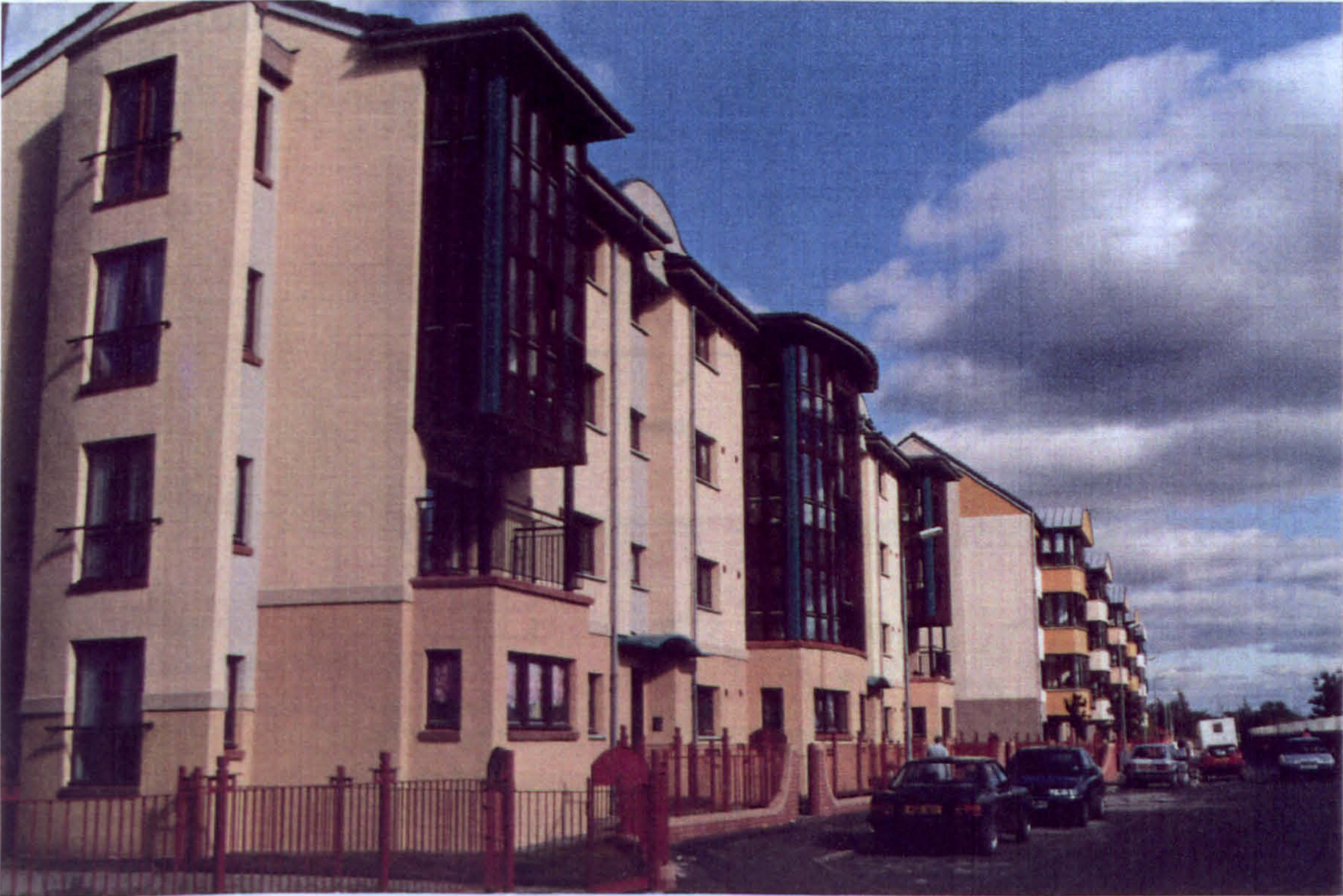
Terrace extended on south elevation to give choice of conservatory enlarged livingroom or balcony
