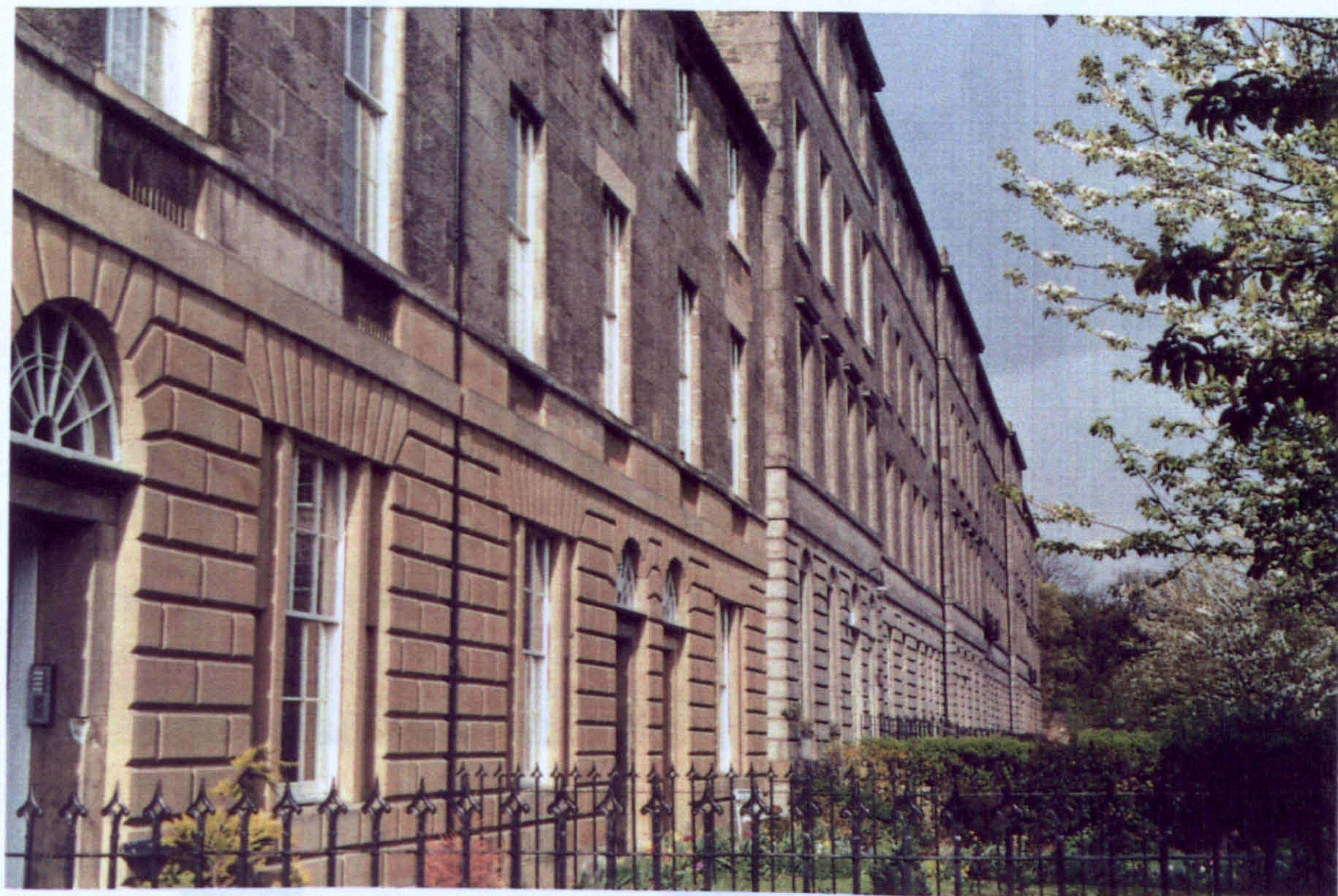
New stone facade to ground floor where shops removed.
