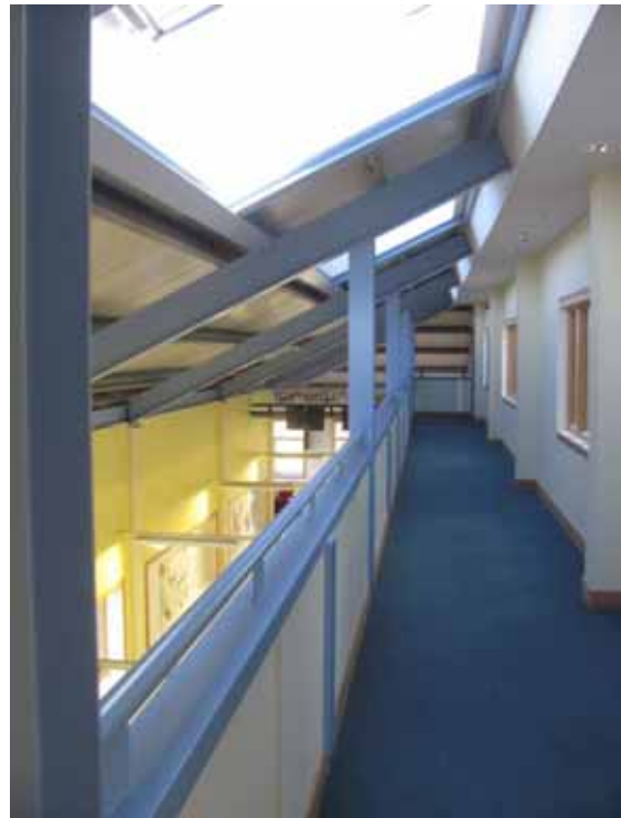
Figure 5: Internal view of first floor gallery, roof lights provide daylighting to gallery and ground floor. The windows on the right allow borrowed daylight in to the main hall.
