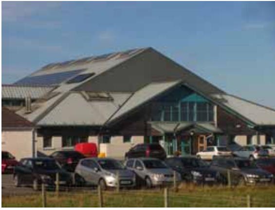
Figure 1a: External view of new-build community resource, Sporsnis, Ness, Isle of Lewis. Solar PV array, solar thermal and rooflights visible from higher ground near the site.
