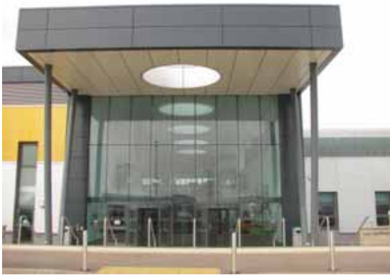
Figure 2a: External view of Banff and Buchan College, Fraserburgh. Solar installation not visible from ground level.
