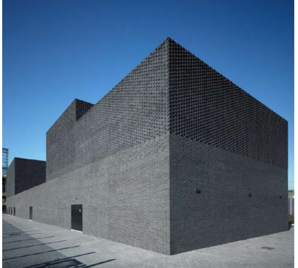
Completed Substation - photographic record of completed building
