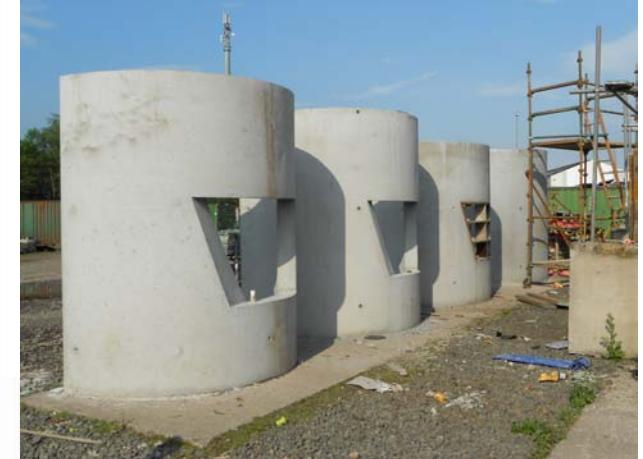
*Design in detail, full size mock-ups of the driven voids and top: the 'thin skin' glass shroud*
