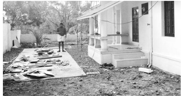
Figure 4: The tank as constructed on site.
