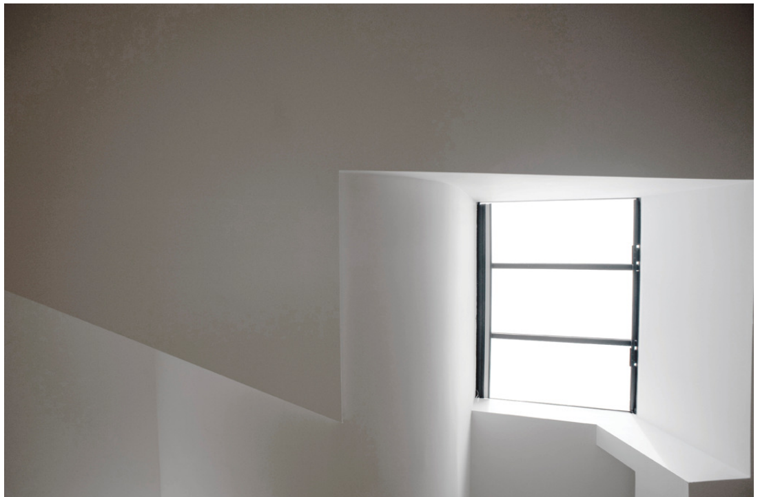
View of rooflight
