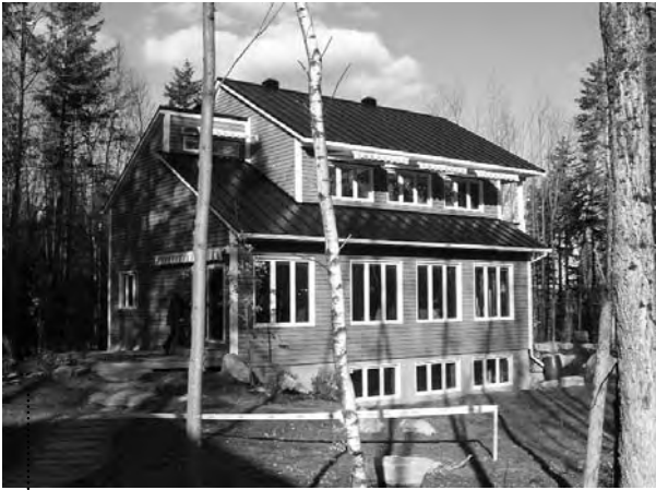
Figure 1. The first EQUilibrium sustainable house built in Canada
