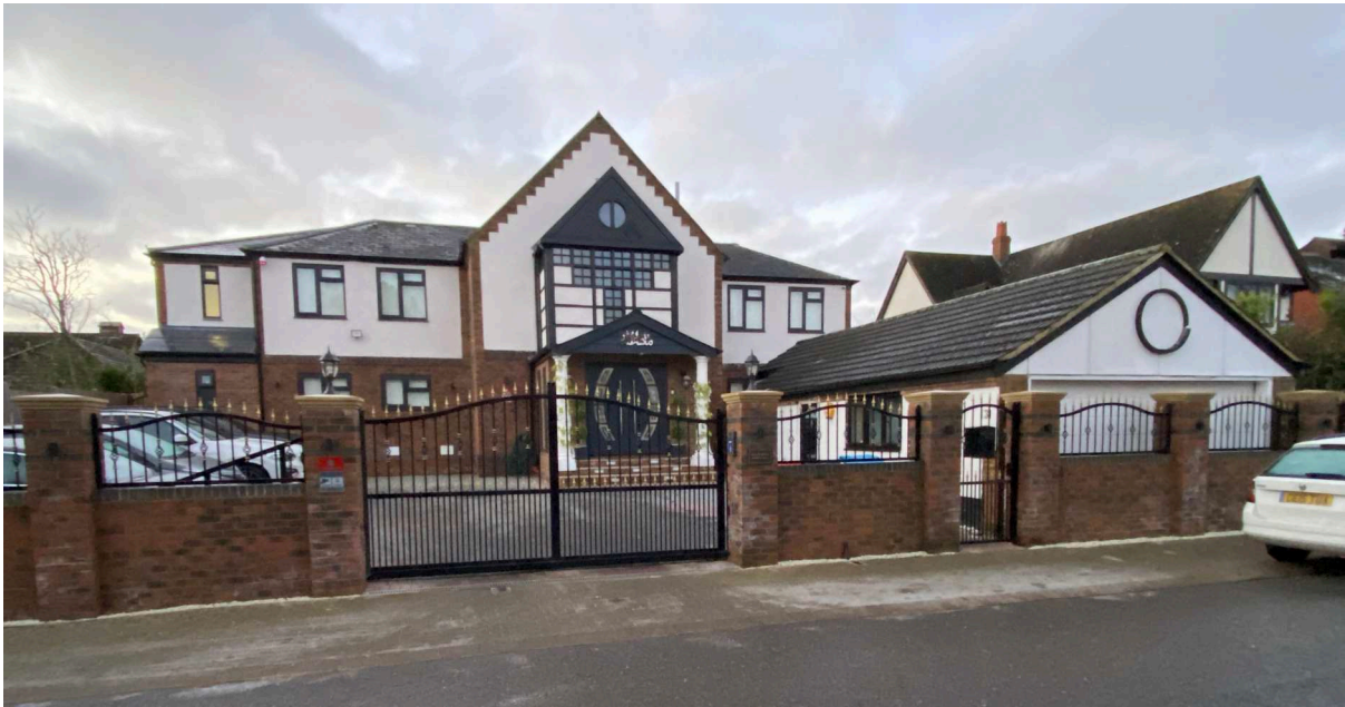
Figure 17. Pilkington House, 1986, designed by Derek Walker, photographed by the author, 2024
