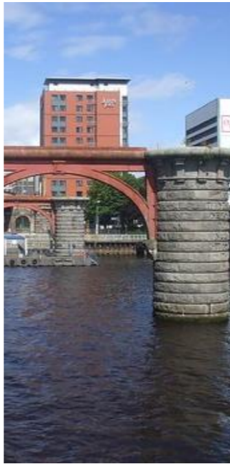
Urban River Tidal Weir
