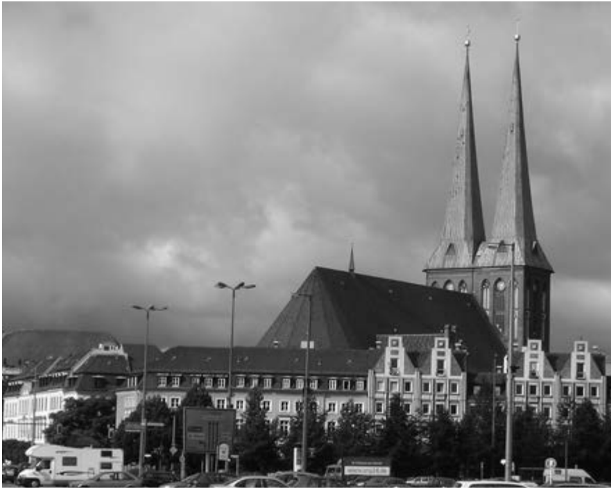
NIKOLAIVIERTEL, EAST BERLIN (1979–1987, GÜNTER STAHN AND OTHERS). IN THE BACKGROUND IS THE REBUILT ST NICHOLAS CHURCH FROM THE THIRTEENTH CENTURY, IN THE FOREGROUND, NEO-HISTORICAL FAÇADES FROM PREFABRICATED ELEMENTS.
