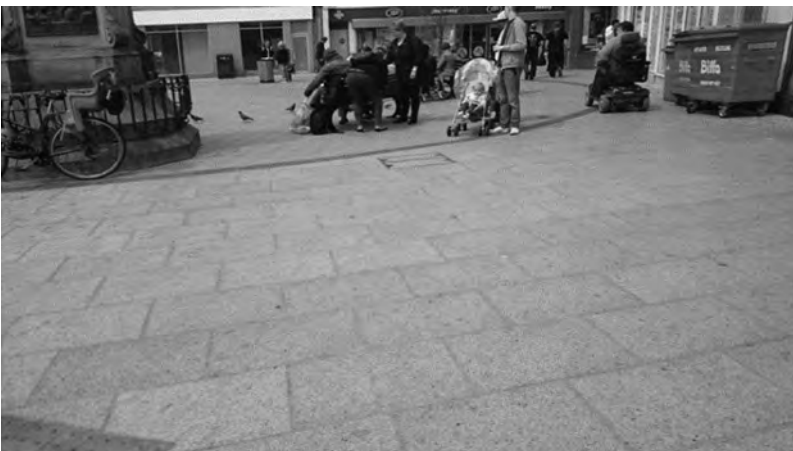
Figure 14. The new pavement at the foot of Leith Walk (LTC). Source: L. Brunelli.
