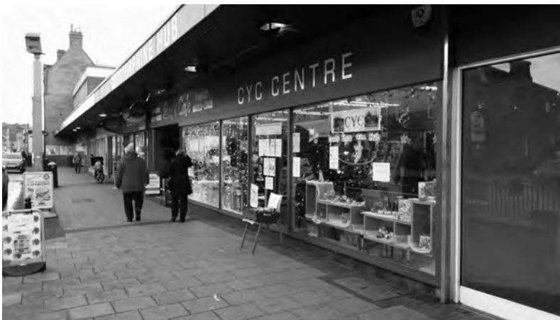
Figure 16. The provisional community centre in CTC, 2016. Source: L. Brunelli.
