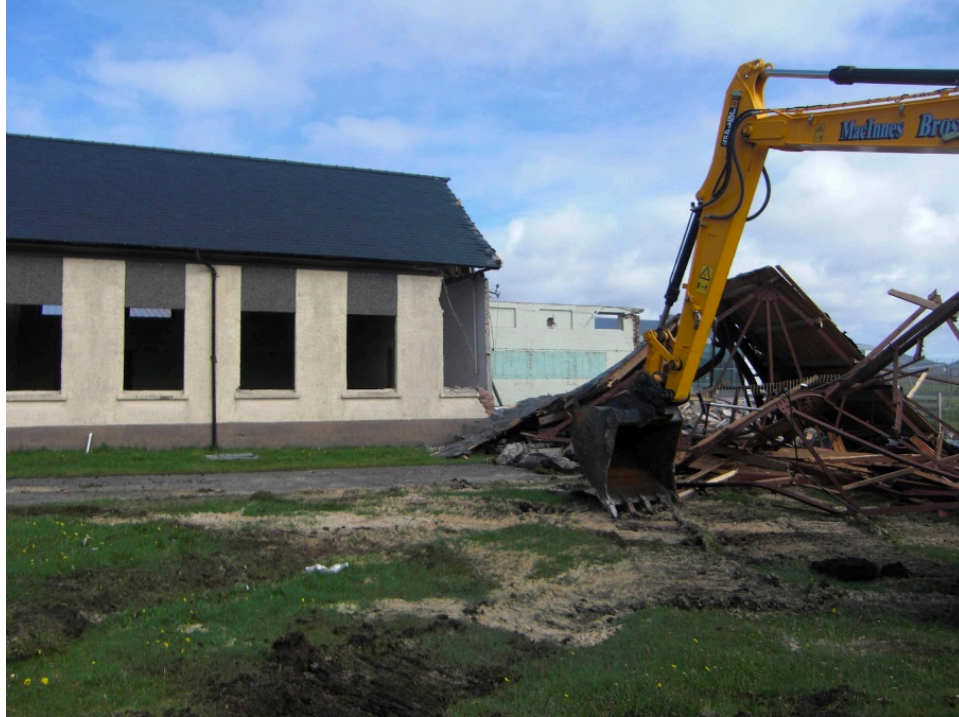
Figure 14: Paible school demolition (Hebrides News, 2011)
