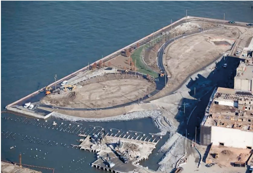
Figure 13: Pier 1 during development
