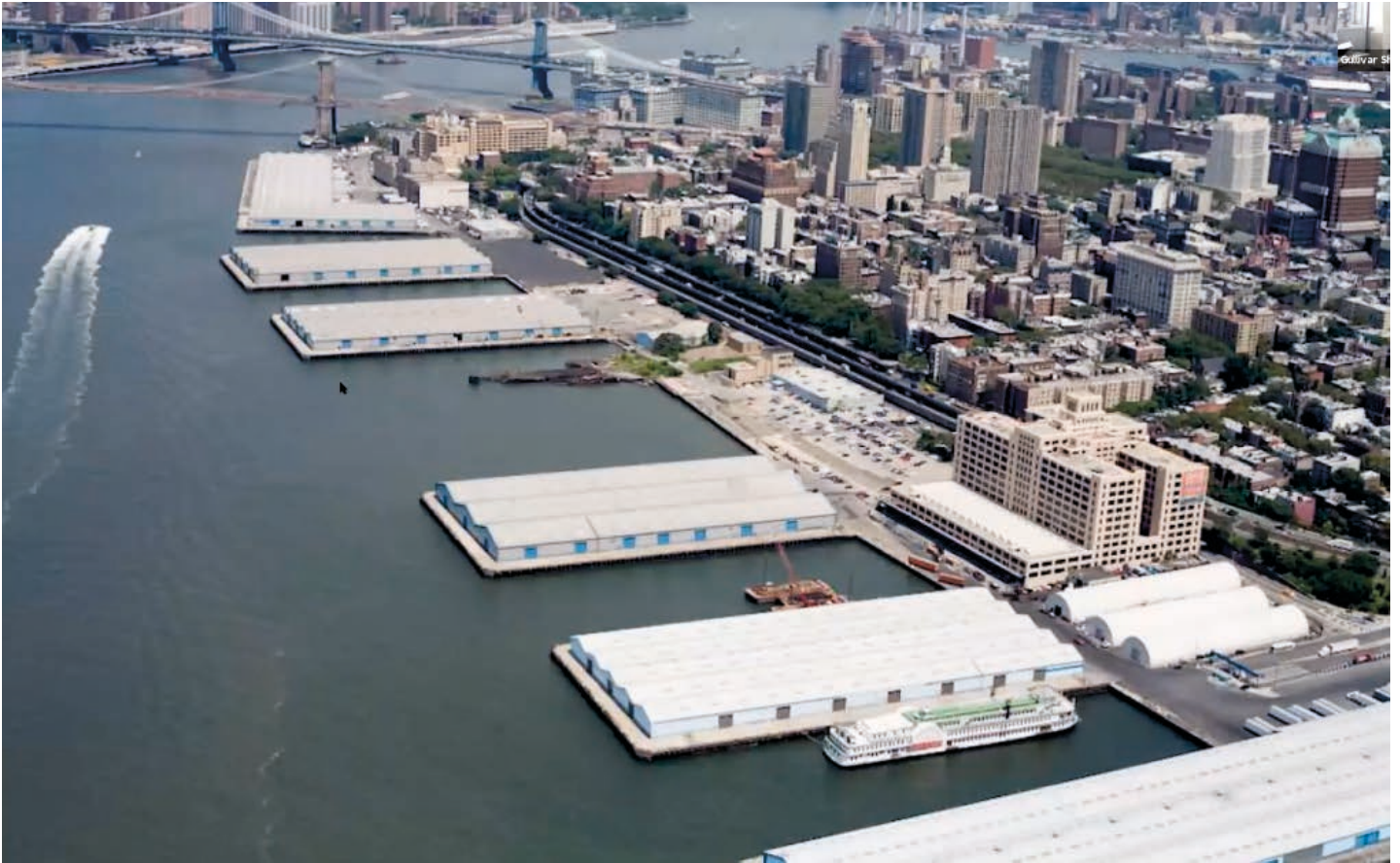
Figure 3: The site 20 years ago
