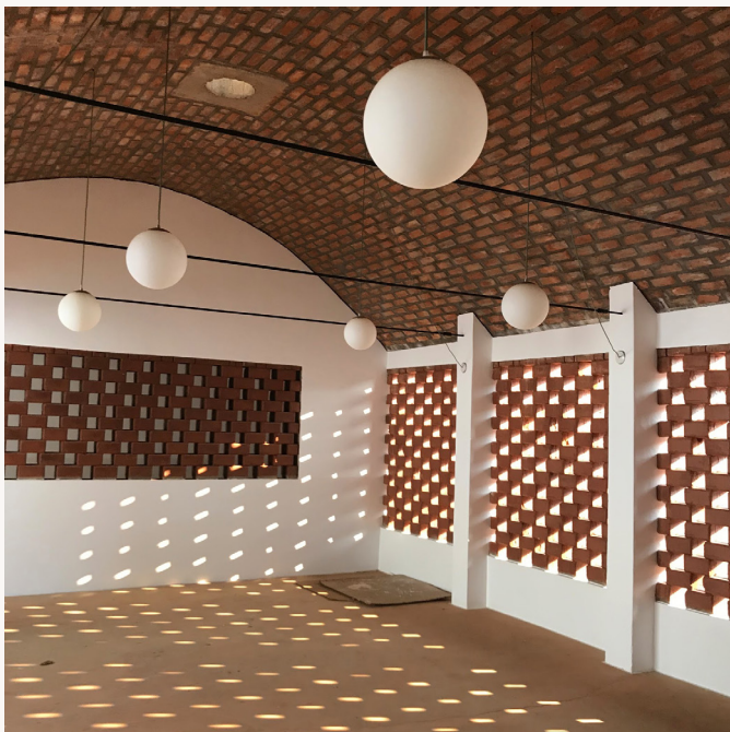
Image: perforated brick walling at the Sachibondu Hospital in Zambia by BuildX Studio
