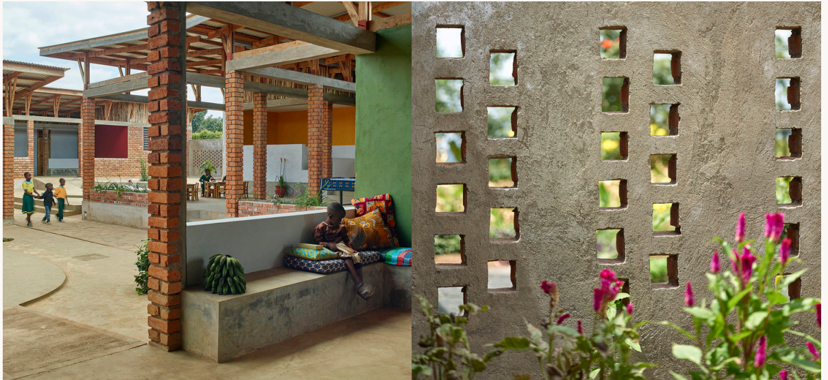
Figure 22. Open brickwork as perimeter walls maintain the contact with the surroundings.
