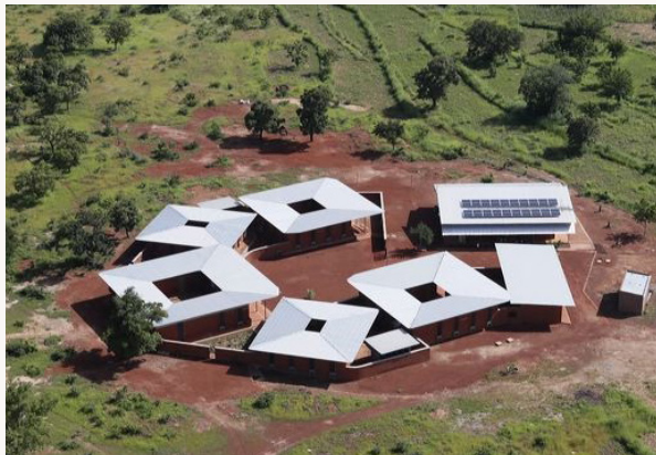
Figure 19. Aerial picture of Noomdo Orphanage showing the placement of the buildings.
