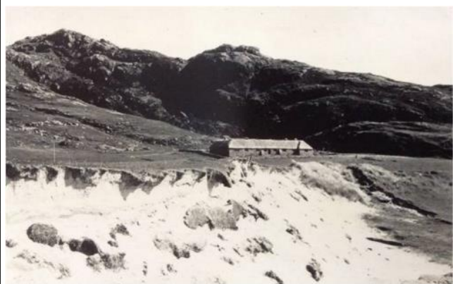
Figure 4: Violet Banks, House at Sanna built by M.E.M. Donaldson , c.1920s, HES PA23815/4. © Historic Environment Scotland Collections
