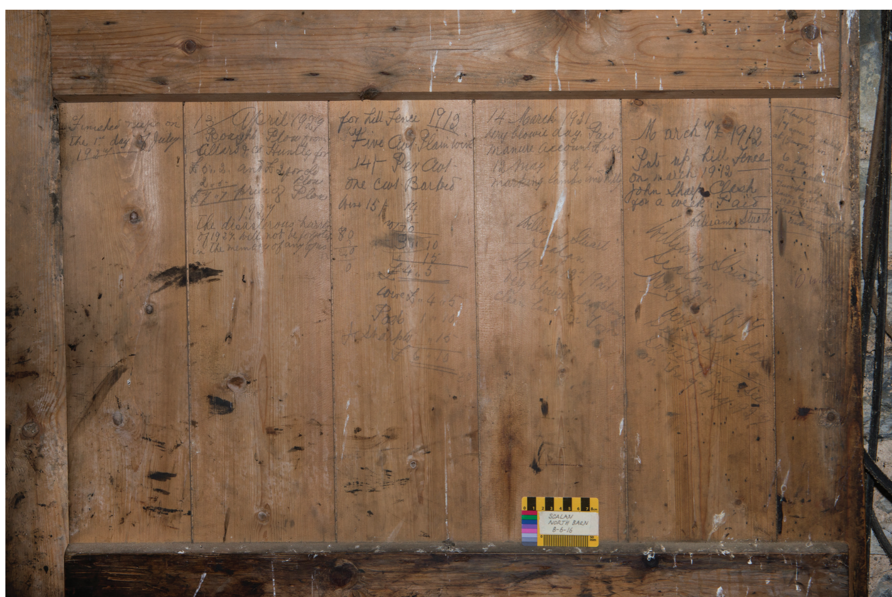
Scalan North Barn, (2016). Copyright: HES DP 242895
