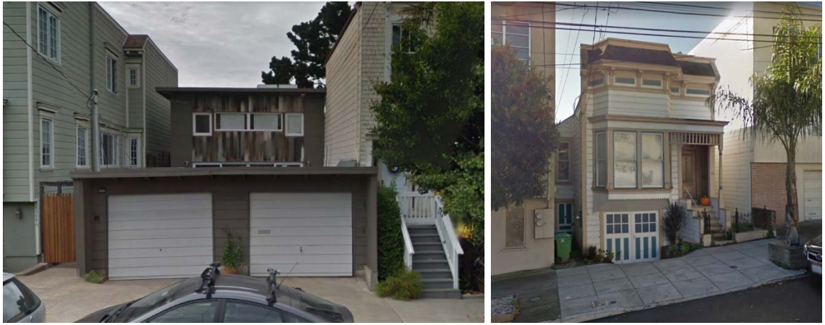
Figure 6.3 Front façades of the SF-PH (left) and SF-CO (right). Source: Google Maps 2018.
