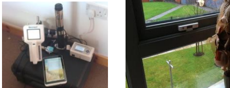
Figure 2: Portable monitoring apparatus and installed t-mac wireless contact sensors at windows
