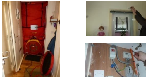
Figure 3: Air Pressure Testing fan in dwelling door (left); and air leakage smoke tests at windows, pipe routes etc.
