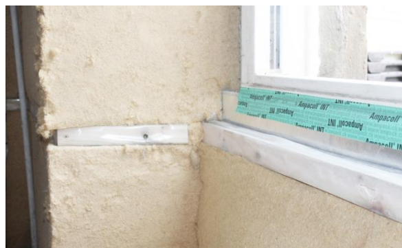
Figure 3: Internal wood-fibre insulation, which aims to provide active moisture control working in combination with the demand control mechanical ventilation system.
