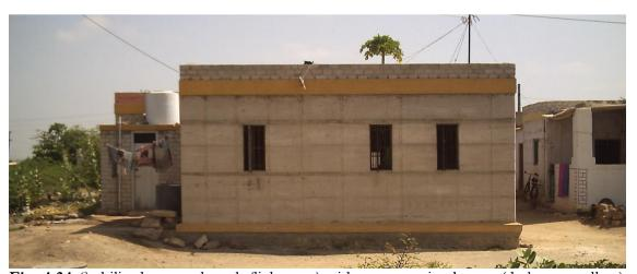
Fig. 4.34: Stabilised rammed-earth (light grey) with concrete ring beams (dark grey, yellow).
