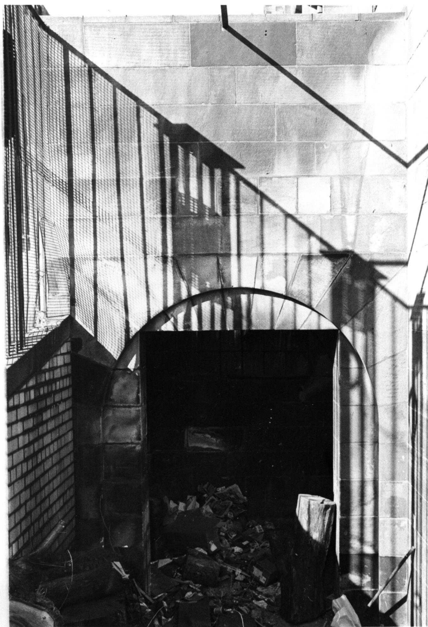
WEST FACADE - SUB BASEMENT DOOR.
