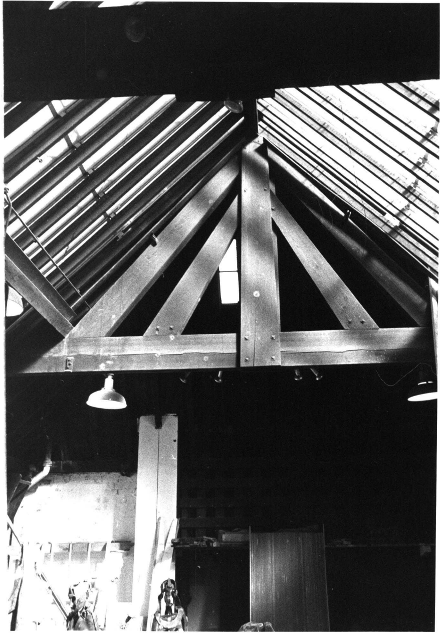
BASEMENT WORKSHOP (WEST WING)
