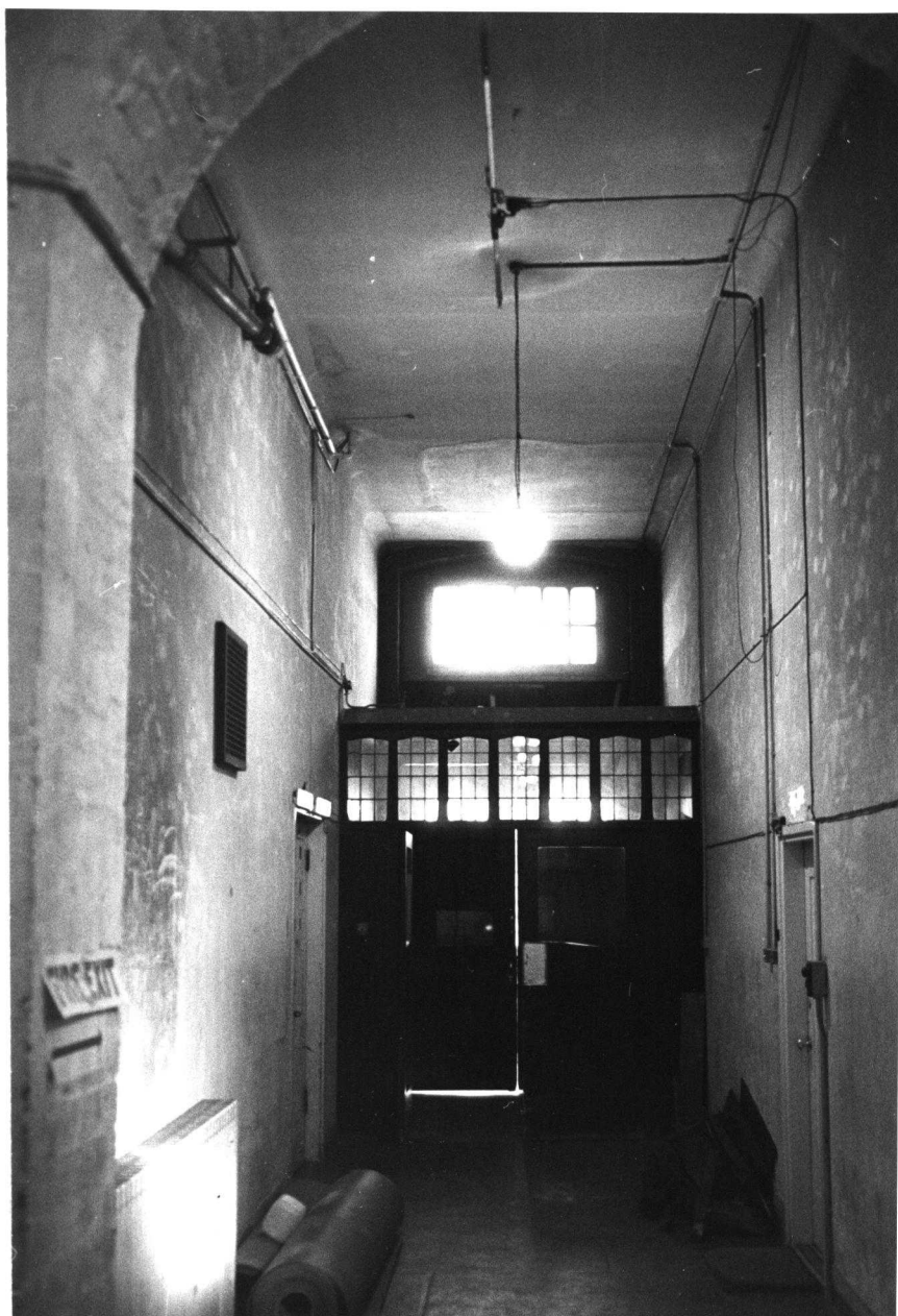
BASEMENT CORRIDOR (EAST WING).
