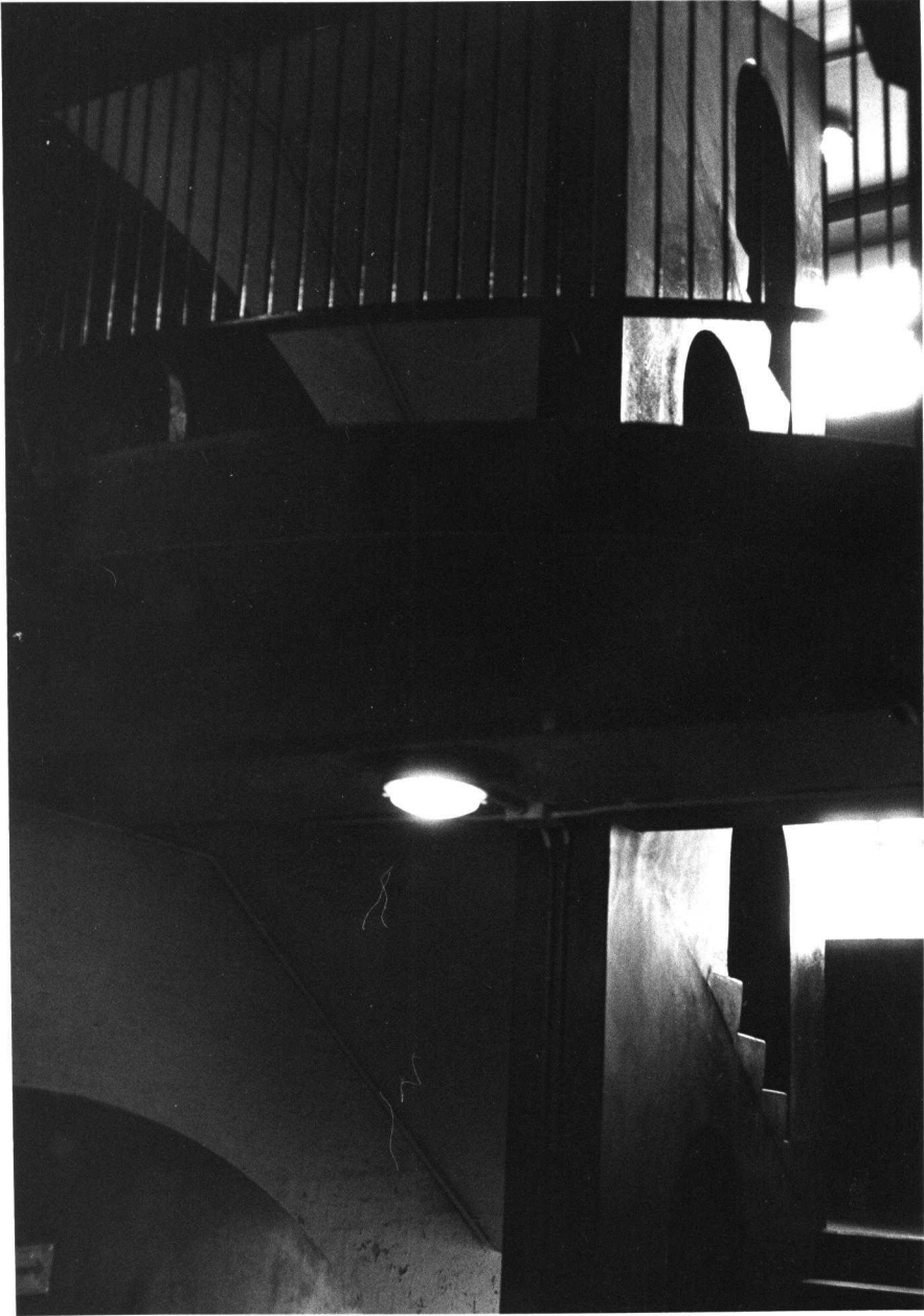
FIREPROOF END STAIRCASE (WEST WING).
