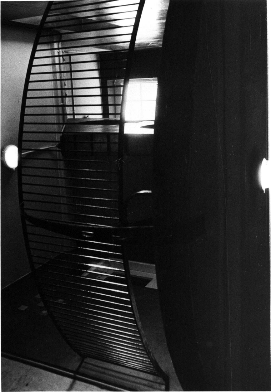
END-STAIR LANDING (EAST-WING)
