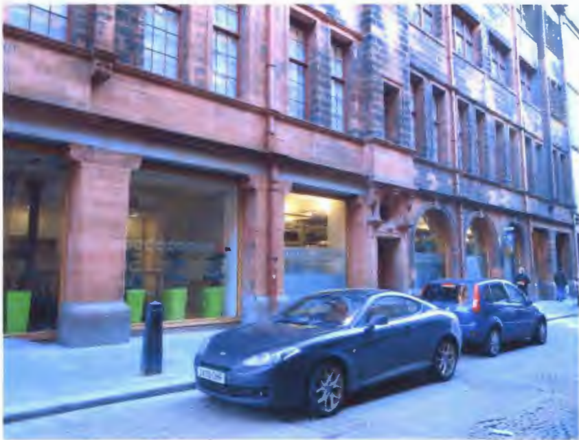
Figure 2 – Westside Mitchell Street in 2011. We can still find the impact of the original building.
