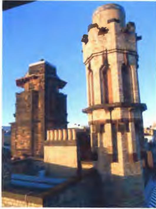
Figure 6 – Water tank bell tower and the chimney
