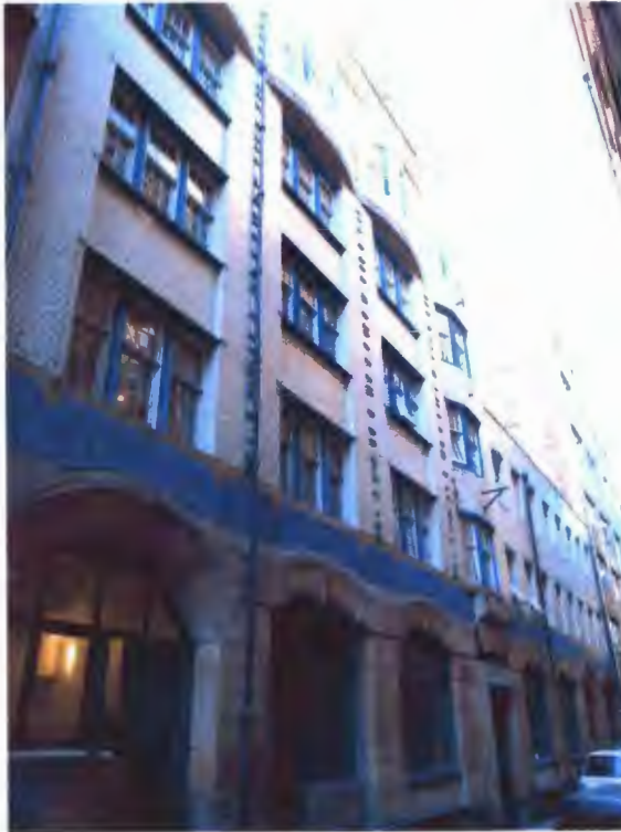
Figure 20 - The south facade of the Daily Record Building.
