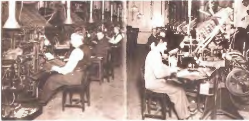
Figure 21 - An old photo in the Herald Building. We can find the white glazing brick on the back of the machines. The white glazing brick was easy to clean up as well as to help lit the room.
