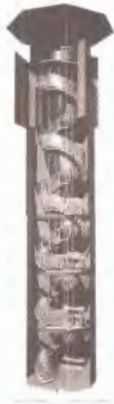
Figure 17 - The Lighthouse's water tank staircase. It starts from third floor.
