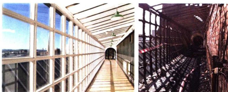
Figure. 12 'Hen run' corridor on the top floor before the fire (left)
