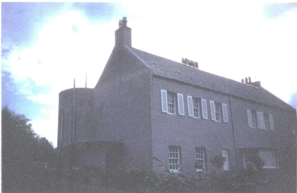
B. Windyhill : View from South-West
