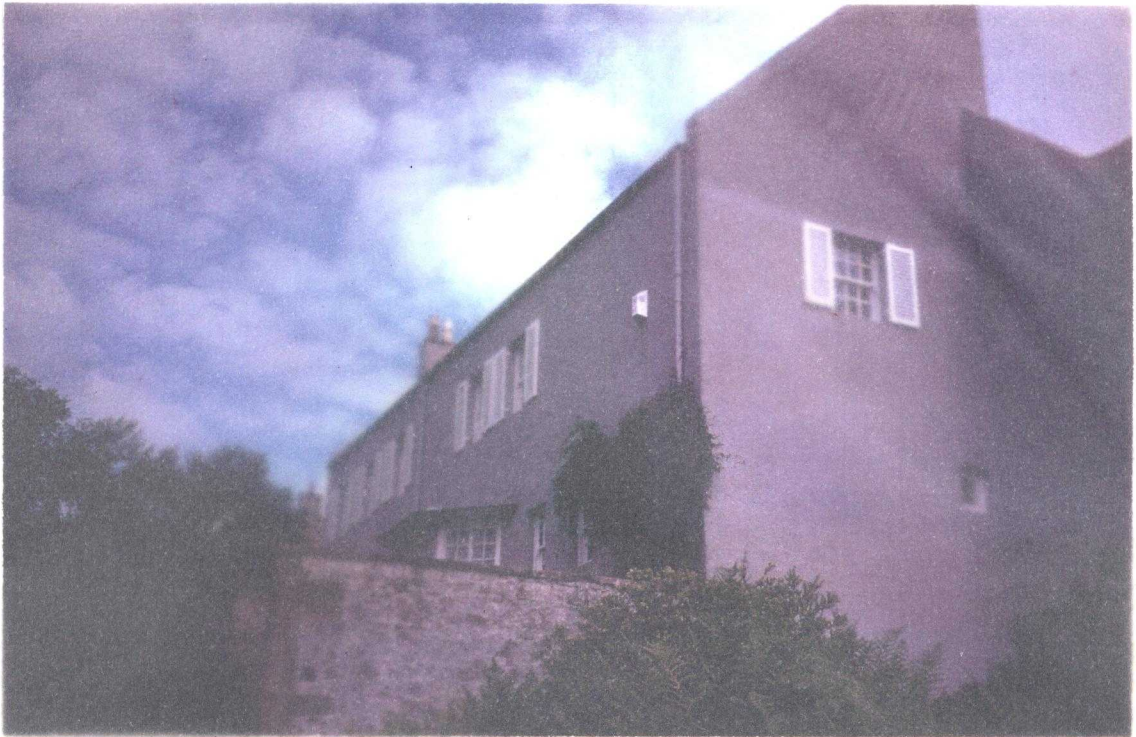
A. Windyhill : View From South-East
