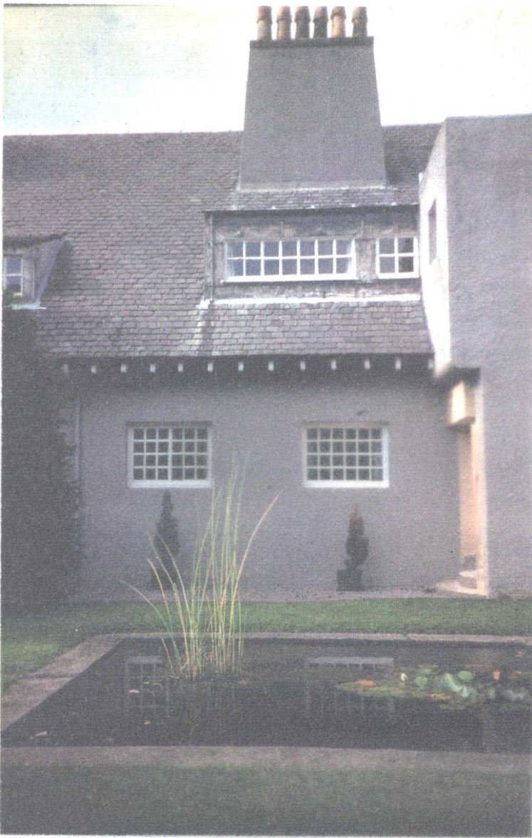
A. Windyhill : Detail of Overhanging Eaves
