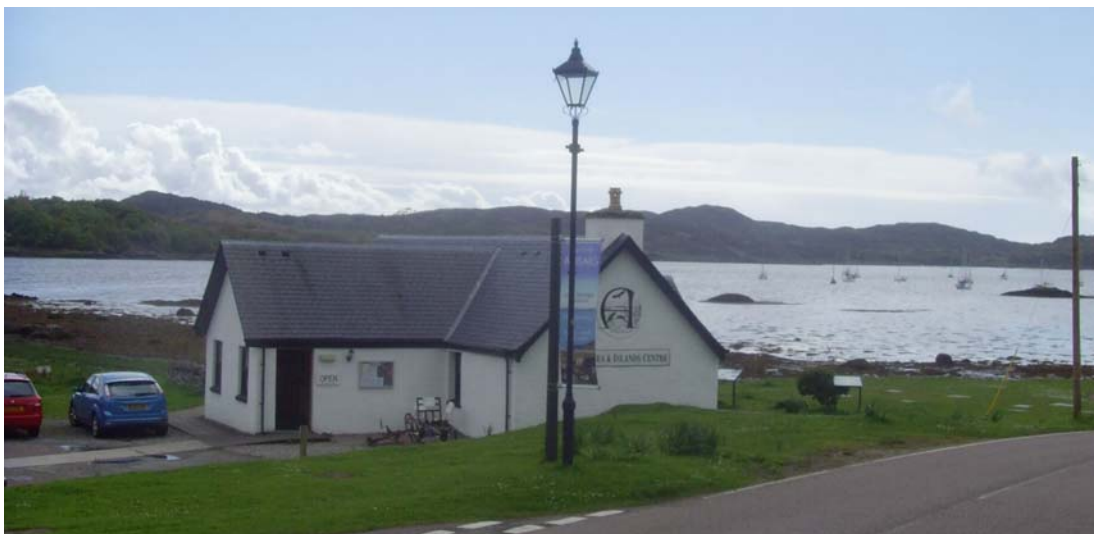
Figure 1. View of LSIC building, north facing entrance and reception and north gable wall of exhibition area.
