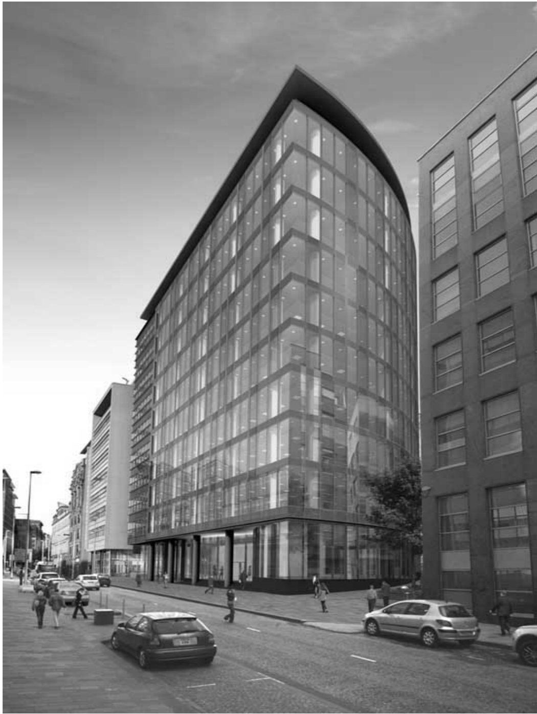
Fig 3.4 Capella 5 Atlantic Quay, York Street
