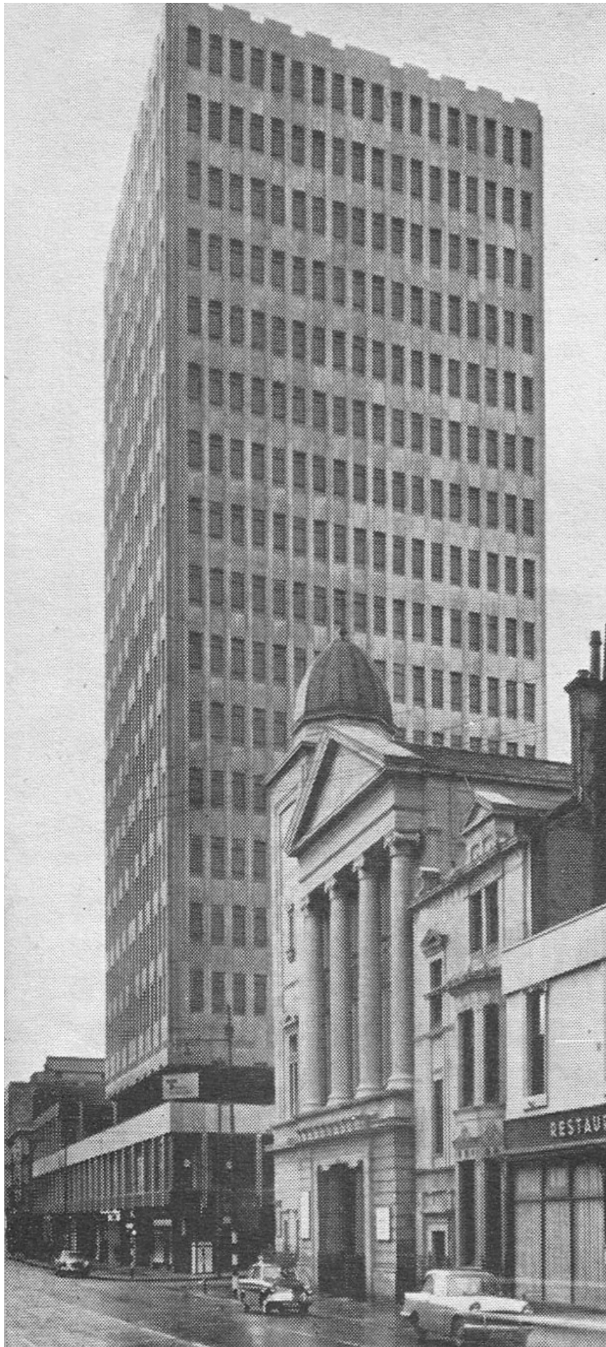
Figure 3.3 St Andrew's House 1962 141 West Nile Street
