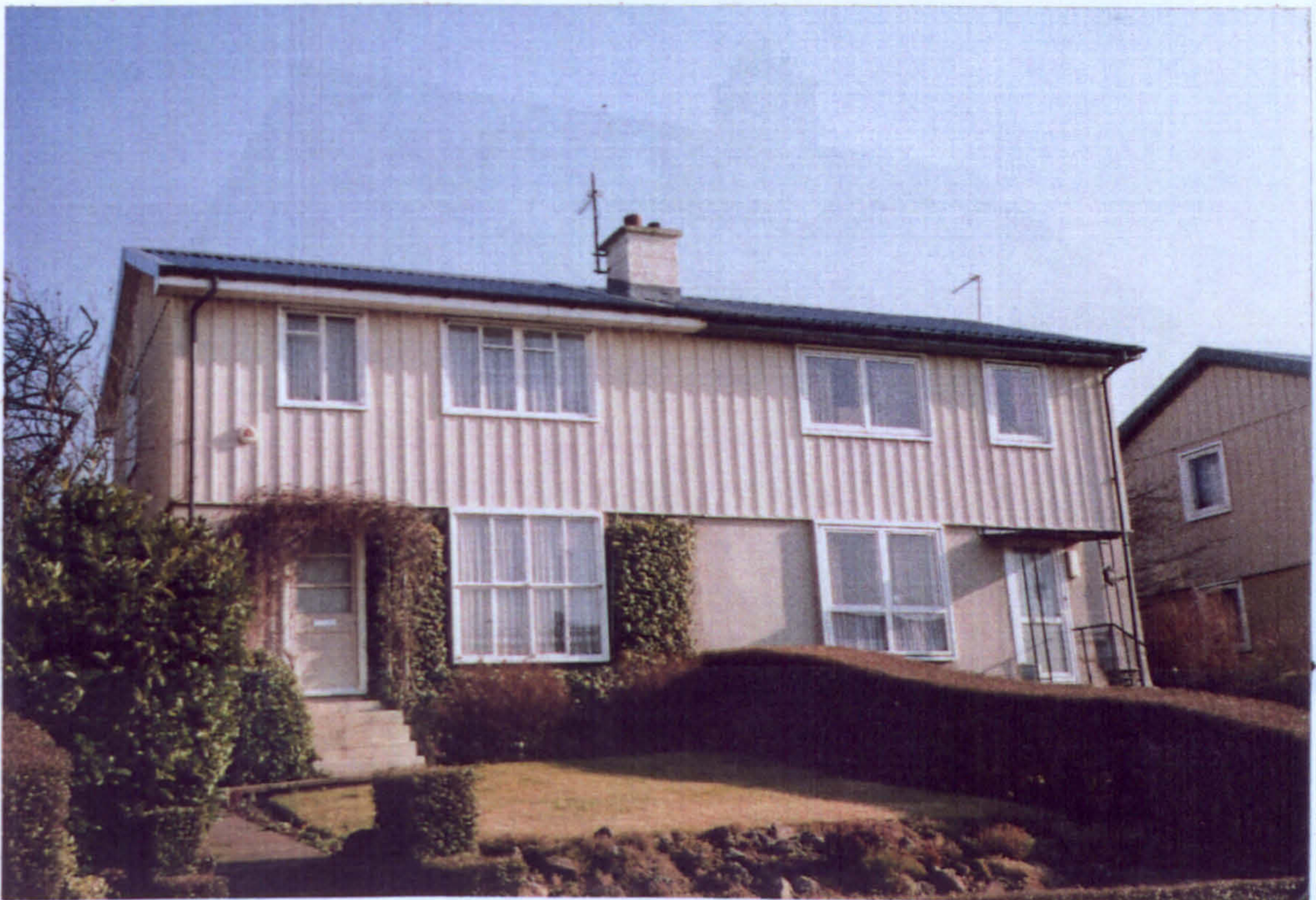
House on left with original door and windows. Note how the window mullions line with sheet corrugations. South of London Road, Kilmarnock
