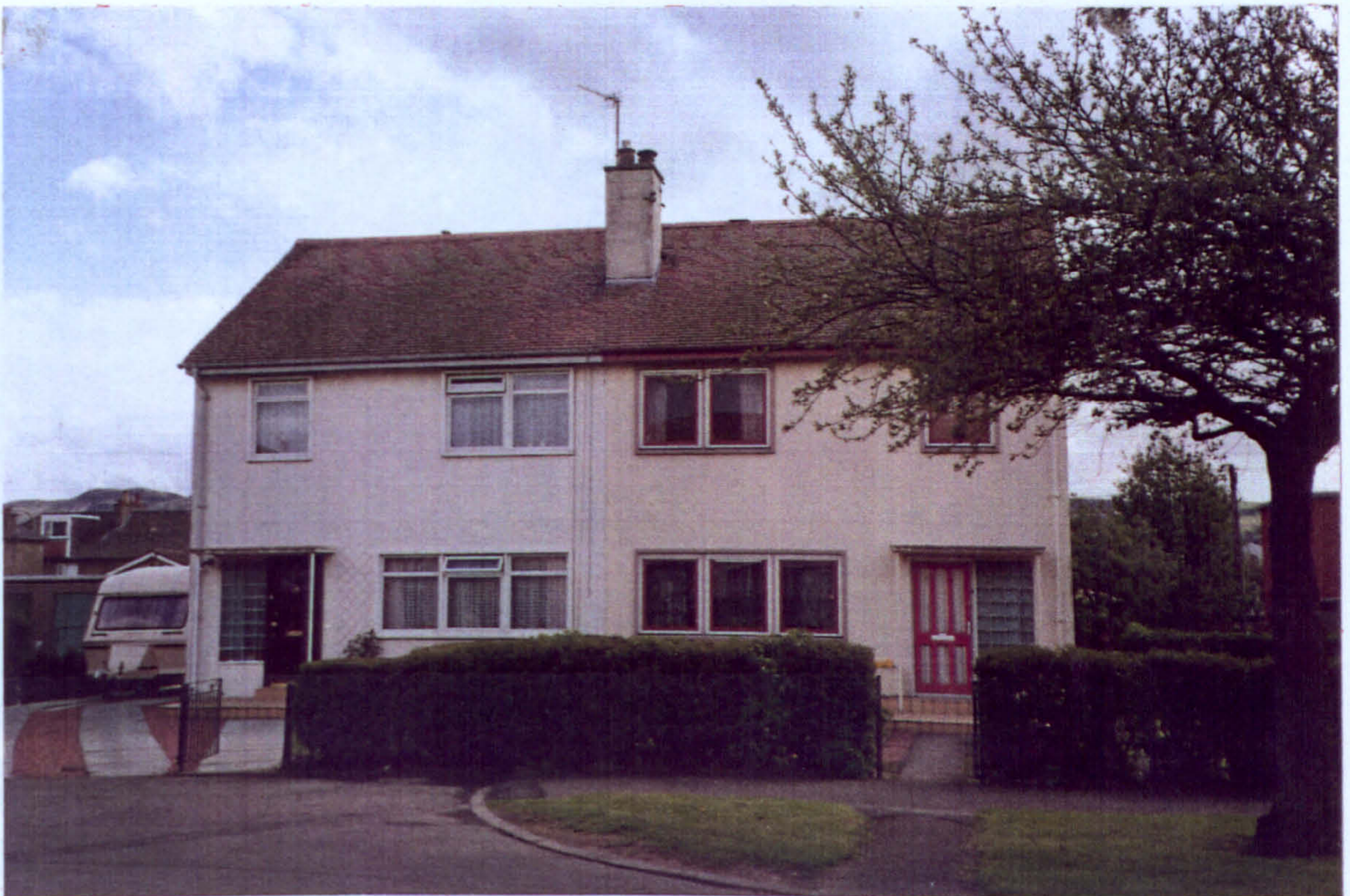
RH plans and above Foamslag Poured Insitu 10/12 Sighthill Neuk. LH plans Foamslag Blockwork houses at 25/27 Sighthill Neuk, Edinburgh
