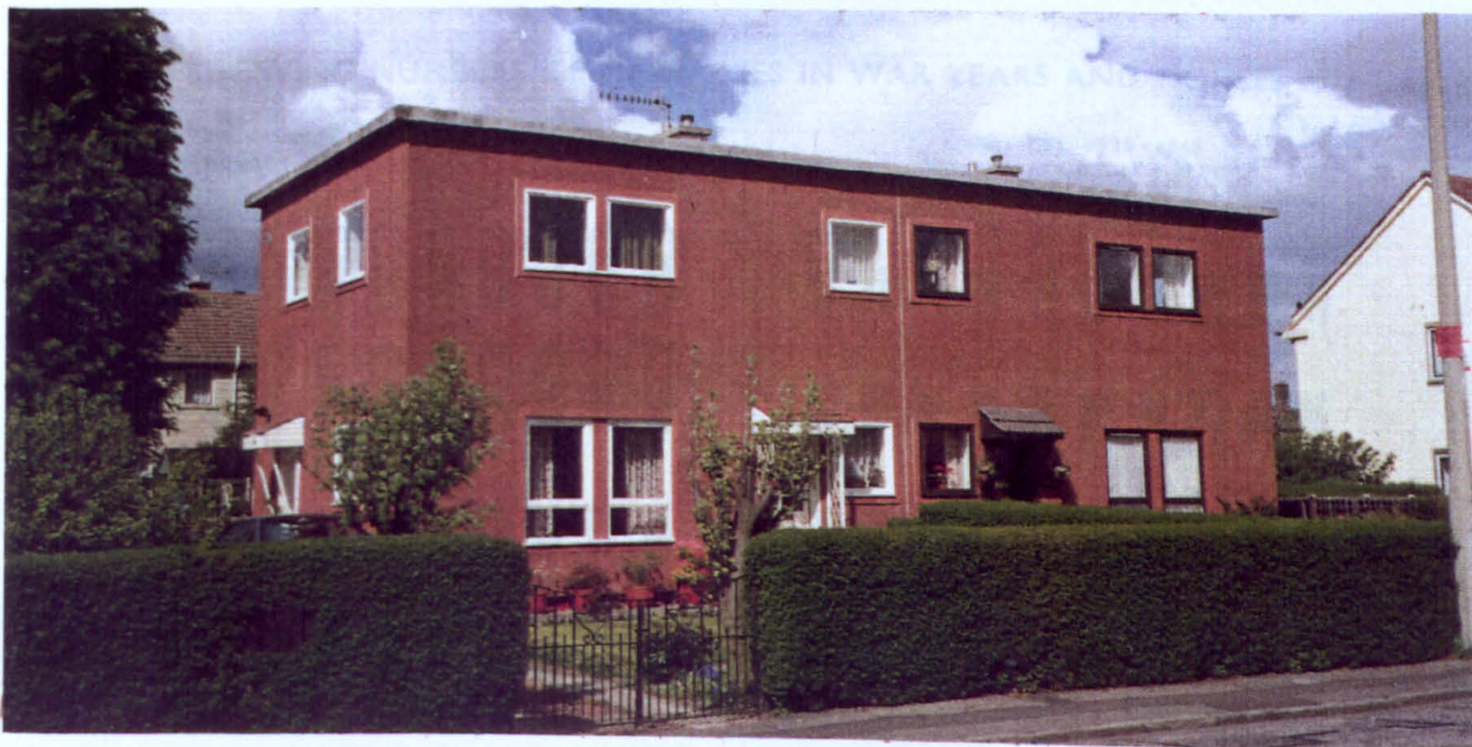
56 and 58 Sighthill Road, Edinburgh. The system was approved by the Burt Committee but these were the only 2 built in Scotland. One of the few systems to have a flat roof.
