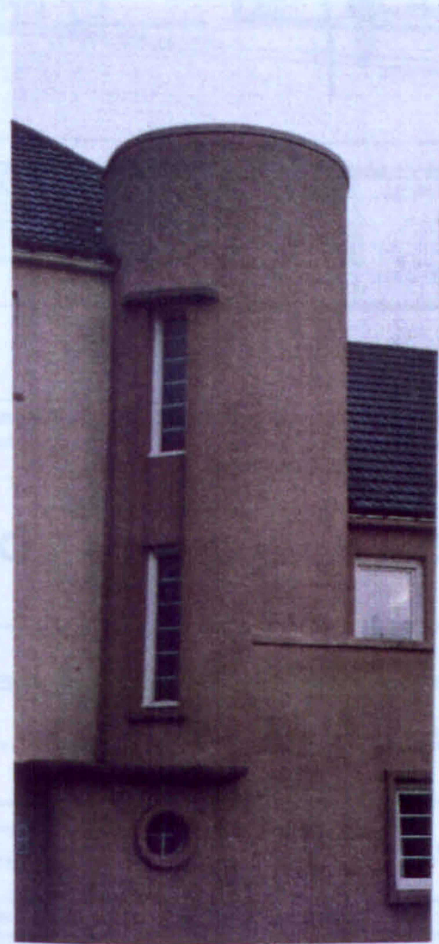
Larchgrove Road was designed in the late 30's but built in 1946. The block encloses an entire street block. Shops and community rooms built in at the centre of the long sides. Horizontal metal windows have been replaced with double glazing with horizontal astragal insets in the glazing cavity.
