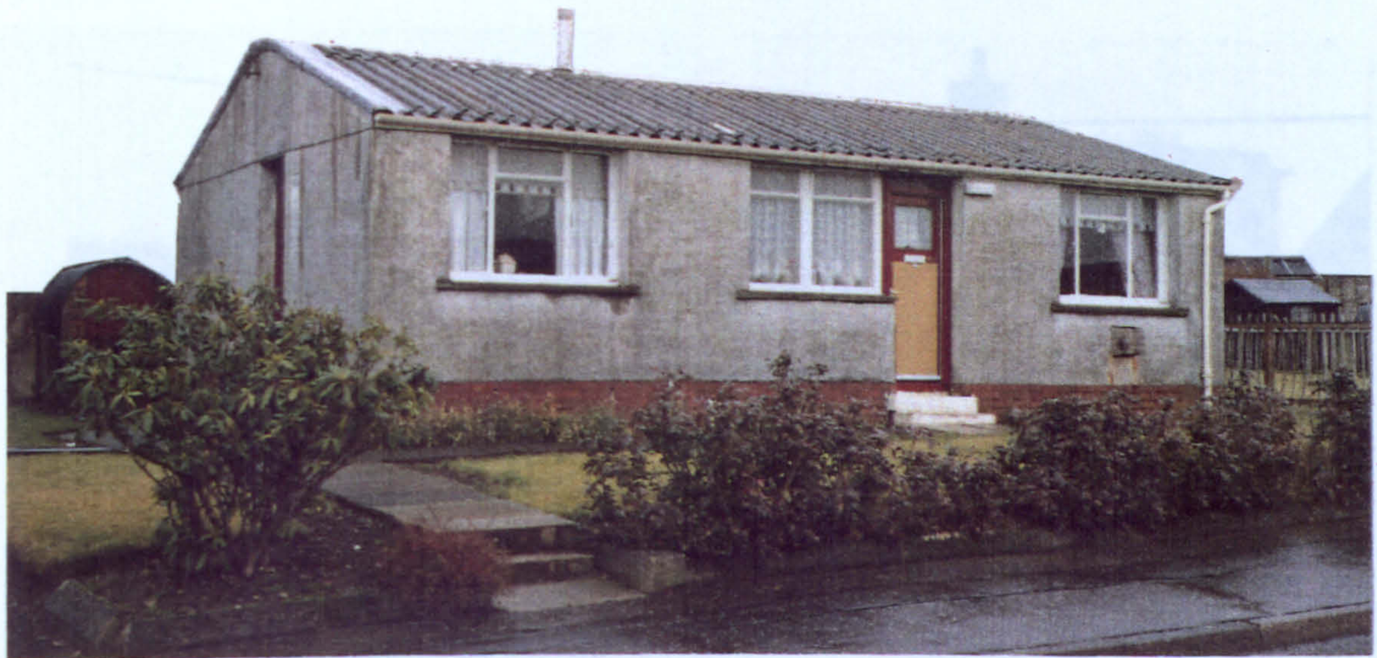
50 year old prefab Broomhill Quad Kilmarnock, may be Seco Mark 1 or Arcon Mark 5 Brick Skin and render added to extend life.
