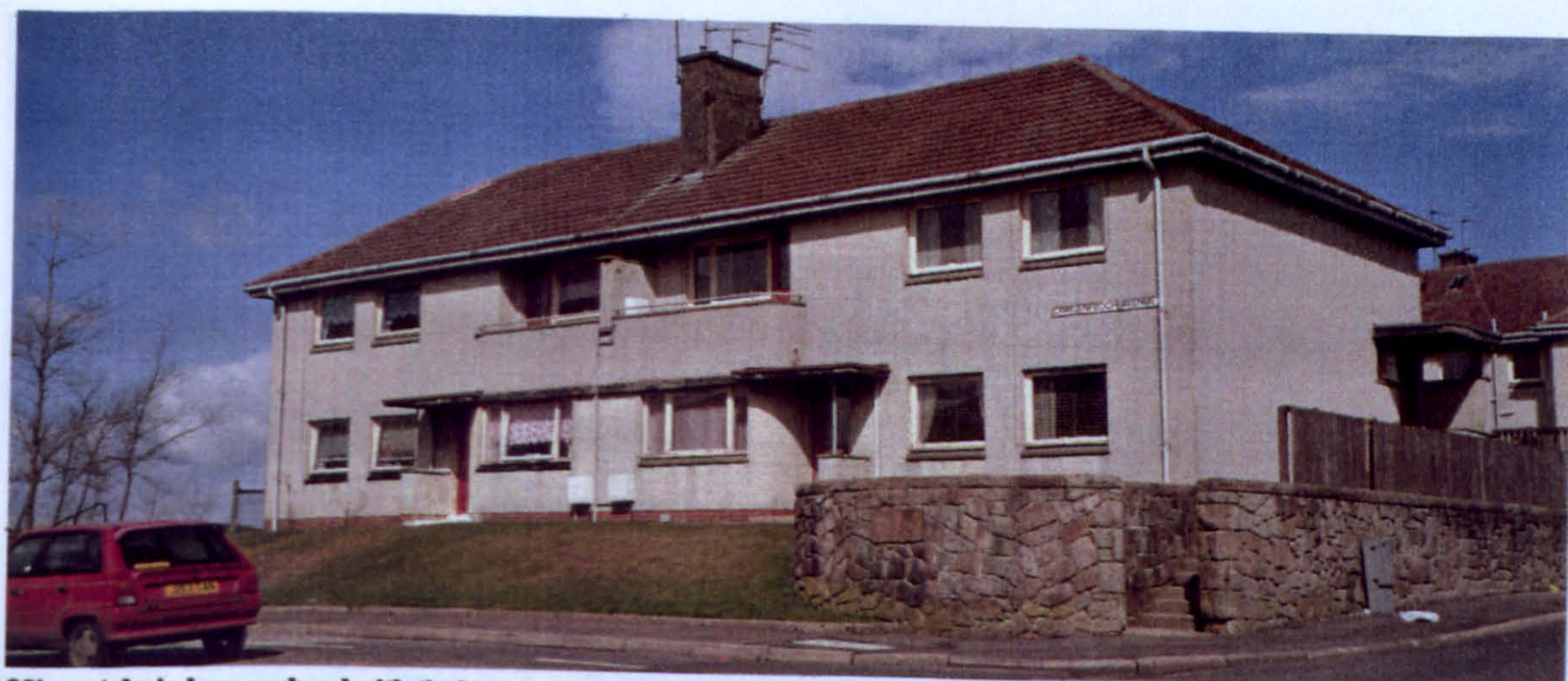
30's metal windows replaced with timber pivots
