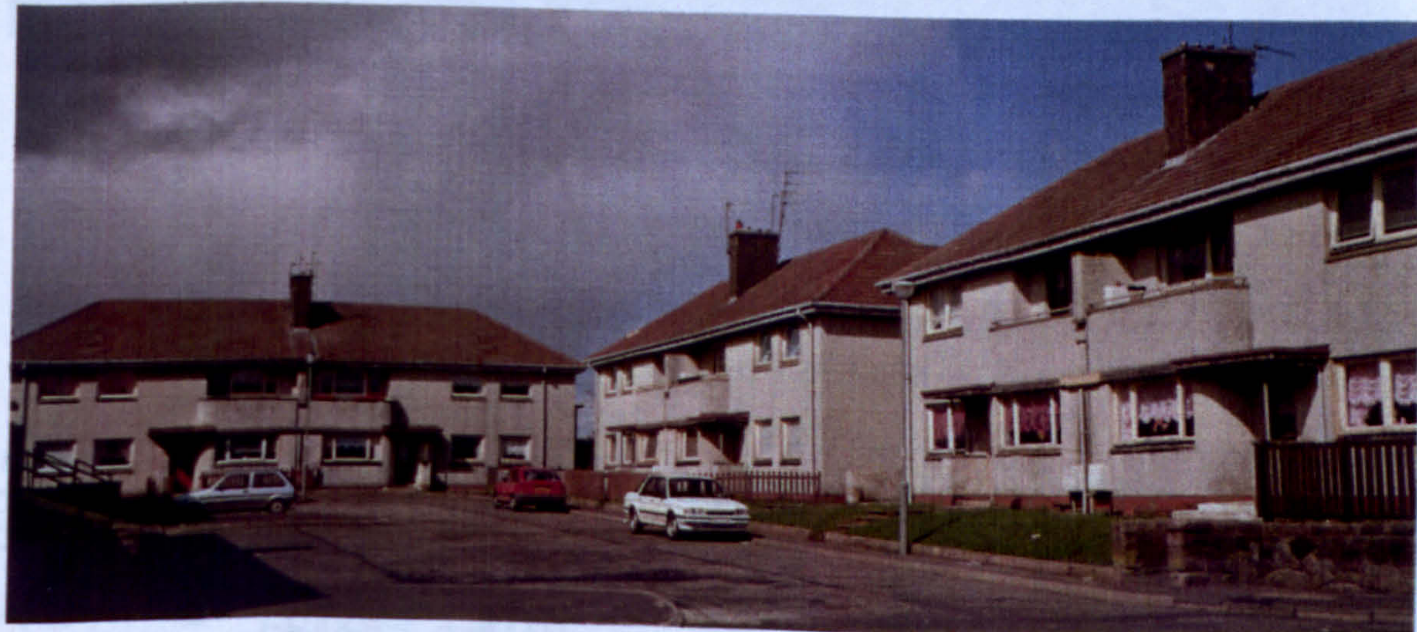
open coal fires replaced with gas central heating slate roofs replaced with tile
