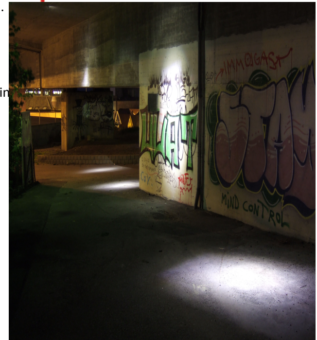
Image of the underpass space with the lighting system in operation.
