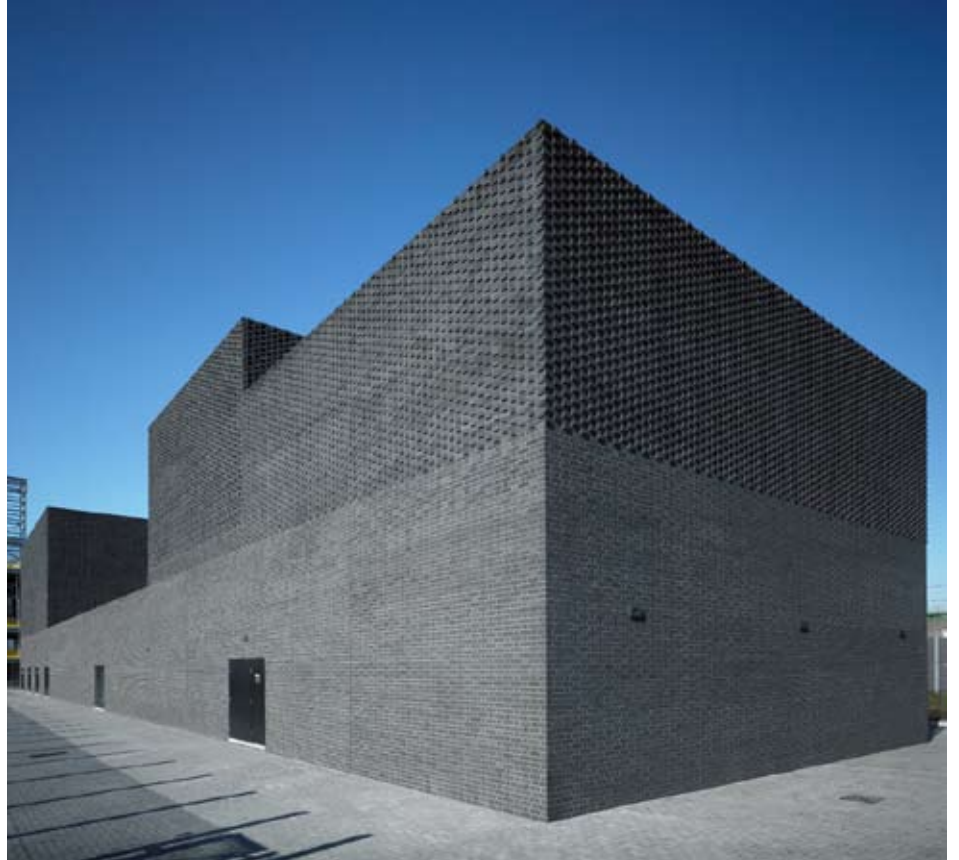
Completed Substation - photographic record of completed building
