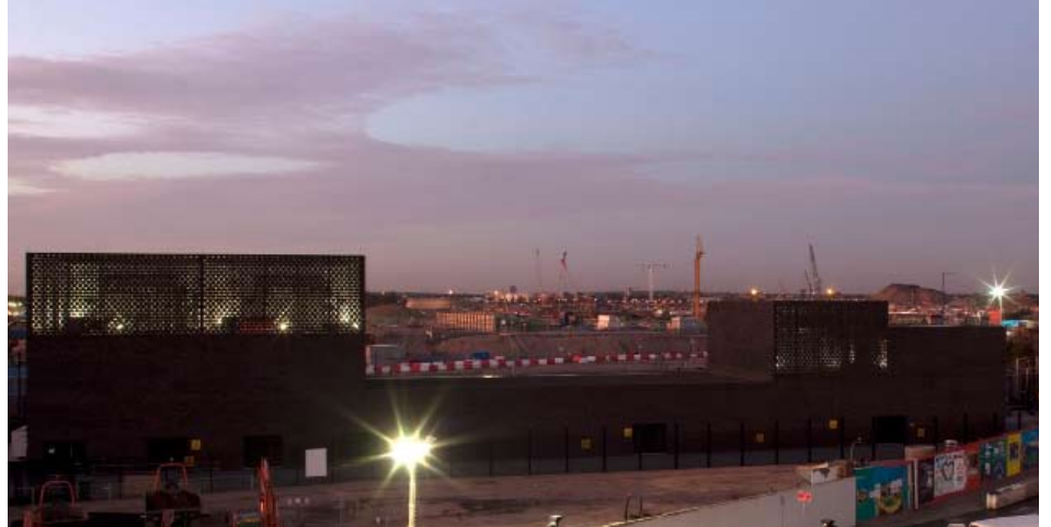
Completed Substation - photographic record of completed building
