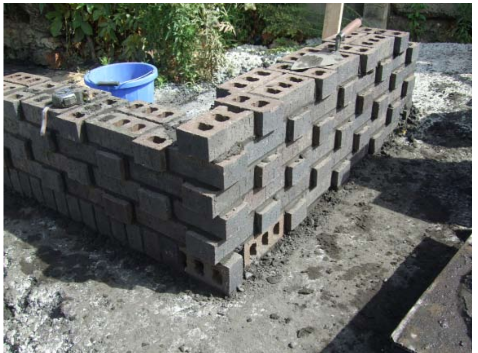
Brickwork Sample Panels - evidence of site enquiry into appropriate detailing methods and of what would be achievable within the parameters of the material and the abilities of the workforce
