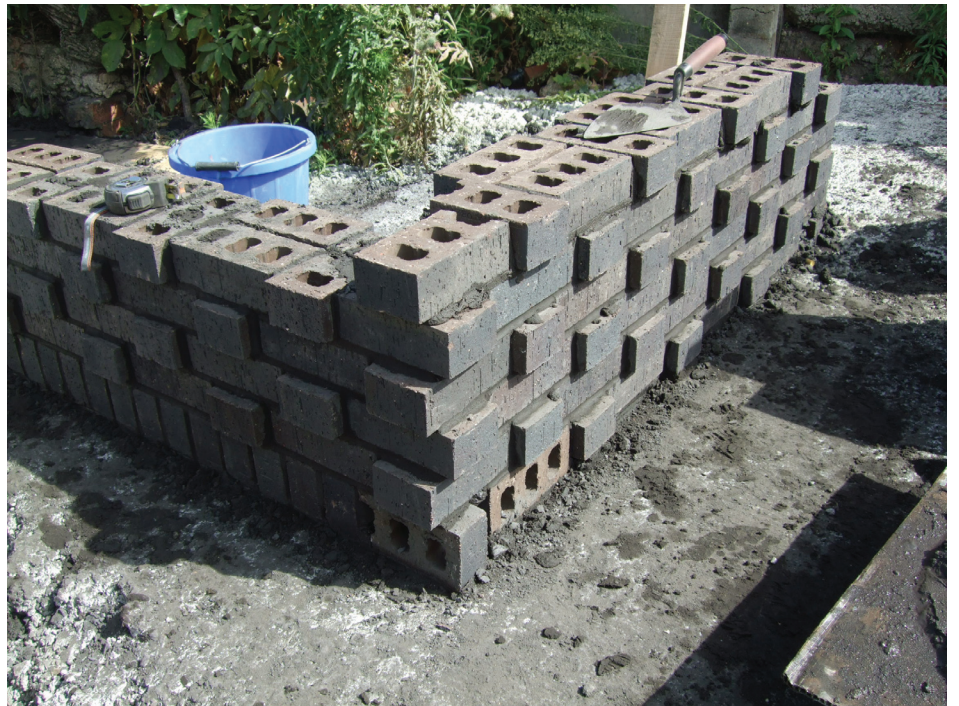
Brickwork Sample Panels
