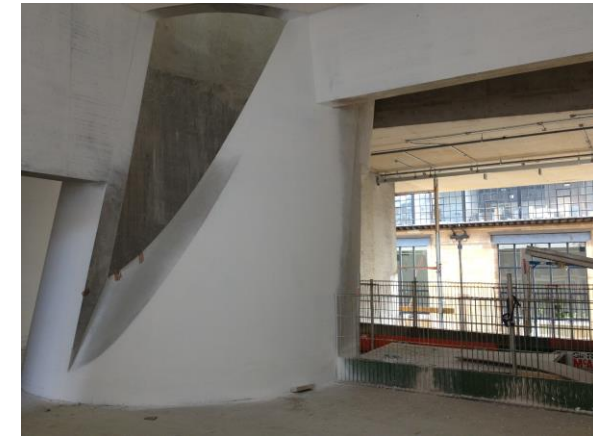
Construction view of driven void
