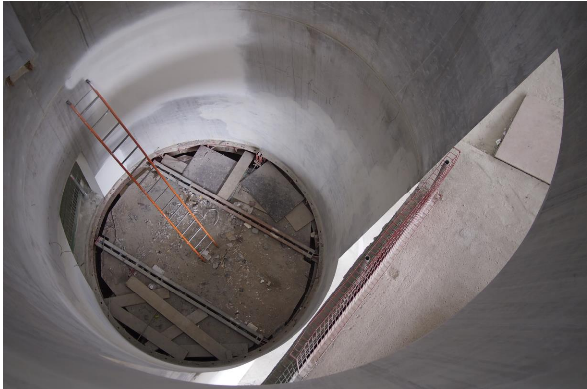
Construction view looking down a driven void
