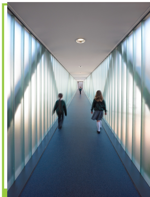
View of translucent glass clad link between
