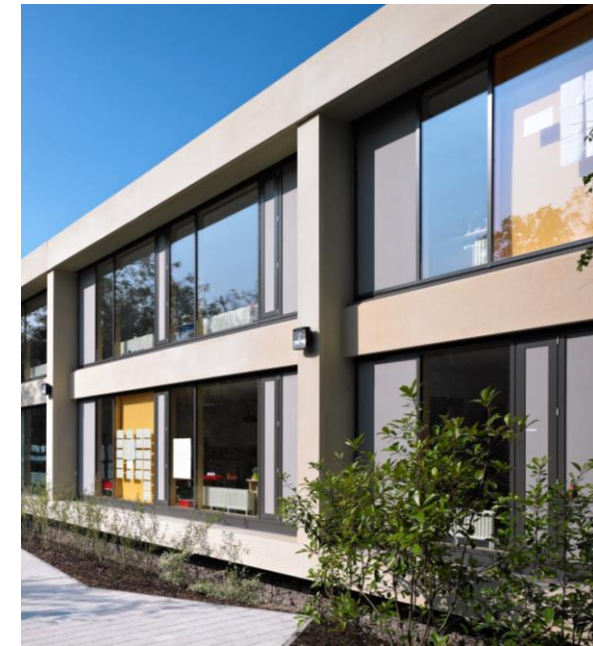
View of teaching wing , acid etched precast concrete panels & full window screens
