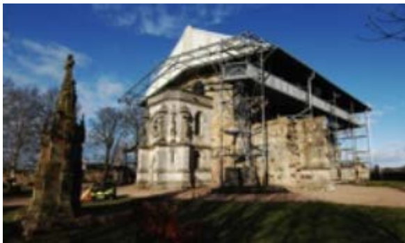
Image One: Chapel exterior with temporary protective metal shed roof
