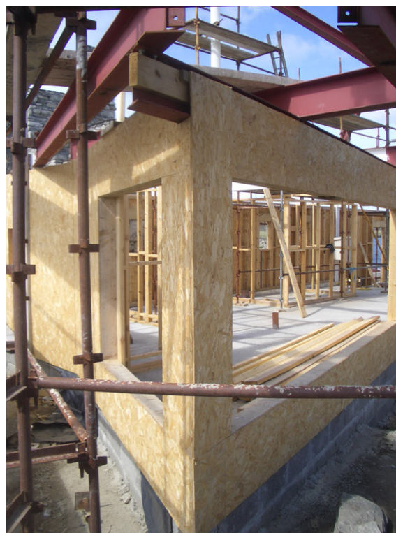
Steel & timber frame contrasting with existing ruined load-bearing construction.
